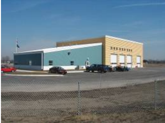
Blue Water Bridge, Salt Storage and Maintenance Facility in Port Huron. Photo courtesy of Hubbell, Roth & Clark, Inc.
