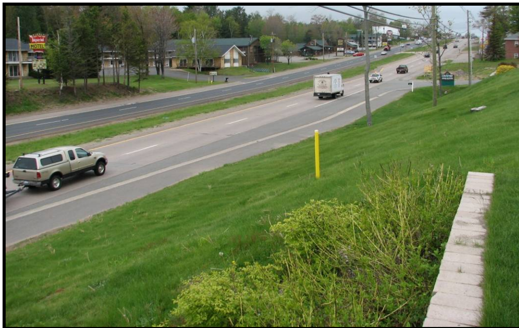
Figure 2-14. Right-turn lane installed upon development of new hotel.
