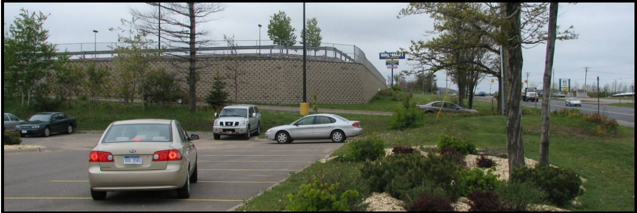
Figure 2-16. Topography prevents cross access between adjacent properties as recommended in access management plan.
