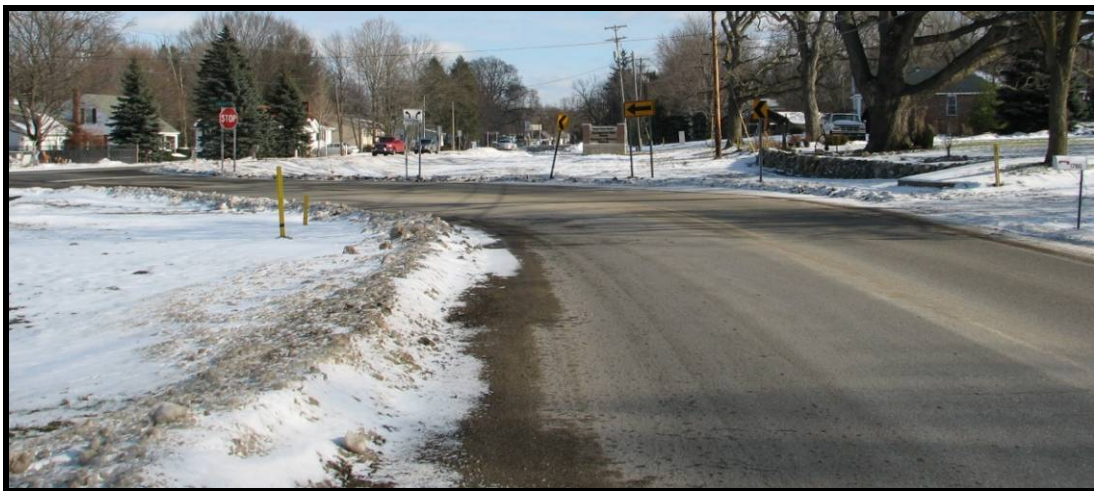
Figure 2-12. Reconfigured intersection to improve geometrics.
