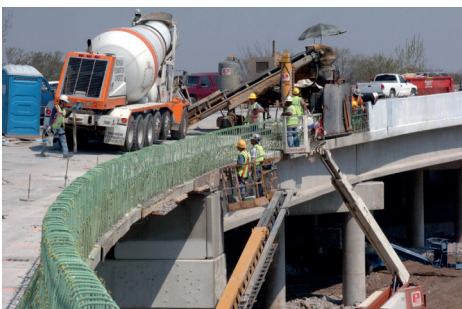
Construction workers installing concrete bridge barriers
