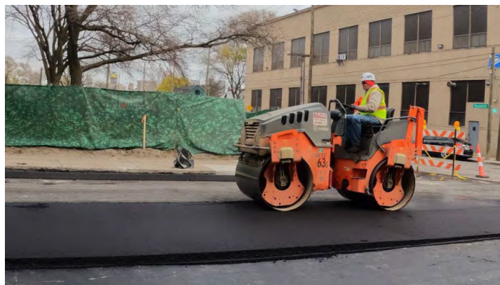
Roller compacting new pavement on 14th Street
