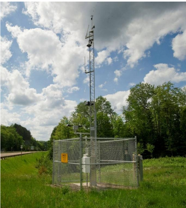
Figure 11 - Environmental Sensor Station
