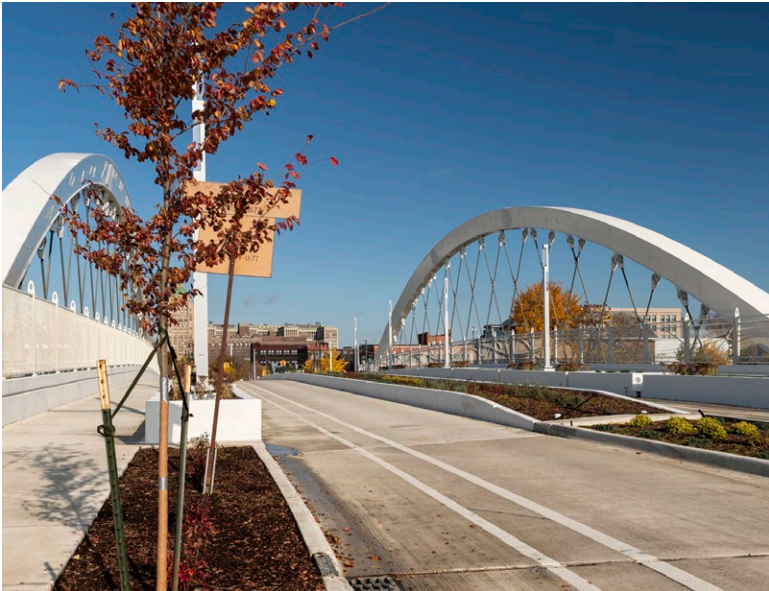
Second Avenue bridge over I-94 in Detroit.
