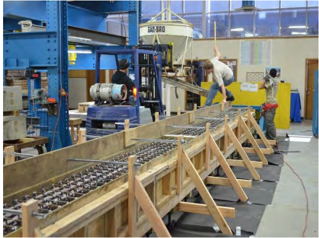
Figure 4.3-8 Placing concrete in the formwork
