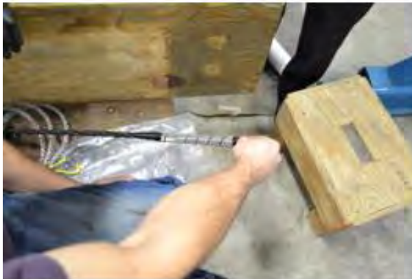
(c) Securing steel mesh in place with tape
