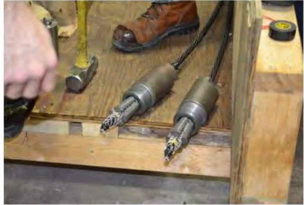
(b) Completed anchorage device
