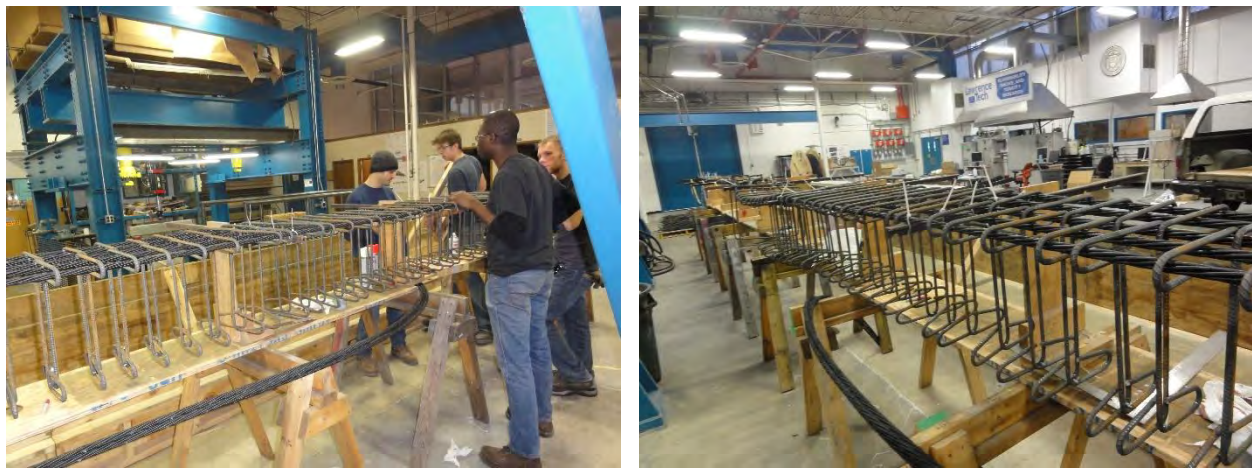
Figure 4.3-2 Assembling the reinforcement cages for decked bulb T beams
