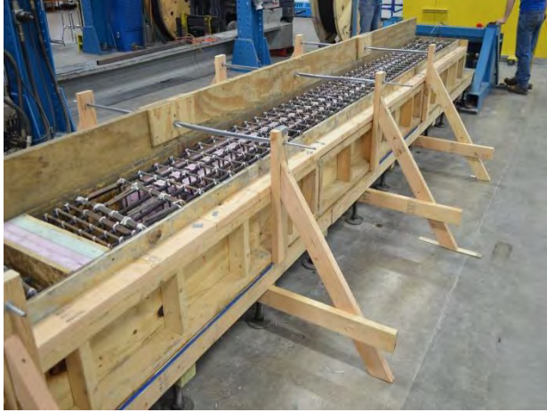
Figure 4.3-4 Completing the formwork and adding separators between beams
