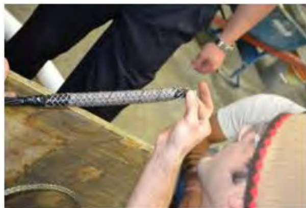
(e) Securing steel wire netting with tape
