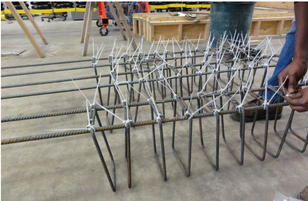
Figure 7.3-3 Assembling the reinforcement cages of the test beams
