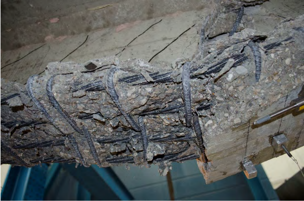
Figure 5.2-26 Close-up picture for CFCC strands in Beam F1 after failure
