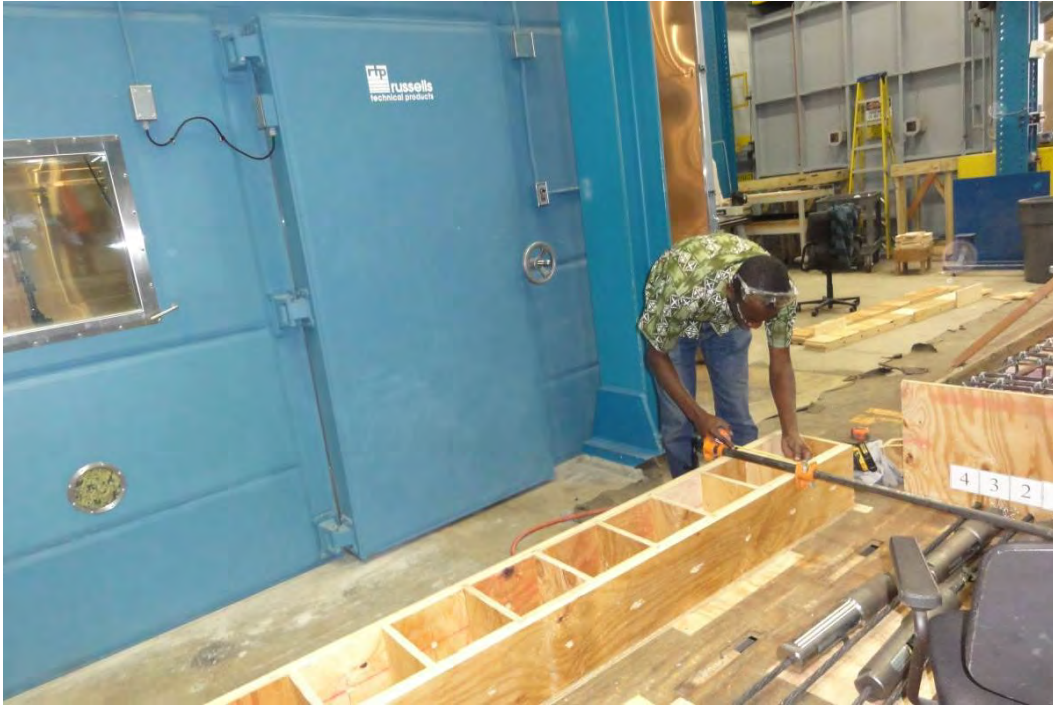
Figure 7.2-2 Formwork for pull-out test specimens
