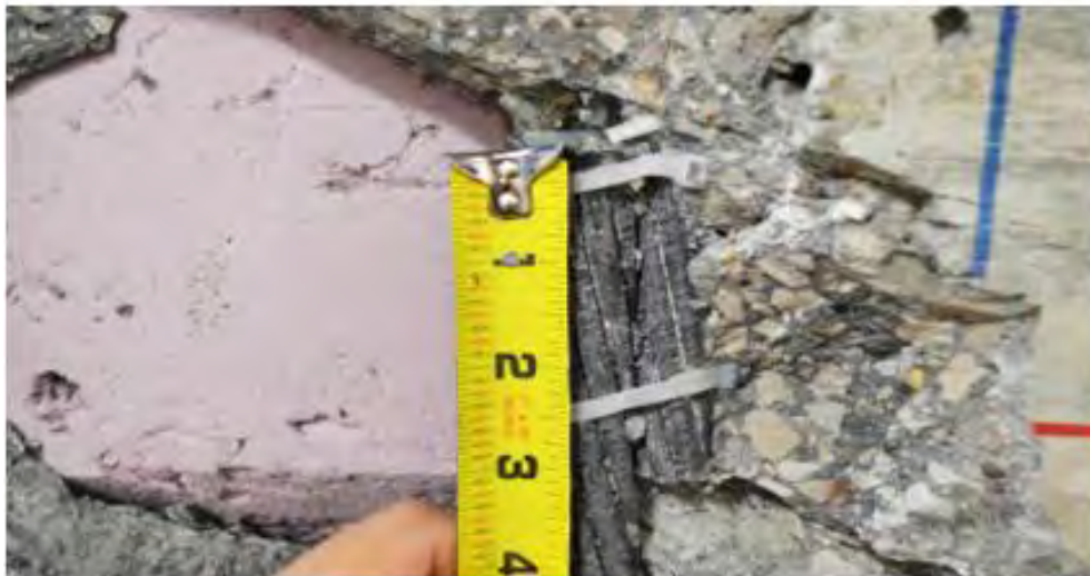
c) Slippage of the 4 in. (102 mm) spliced stirrups
