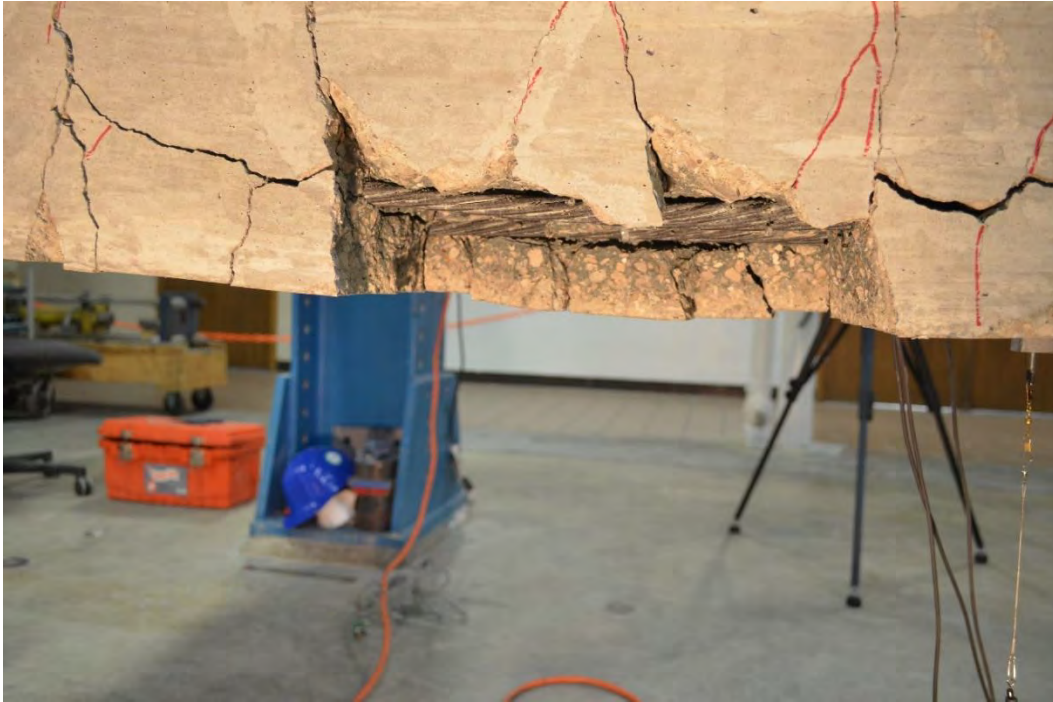
Figure 7.3-23 Close-up view of B4-0.5 showing CFCC slippage at the end of the splice
