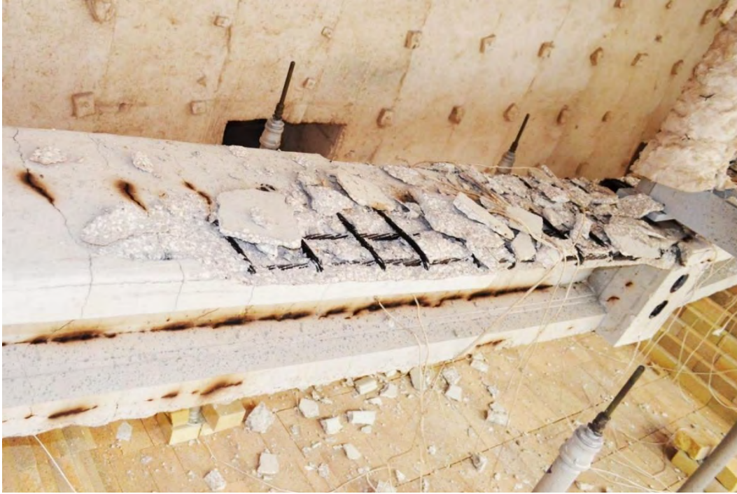
Figure 6.3-44 Concrete spalling of Beam C100-20-4 after fire
