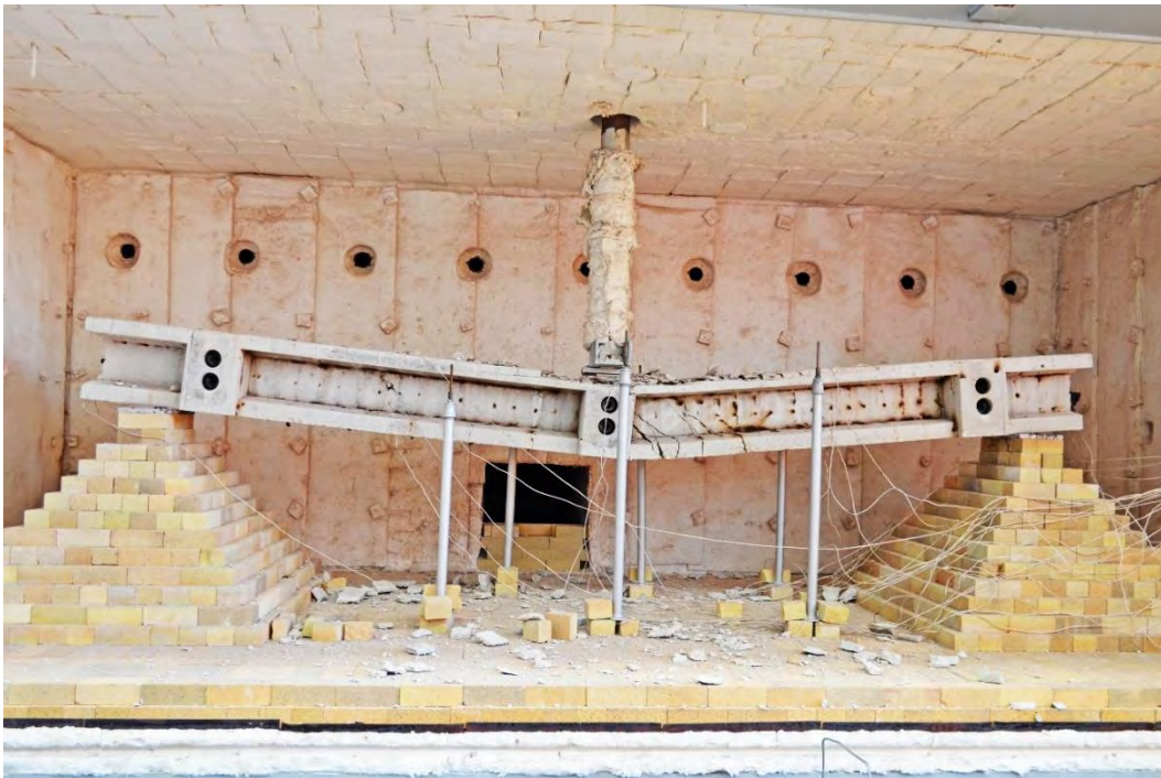
Figure 6.3-55 Beam C132-25-1 after fire
