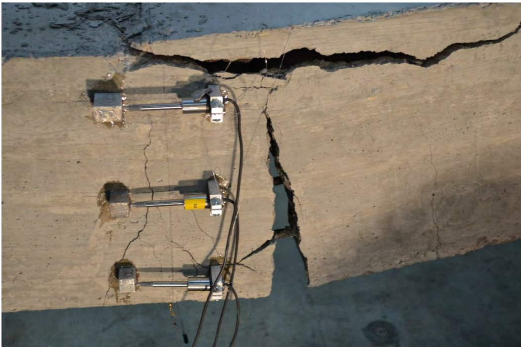
Figure 7.3-14 Close-up view of B1-0.5 showing a large crack at the end of splice
