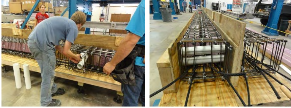
Figure 8.2-5 Installing PVC conduits in the end block of the beams
