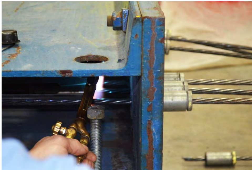
Figure 8.2-15 Release of steel strands at transfer
