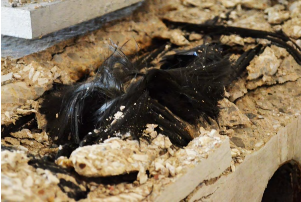
Figure 6.3-38 Carbon fiber filaments after burning of epoxy adhesive in Beam C100-20-3
