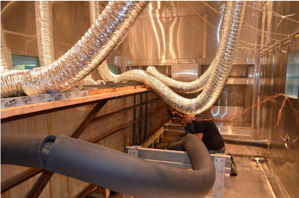
Figure 5.2-5 Duct work for air freezing and water thawing according to ASTM C666
