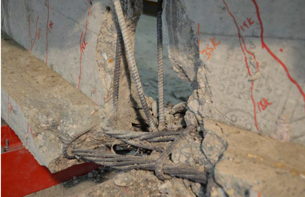
Figure 8.2-58 Un-ruptured prestressing strands of Beam O-2 at failure
