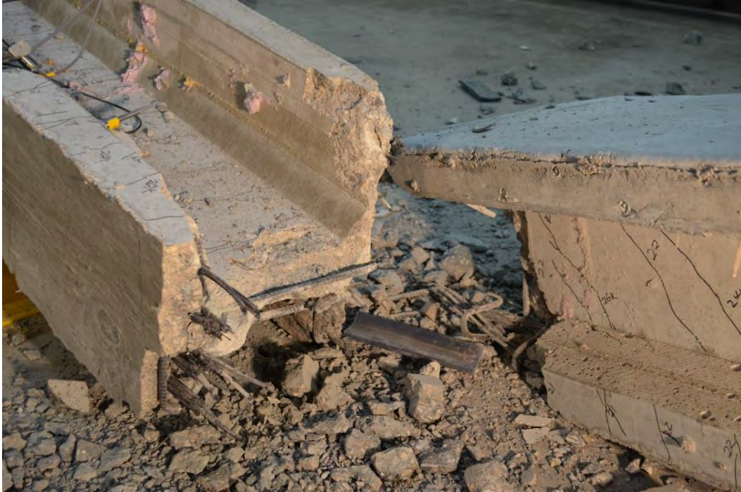
Figure 8.2-52 Ruptured prestressing strands at failure of Beam O-1
