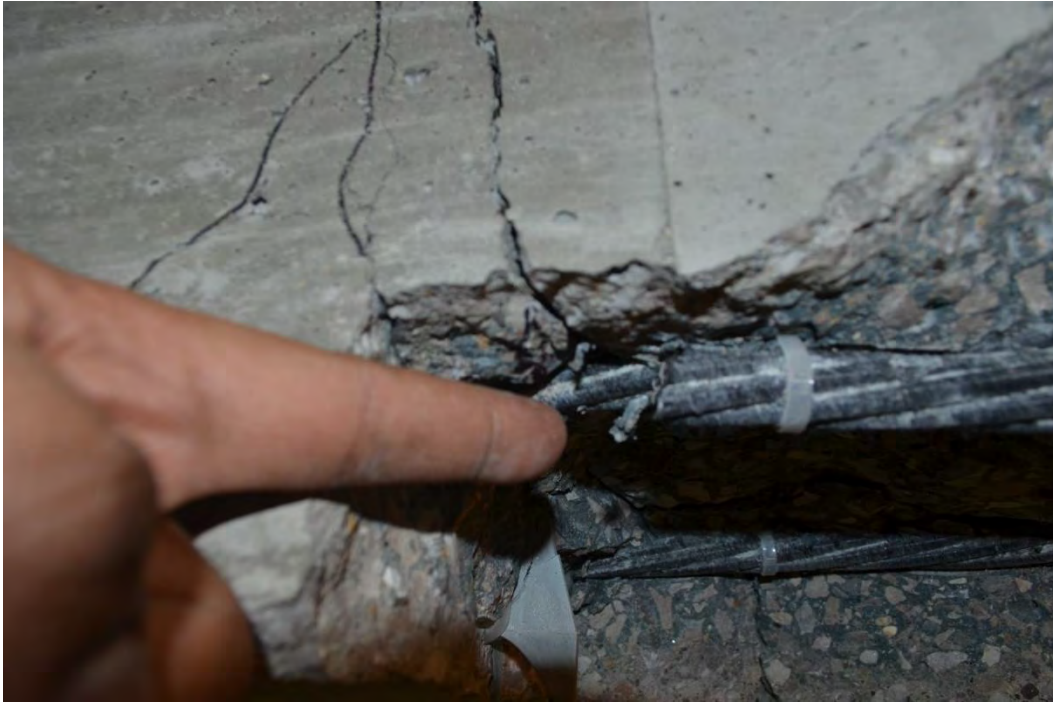
Figure 7.3-37 Close-up view of B4-0.6 showing CFCC slippage at splice end
