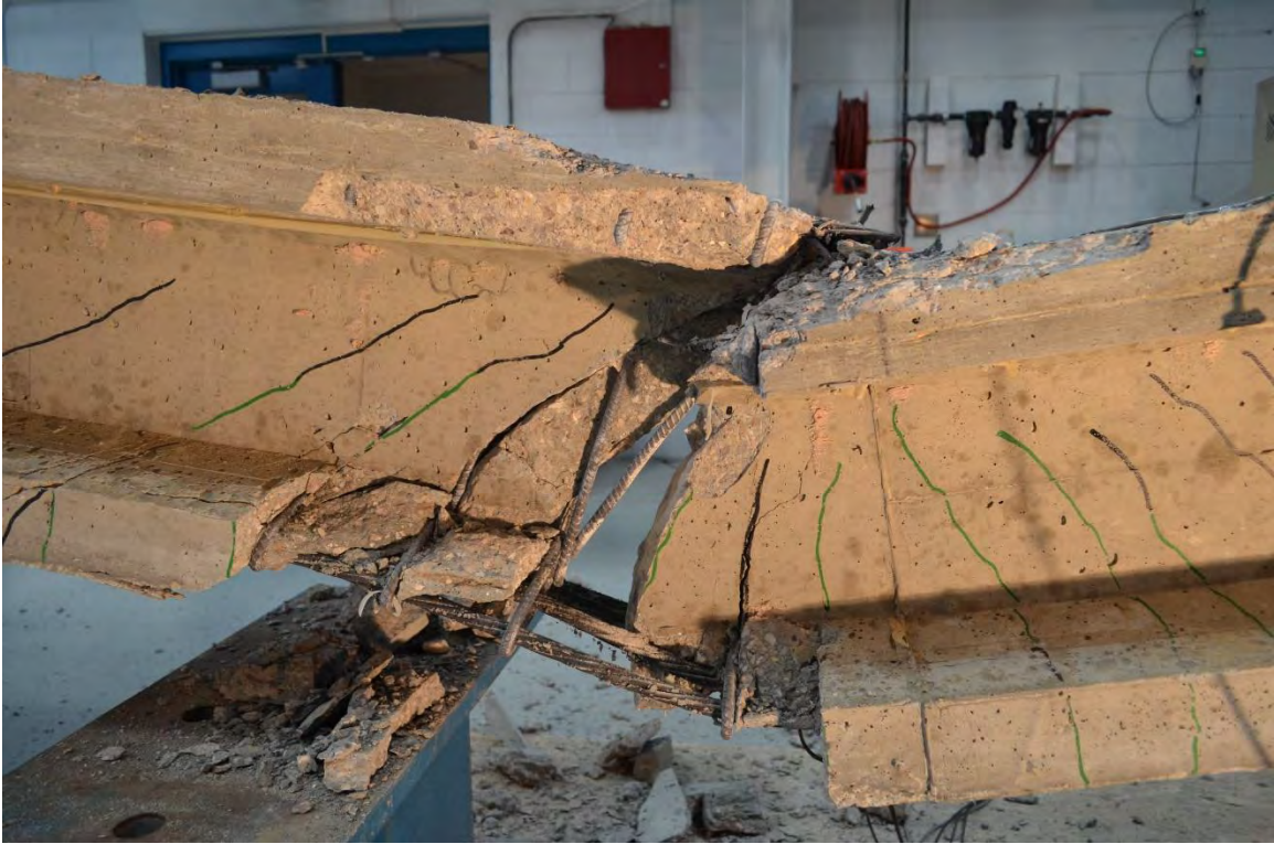
Figure 5.2-30 Close-up picture for CFCC strands in Beam F2 after failure
