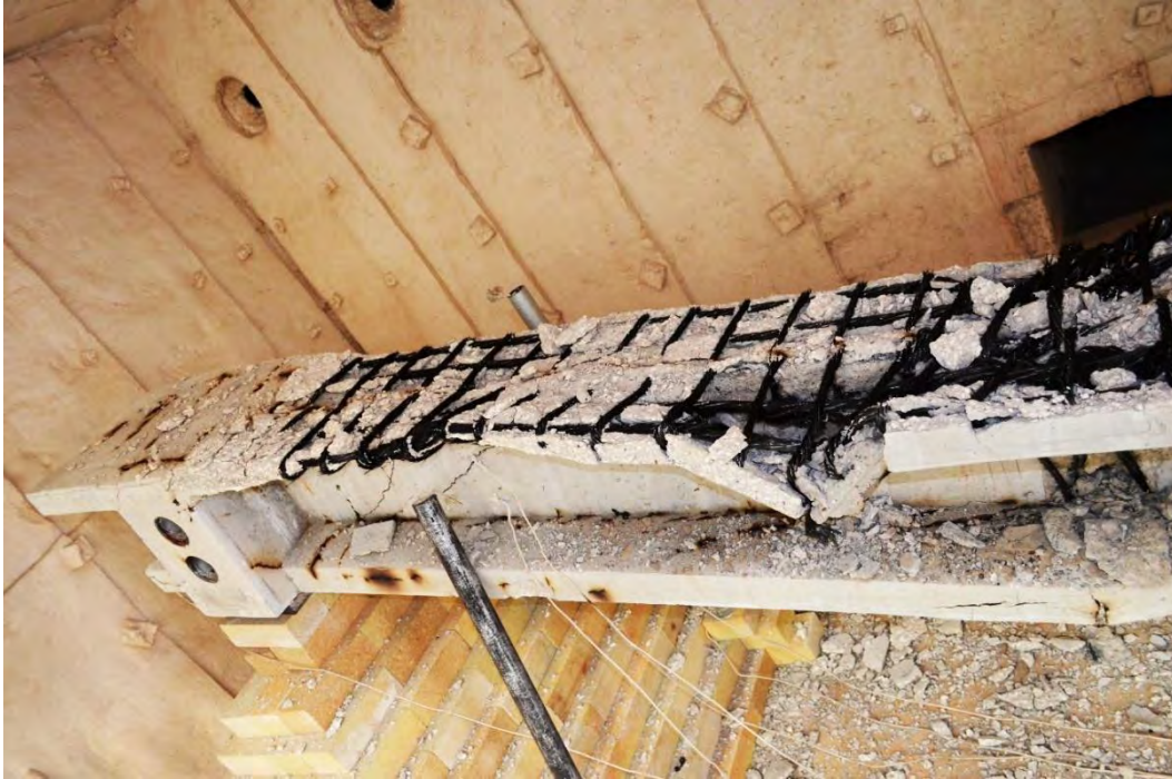
Figure 6.3-26 Concrete spalling on CFCC stirrups side of Beam C100-20-1 after fire
