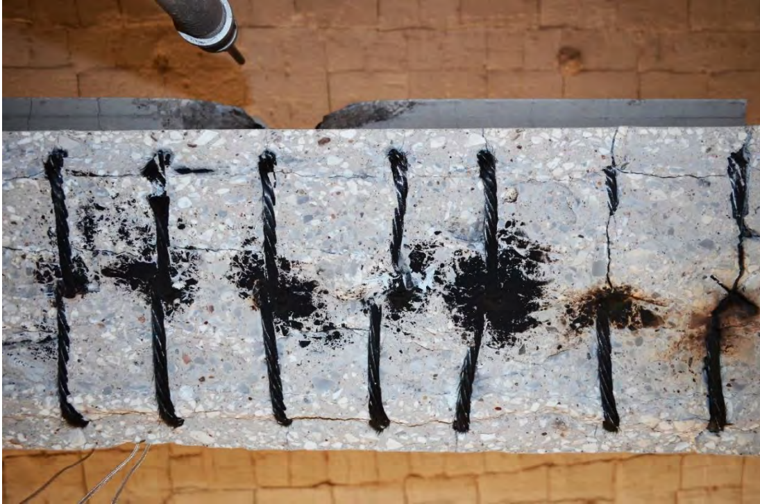
Figure 6.3-32 Concrete spalling of bottom flange of Beam C100-20-2 after fire, bottom side view
