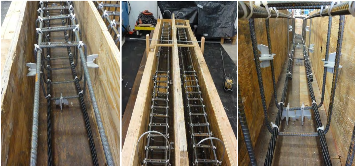
Figure 7.3-5 Placing the reinforcement cages in the formwork
