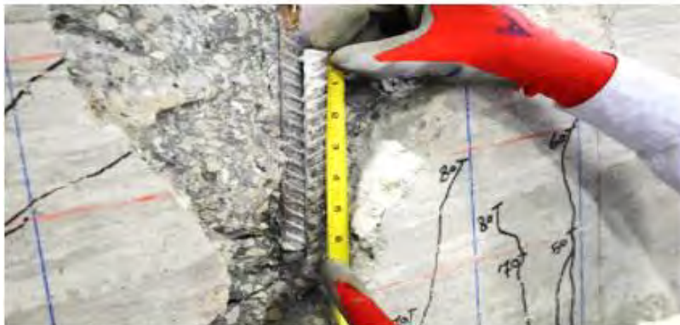
c) Slippage of the 7 in. (178 mm) spliced stirrups
