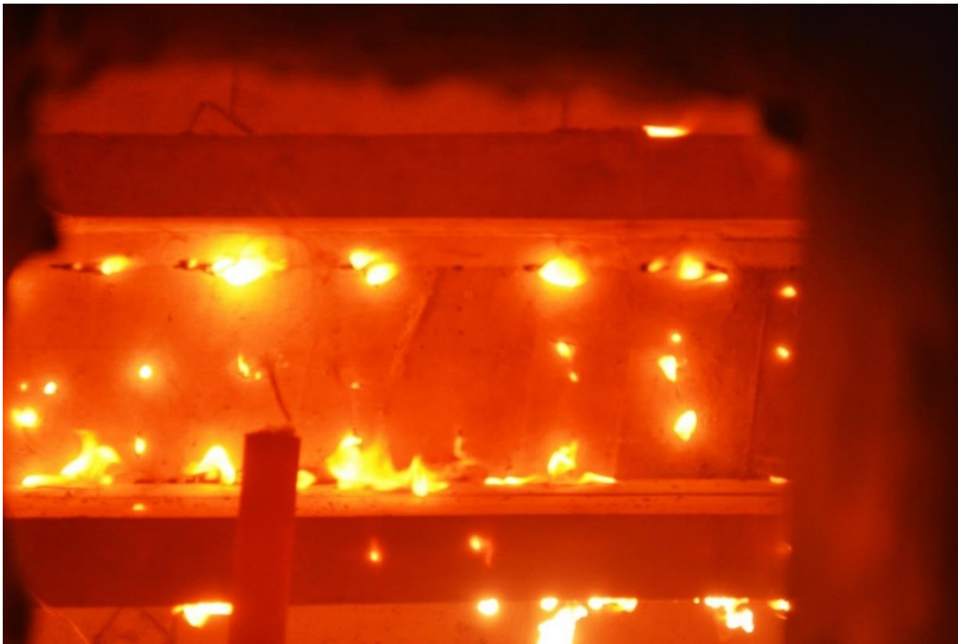
Figure 6.3-18 Burning of CFCC stirrups in Beam C72-14-1 during fire
