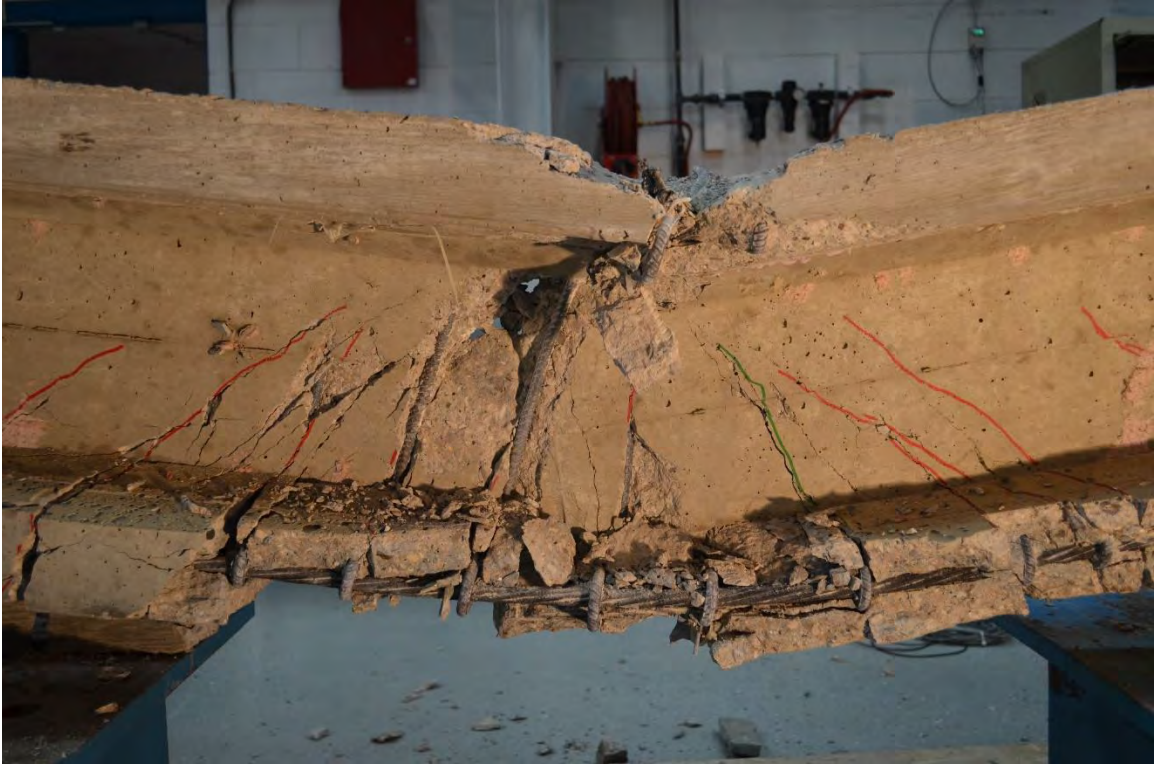
Figure 5.2-38 Close-up picture for CFCC strands in Beam H2 after failure
