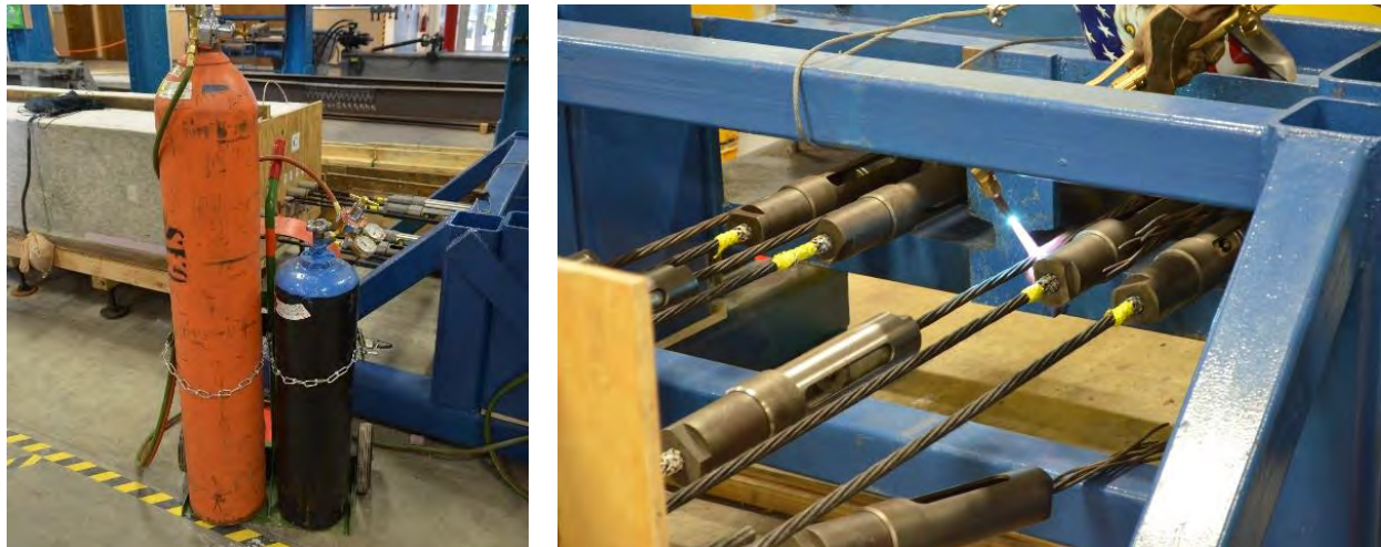
Figure 7.4-13 Releasing of prestressed strands
