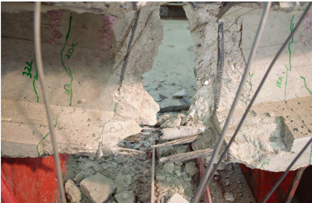
Figure 8.2-55 Ruptured prestressing strands at failure of Beam I-2
