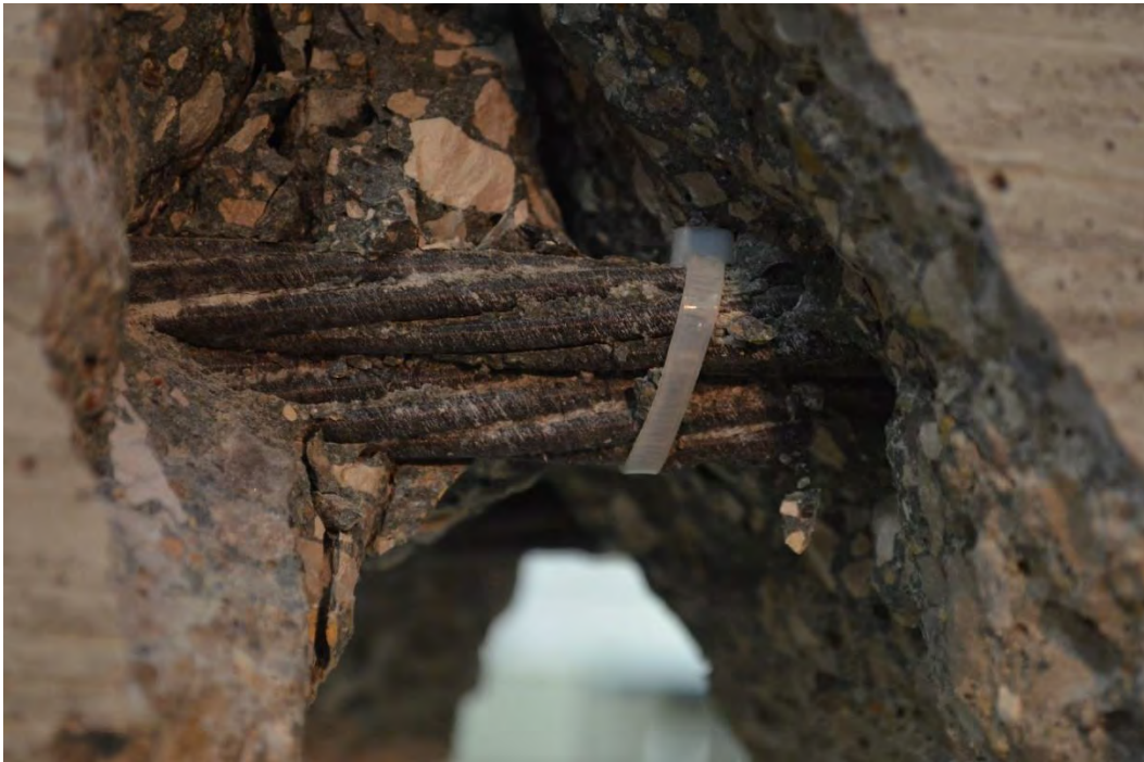
Figure 7.3-20 Close-up view of B3-0.5 showing CFCC slippage at the end of splice
