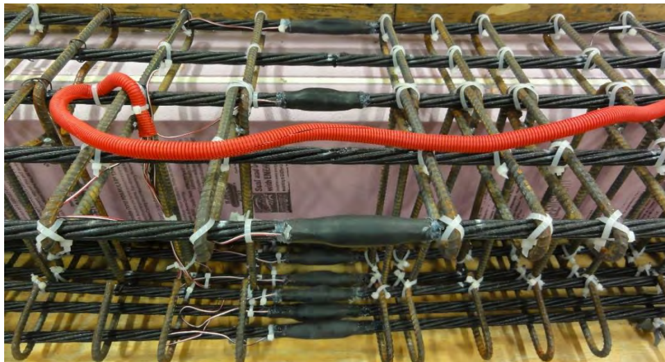
Figure 8.2-12 Installed strain gages on longitudinal reinforcement
