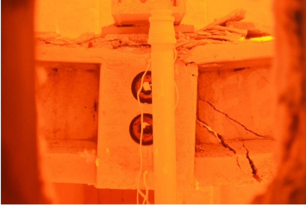
Figure 6.3-56 Close up view of mid-section of Beam C132-25-1 just after failure
