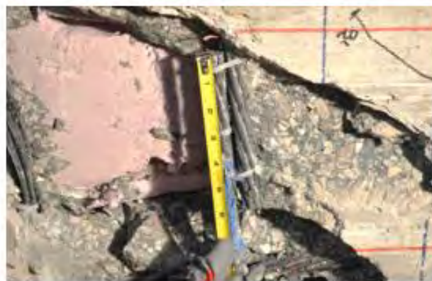
c) Slippage of the 7 in. (178 mm) spliced stirrups
