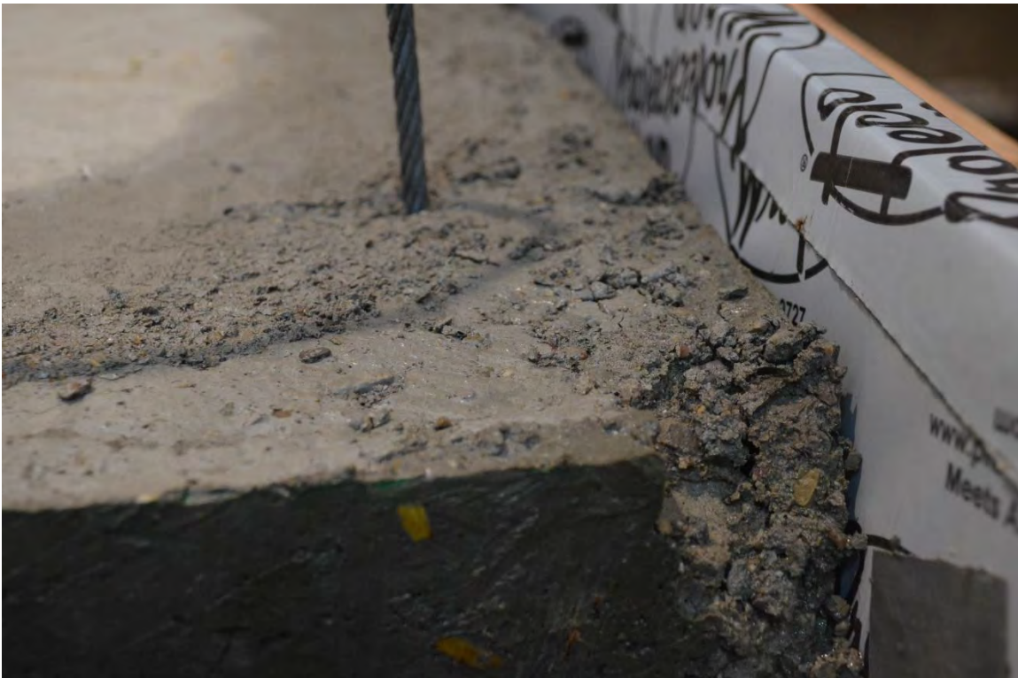
Figure 5.2-9 Deterioration of decked bulb T beams after exposure to 300 freeze-thaw cycles
