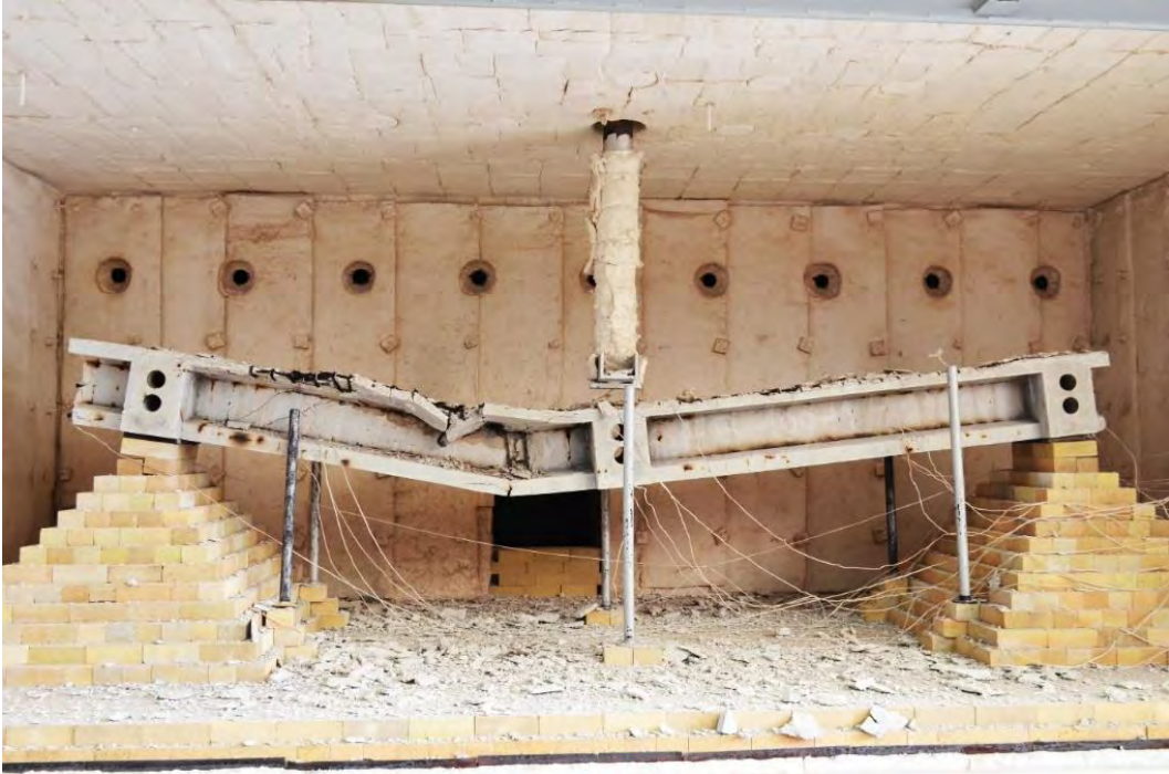
Figure 6.3-25 Beam C100-20-1 after fire
