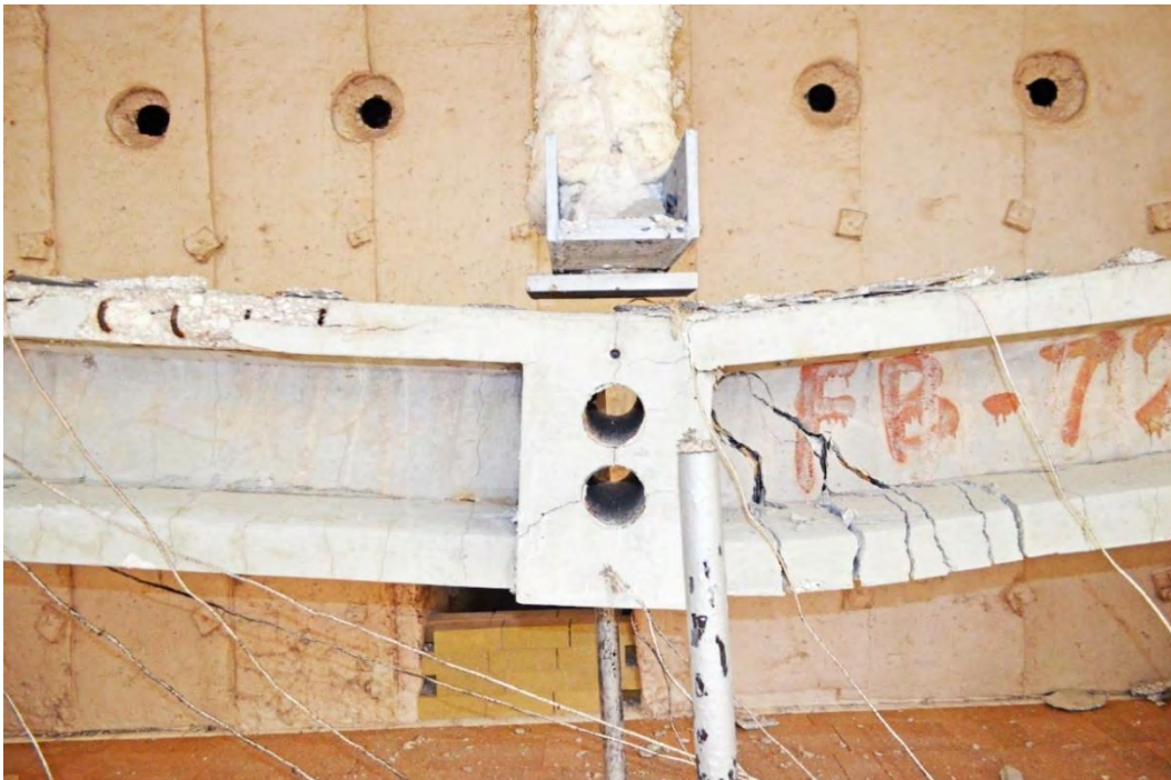
Figure 6.3-20 Close-up view of Beam C72-14-1 after failure
