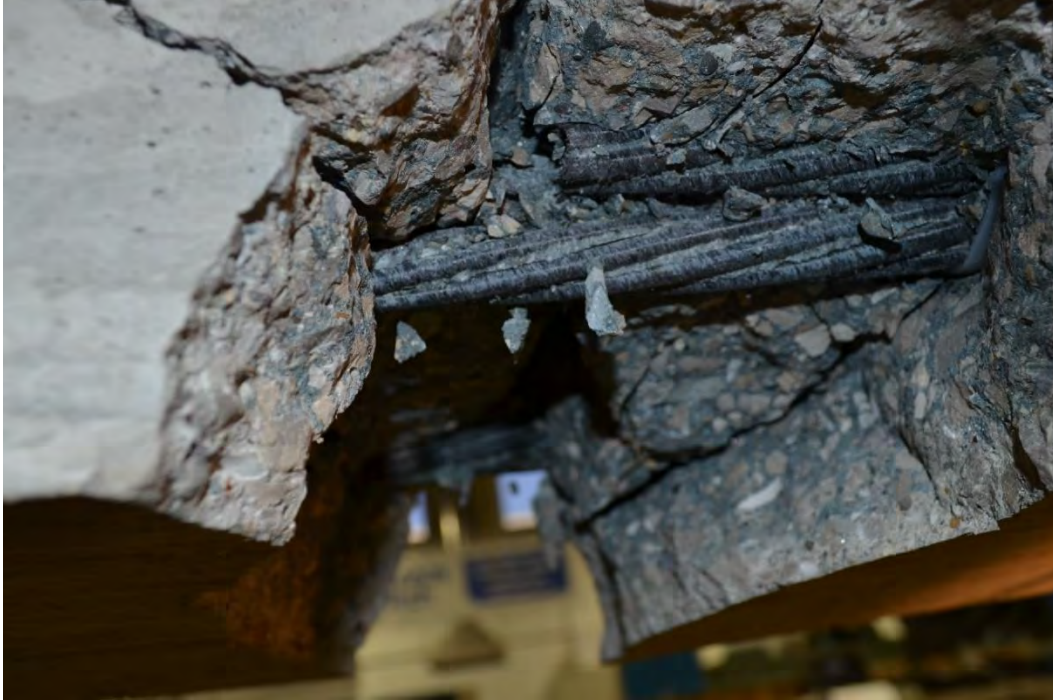
Figure 7.3-31 Close-up view of B2-0.6 showing CFCC slippage at the end of the splice
