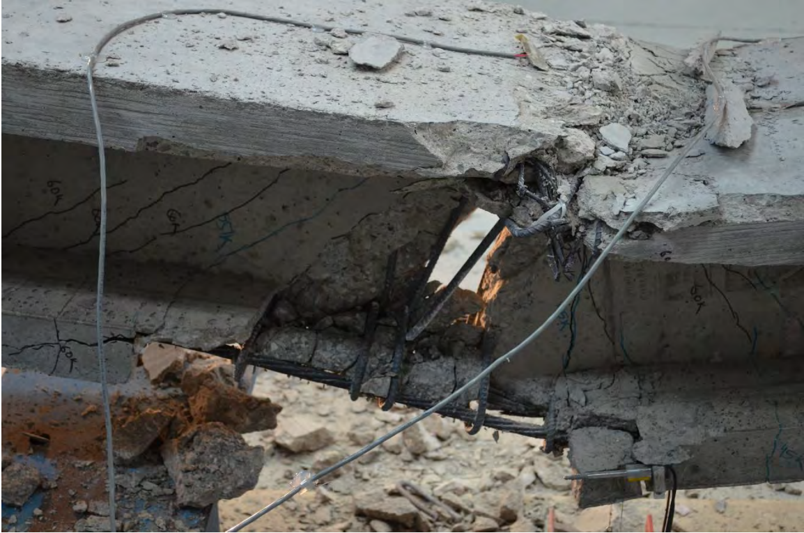
Figure 5.2-22 Rupture of strands and concrete spalling of Beam C2
