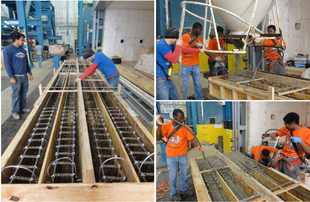
Figure 7.3-6 Casting the concrete in the test specimens
