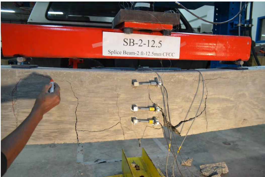
Figure 7.3-16 Failure of B2-0.5
