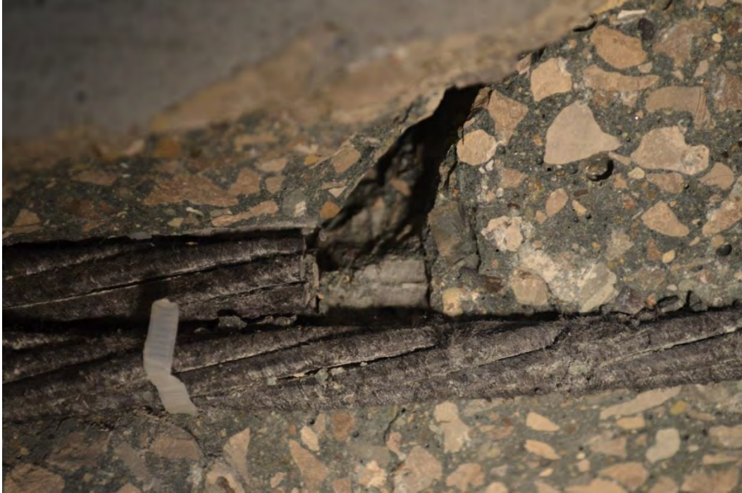
Figure 7.3-17 Close-up view of B2-0.5 showing CFCC slippage at the end of splice
