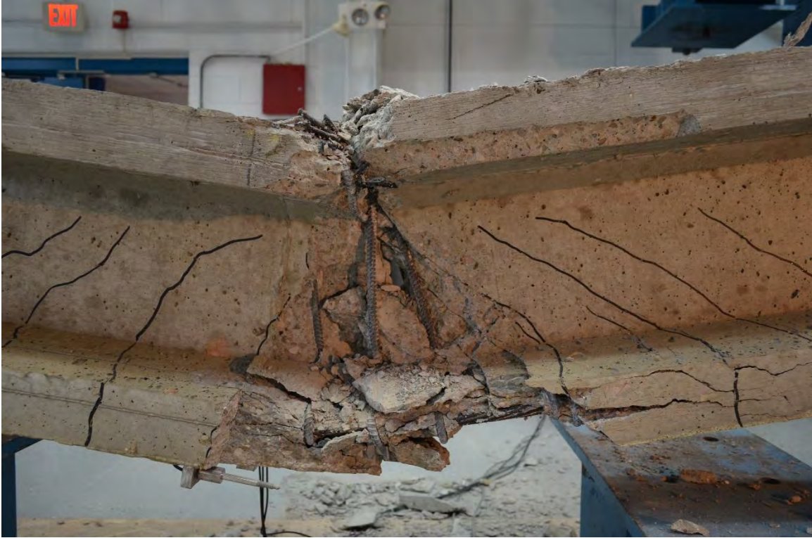
Figure 5.2-34 Close-up picture for CFCC strands in Beam H1 after failure
