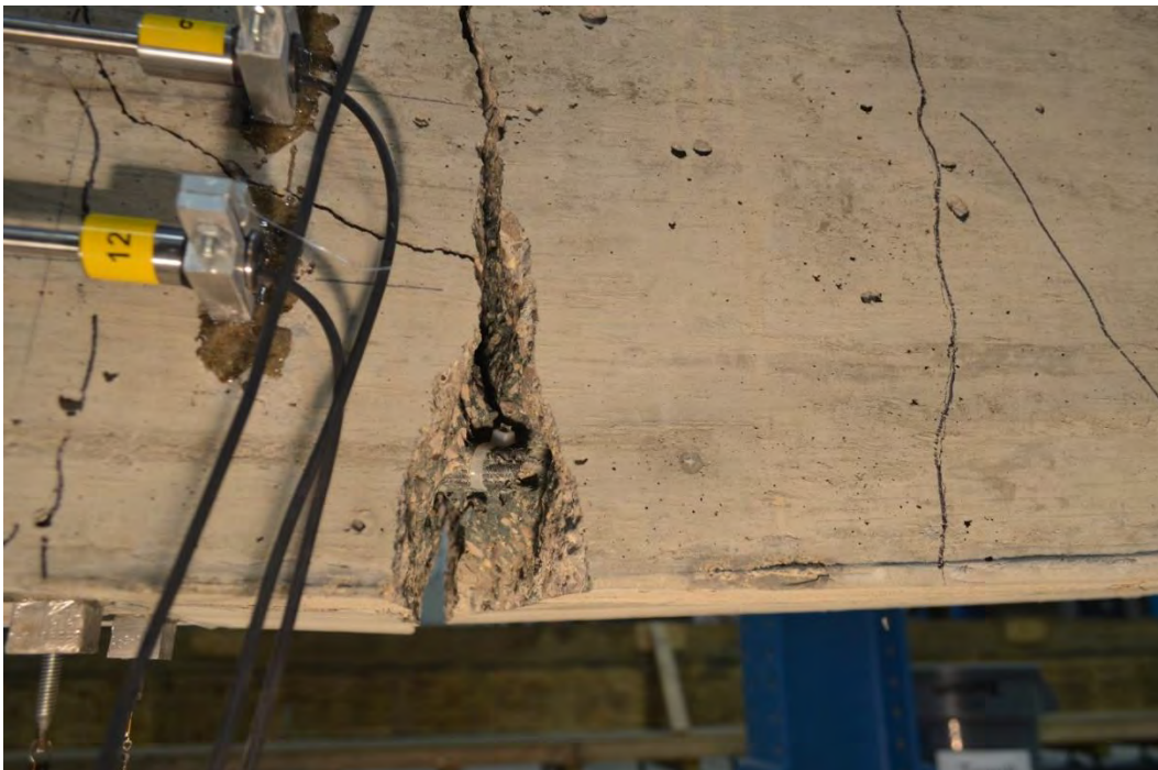
Figure 7.3-28 Close-up view of B1-0.6 showing the CFCC slippage at the end of the splice
