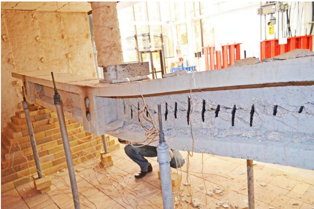
Figure 6.3-12 Rear view of Beam S132-25-1 after fire
