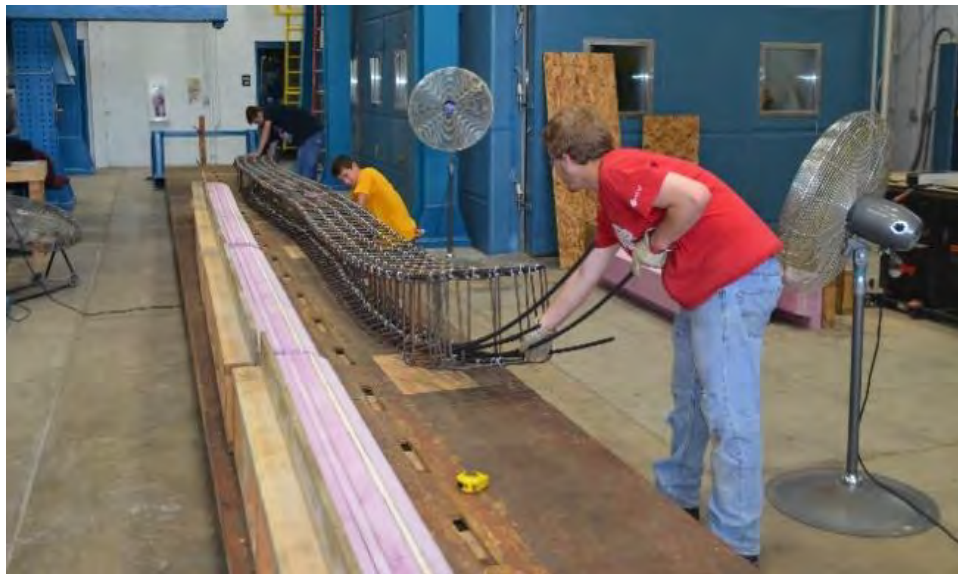
Figure 8.2-9 Bottom prestressing installation
