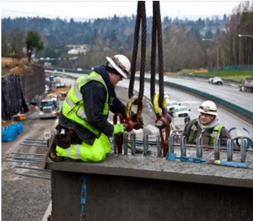
(a) PC girder being lifted using lifting loops
