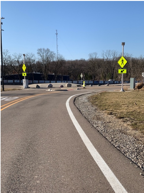
Figure 17: Mid-block pedestrian crossing with rapid RRFB.
