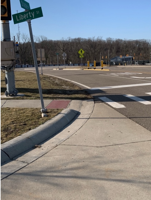
Figure 12: Examples of pavement transitions (asphalt to gravel and concrete to asphalt) and a low sloping curb.
