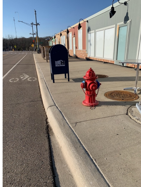
Figure 21: Examples of items regularly found along the roadside (mailbox, fire hydrant) and squared curbing.
