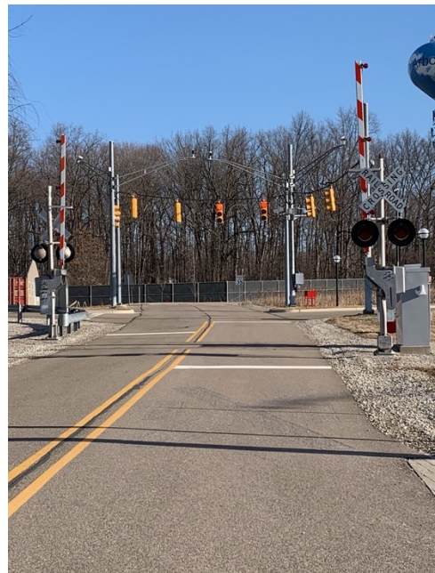
Figure 11: Gated railroad grade crossing and traffic signal heads suspended from metal poles.
