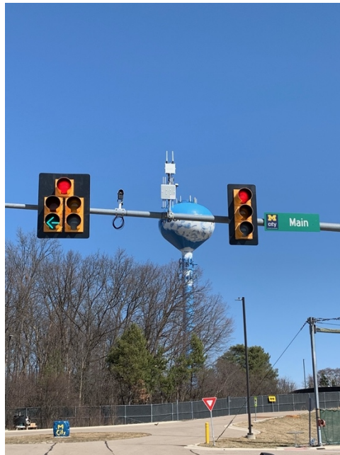
Figure 7: Infrastructure-to-vehicle communication radios and a vehicle detection camera.
