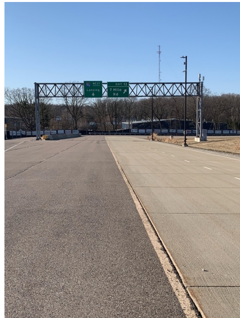
Figure 23: Concrete and asphalt pavement and highway signage on a truss.
