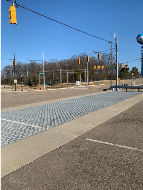
Figure 14: Section of grated metal bridge surface.
