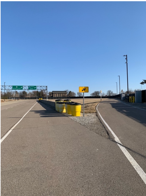
Figure 22: Exit ramp with metering, crash attenuators, Jersey barrier, and truss-mounted signage.
