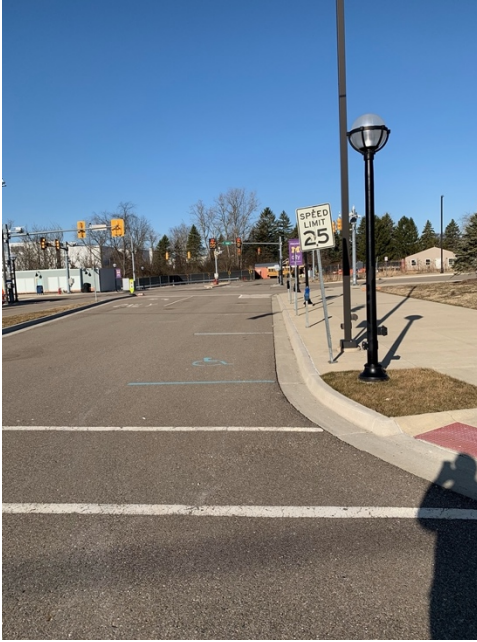
Figure 26: Parallel parking spots, including an accessible handicapped spot and post-mounted streetlights.
