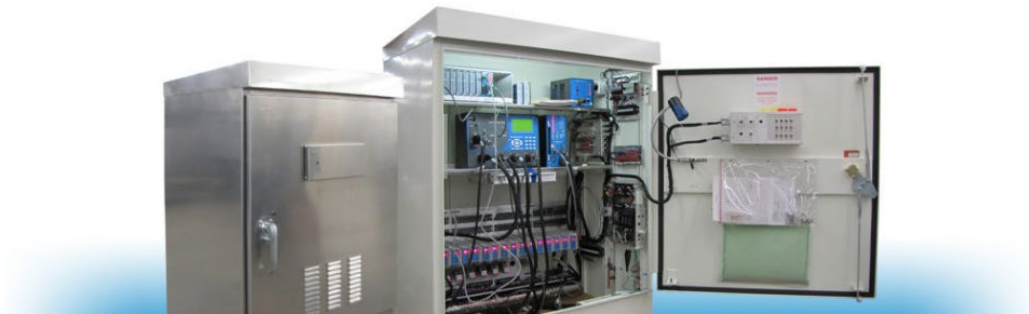
FIGURE 9. MDOT STANDARDS FOR TRAFFIC SIGNAL CONTROL CABINETS REQUIRE A MODULAR LAYOUT TO ALLOW FOR FUTURE TECHNOLOGIES
