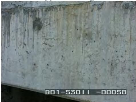
(c) Map cracking on exterior girder web
