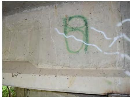
(b) Diagonal cracking – From girder bottom to girder top
