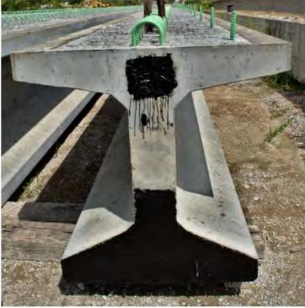
Cross-section of a bulb-tee girder with harped strands
