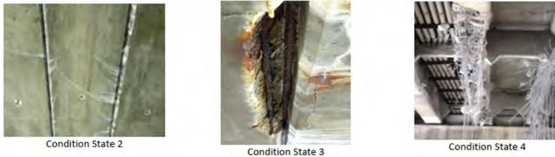
**Figure 2-9. CS Table 2 for PSC elements with supplemental information for inspectors (MiBEIM 2017)**
