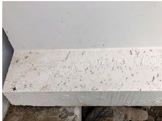
(b) Epoxy injected and repaired cracks
