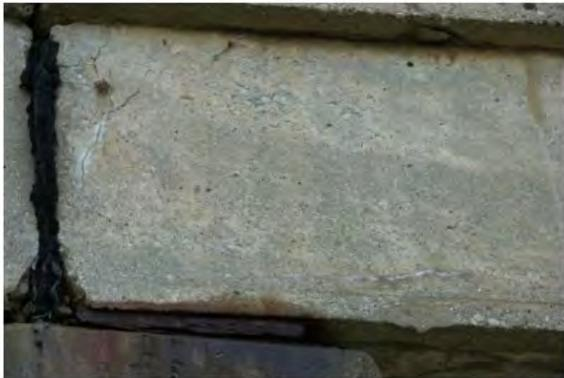
(a) End cracking
