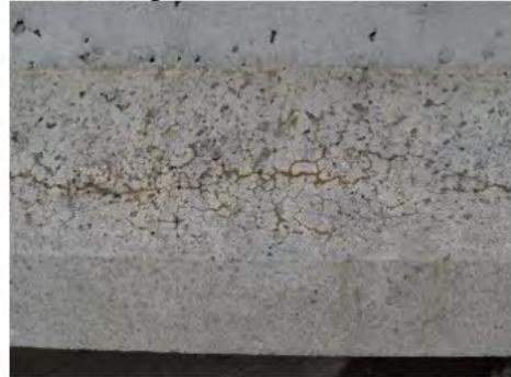
(b) Bottom flange map and longitudinal cracking
