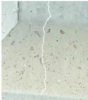
(a) Vertical cracking
