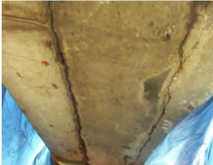
(a) Longitudinal cracking
