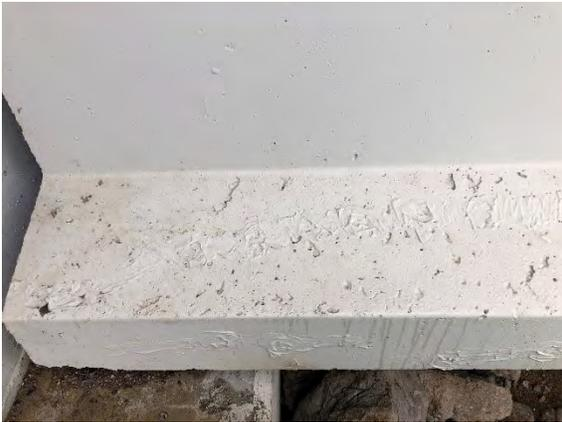
(b) Epoxy injected and repaired cracks
