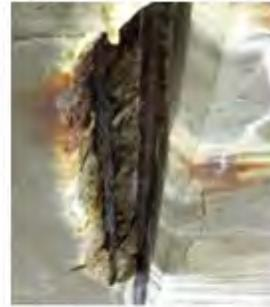
(c) Exposed prestressing with section loss
