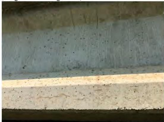
(c) Bottom flange showing longitudinal cracks
