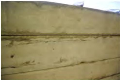
(a) Longitudinal cracks in box-beam bottom flange (Frosch et al. 2020a)
