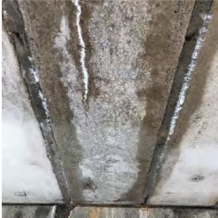
(a) Severe random cracking at beam soffit at beam end
