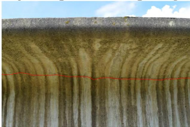
Longitudinal crack at the top of the web
