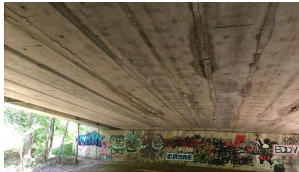
(b) Moist shear keys and longitudinal cracking
