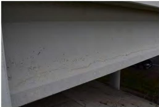
(c) Wide longitudinal cracking
