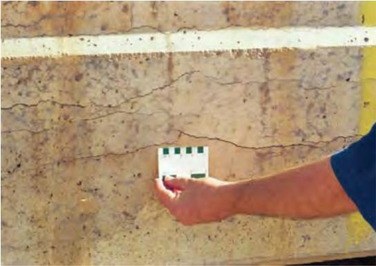
b) PC box beam cracking
