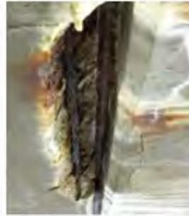
(c) Exposed prestressing with section loss
