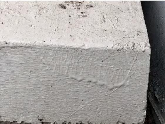
(c) Exposed cracks on top of the bottom flange
