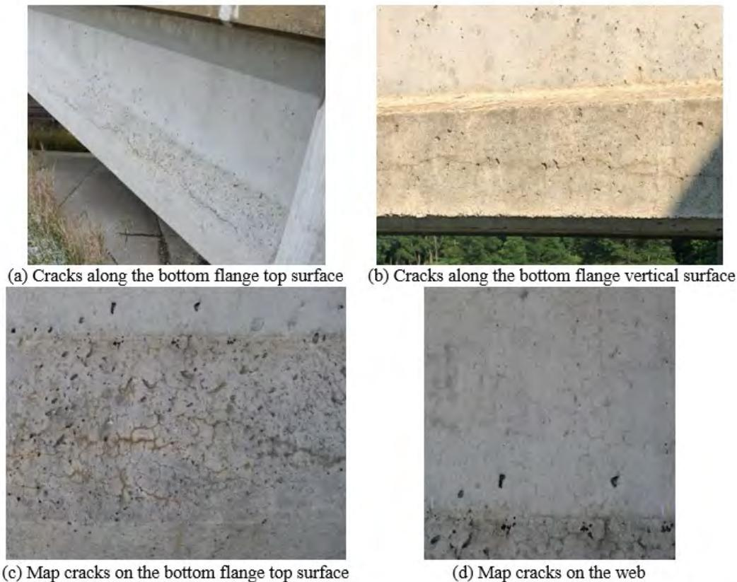
**Figure 3-9. Map and longitudinal cracks in PSC I-beams**
