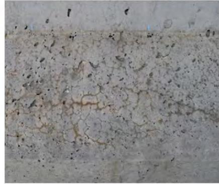
(b) Heavy map cracking on bottom flange
