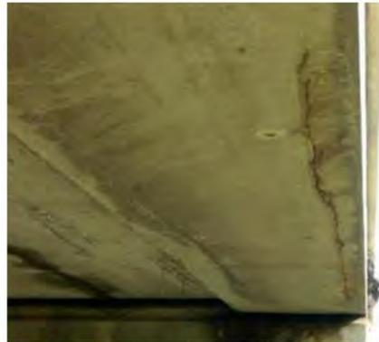
(b) Bottom flange longitudinal cracking
