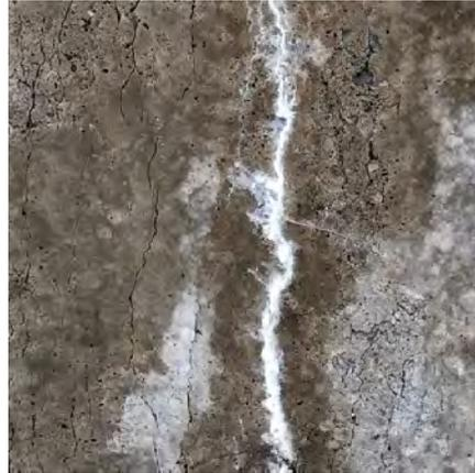
(b) Close up view random cracking at beam end
