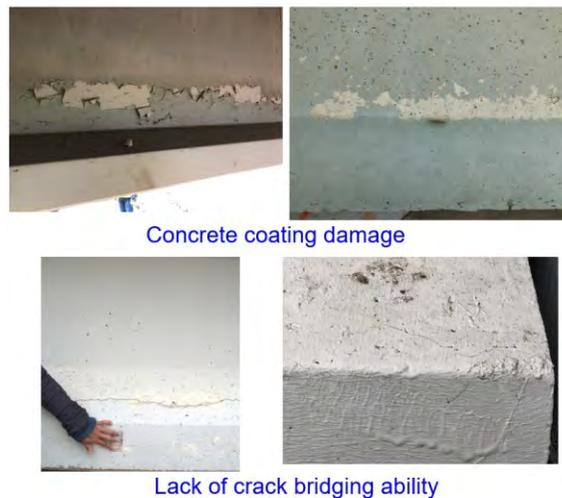
**Figure 3-12. Concrete surface coating damage and lack of crack bridging ability**
