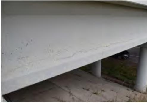
(a) Bottom flange longitudinal cracking
