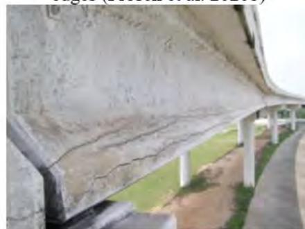
(f) Longitudinal cracks in I-beam bottom flange (Williams and Choudhuri 2010)
