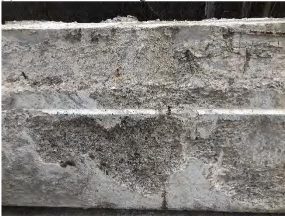
(c) Scaling on the web within beam span
