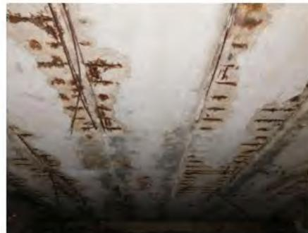
(b) Spalling, corrosion, and broken prestressing strands in box-beams (Frosch et al. 2020a)
