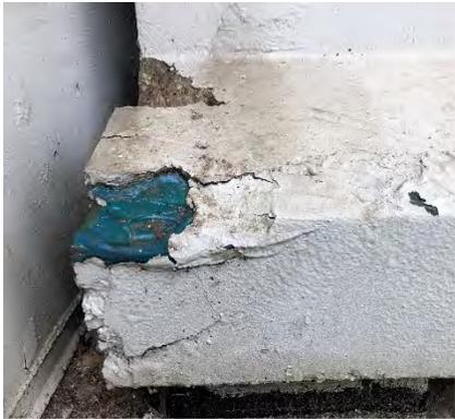
c) Beam end cracking
