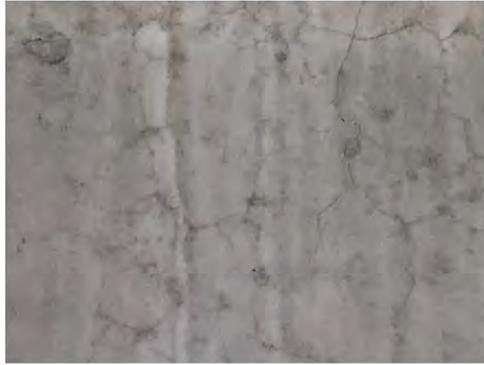
(a) Heavy map cracking on web
