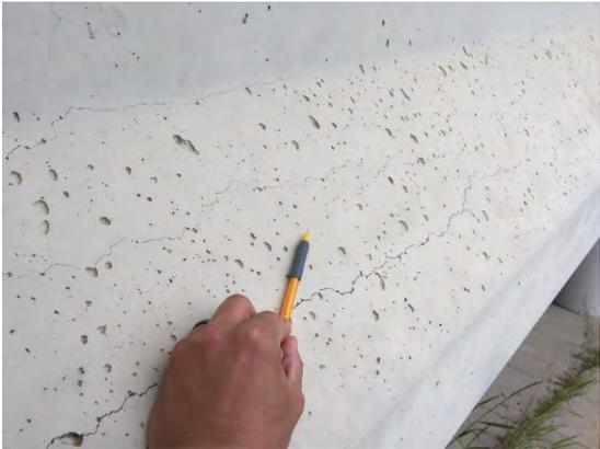
a) PC-I girder cracking
