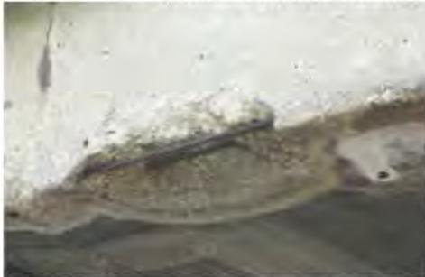
(b) Exposed prestressing with moderate spall
