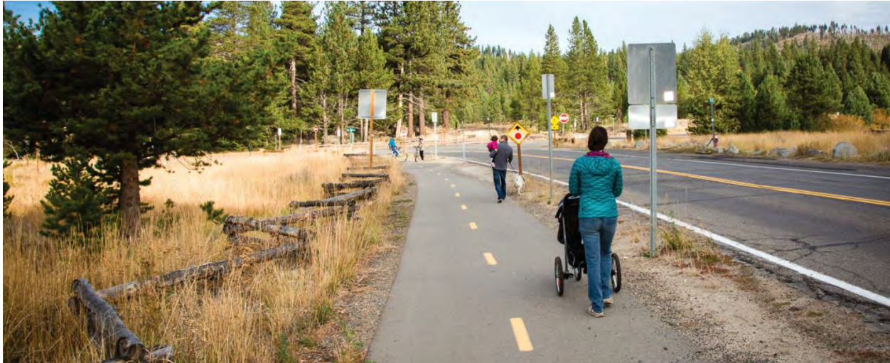
Figure 69. Example of a Sidepath in South Lake Tahoe, California [A.23]
