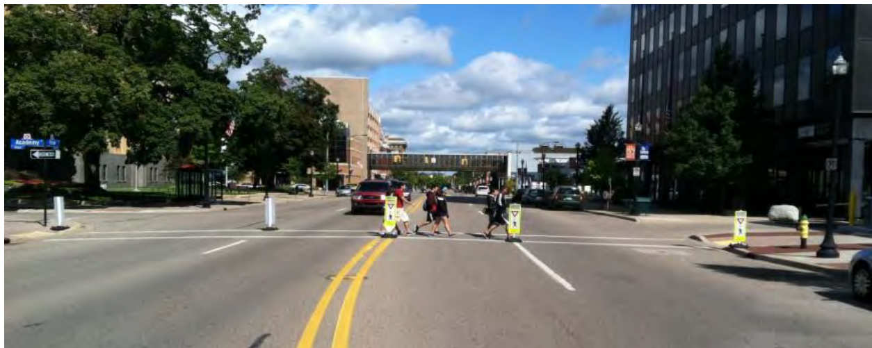
Figure 23. Example of R1-6 Signs Used as a Gateway Treatment in Michigan [C.47]
