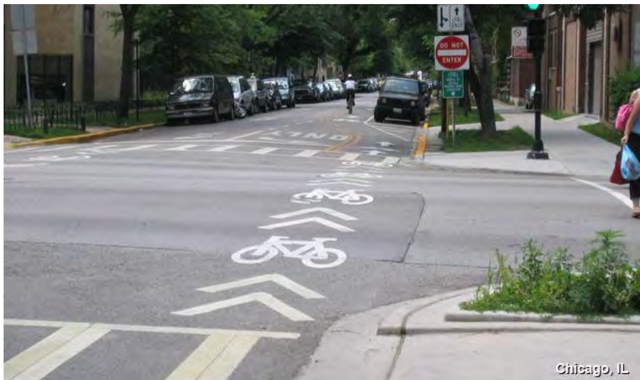
Figure 42. Example of Intersection Crossing Markings in Chicago, Illinois [A.11]
