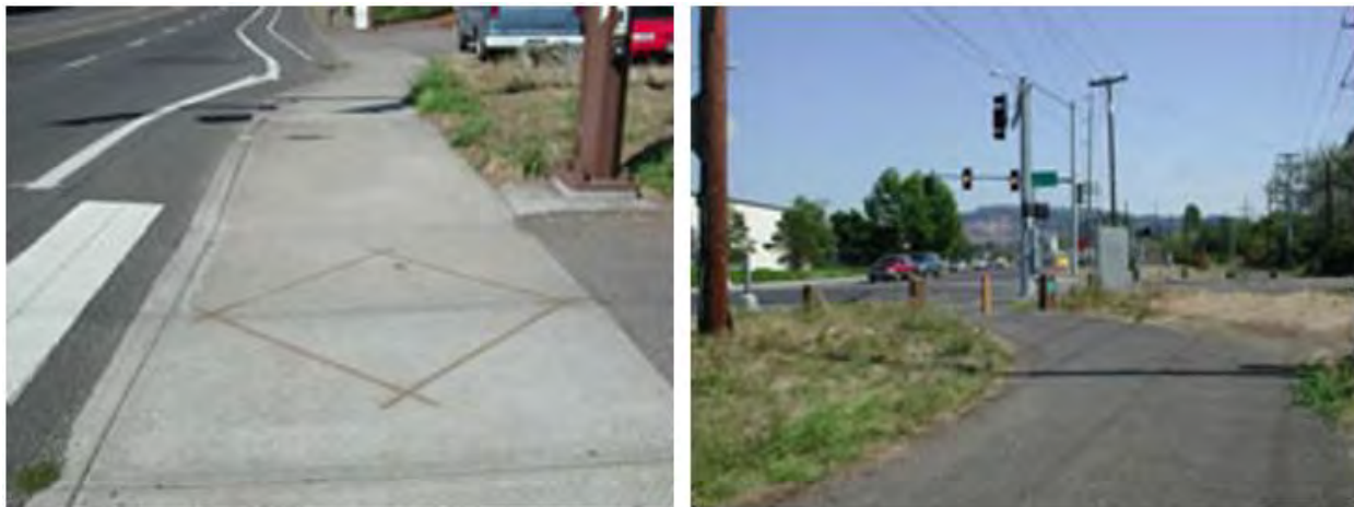
Figure 12. Example of Bicycle Loop Detectors installed at a Trail Crossing in Portland [1]
