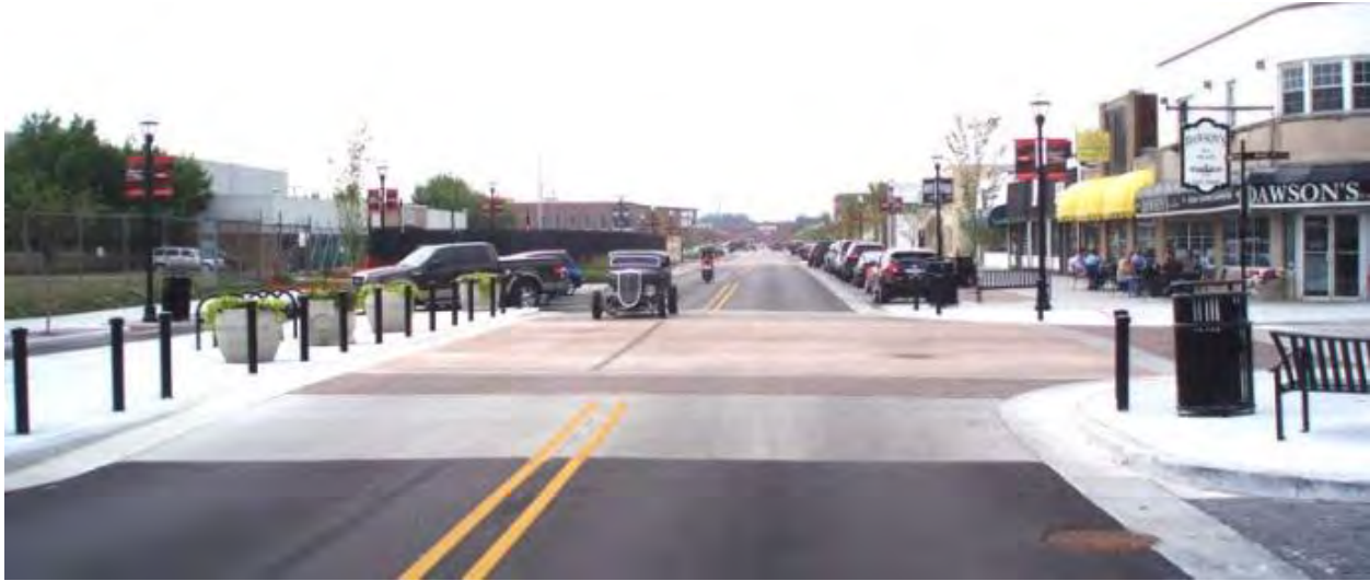
Figure 12. Raised Intersection Example from NACTO [A.13]
