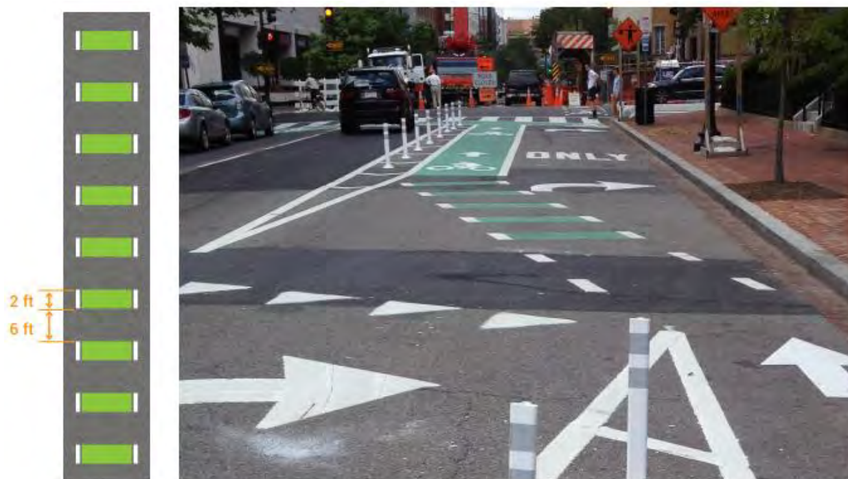
Figure 54. Example of Green Pavement Markings Across a Mixing Zone in Washington, D.C. [A.11]
