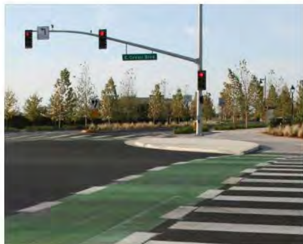
Figure 45. Protected Intersection Example from Davis, California [A.10]
