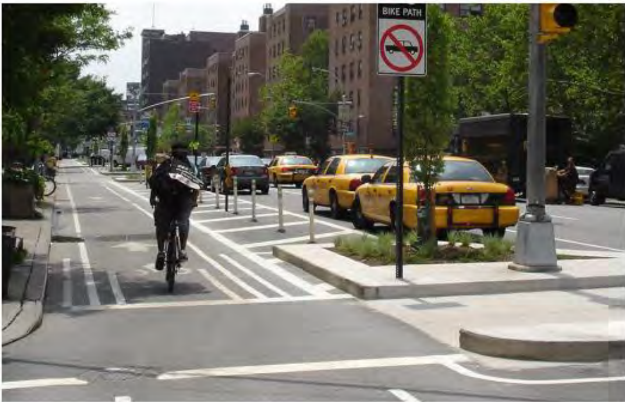
Figure 65. Example of Separated Bicycle Lane with Raised Curb Island in New York City [A.11]
