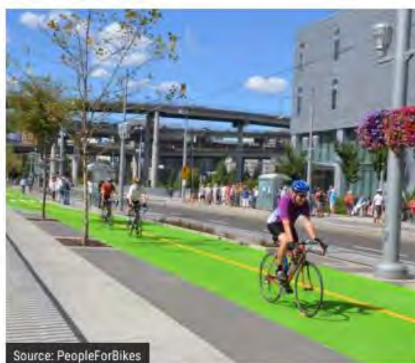
Figure 66. Example of Separated Bicycle Lane from Portland, Oregon [A.10]
