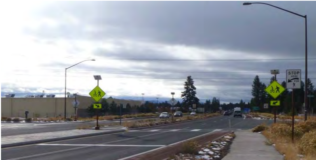
Figure 27. Example of a RRFB Installation in Oregon [A.86]
