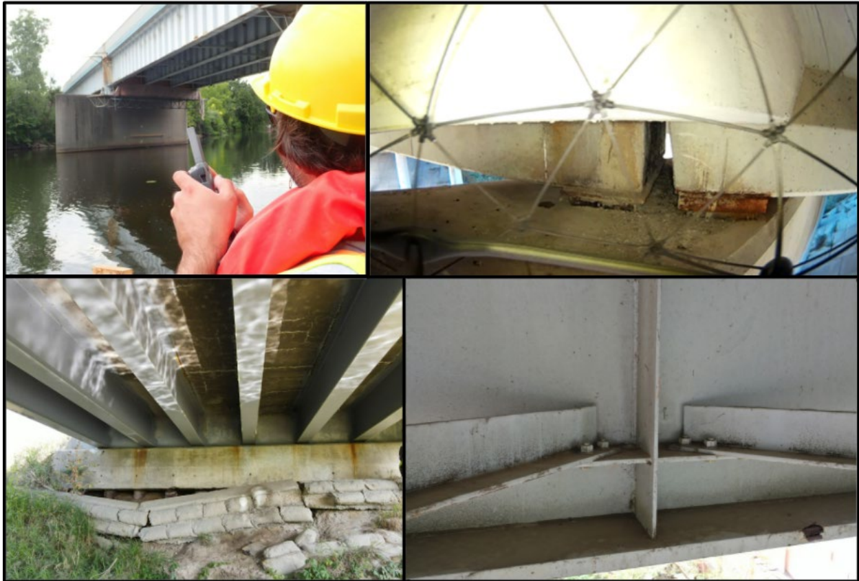
Figure 3.2.28: Example situations highlighting the utility of drones in surveying locations that are otherwise difficult to assess. A drone pilot captures imagery of bridge beams under I-96 at Grand River (top-left), a caged drone system is able to get very close to difficult to see areas (top-right), imagery of bridge substructure at Beyer Rd (bottom-left and bottom-right).
