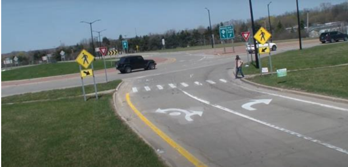
Figure 10 Staged Pedestrian Crossing Event at Roundabout Crossings
