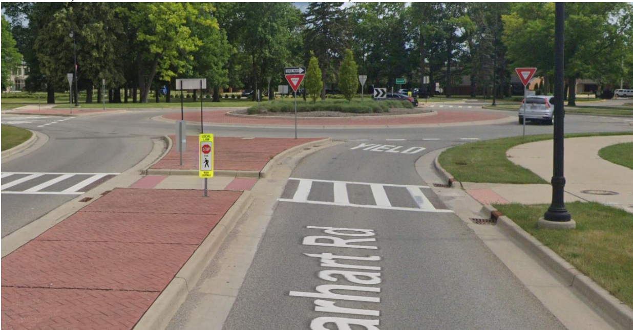
(c) In-street warning sign (Geddes at Earhart Road)
