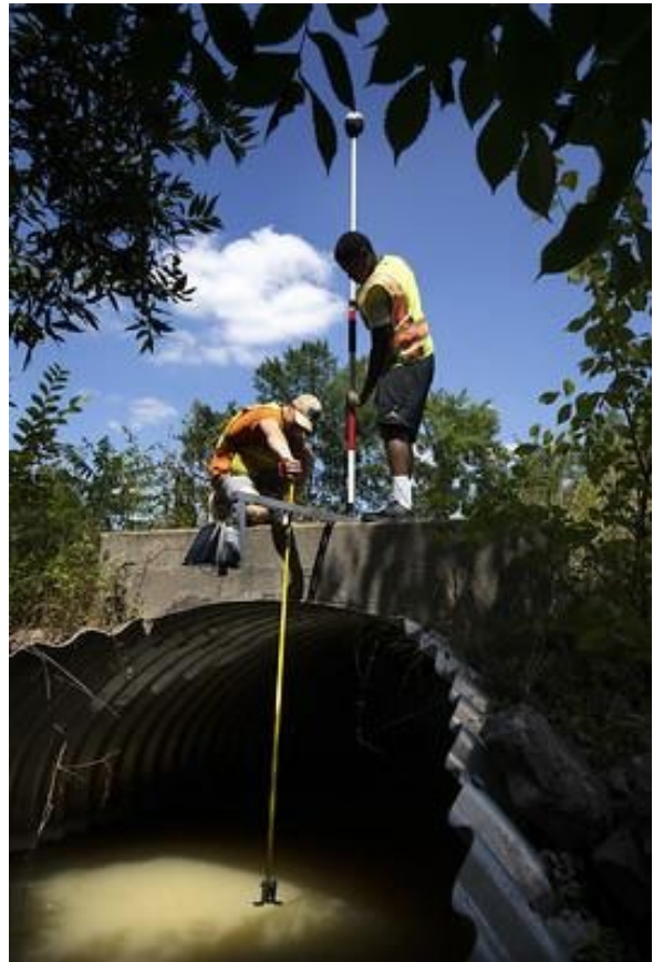
Figure 8. Mitchell Wojtowicz and Kenneth Ferrell deploying an Open-Storm Sensor
