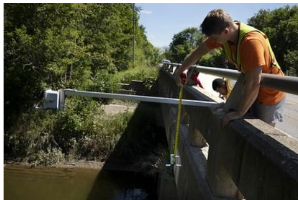
Figure 5. Mitchell Wojtowicz and Kenneth Ferrell deploying an Open-Storm Sensor
