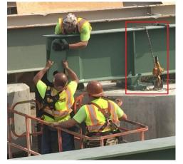
During construction, a chain-down system (outlined in red) securely anchors this steel I-girder to the bridge substructure and provides resistance to wind loading stresses.
