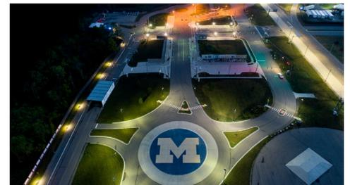
Mcity includes a variety of types and colors of lighting to help evaluate how connected and automated vehicles detect road and lane boundaries, as well as obstacles in the roadway.
