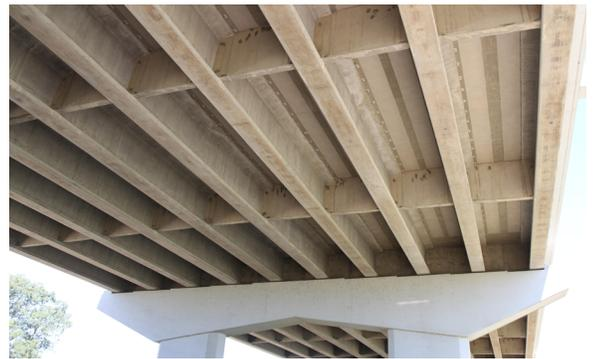
Diaphragms placed at intermediate locations (the members running left to right in this image) can help transfer loads; this research helped determine when they are needed. (Image courtesy of John A. Weeks III)
