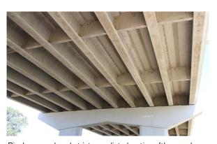
Diaphragms placed at intermediate locations (the members running left to right in this image) can help transfer loads; this research helped determine when they are needed. (Image courtesy of John A. Weeks III)
