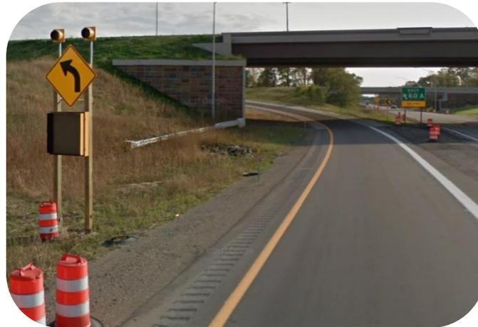
FIGURE A-11. EXAMPLE OF A CURVE SPEED WARNING SIGN
