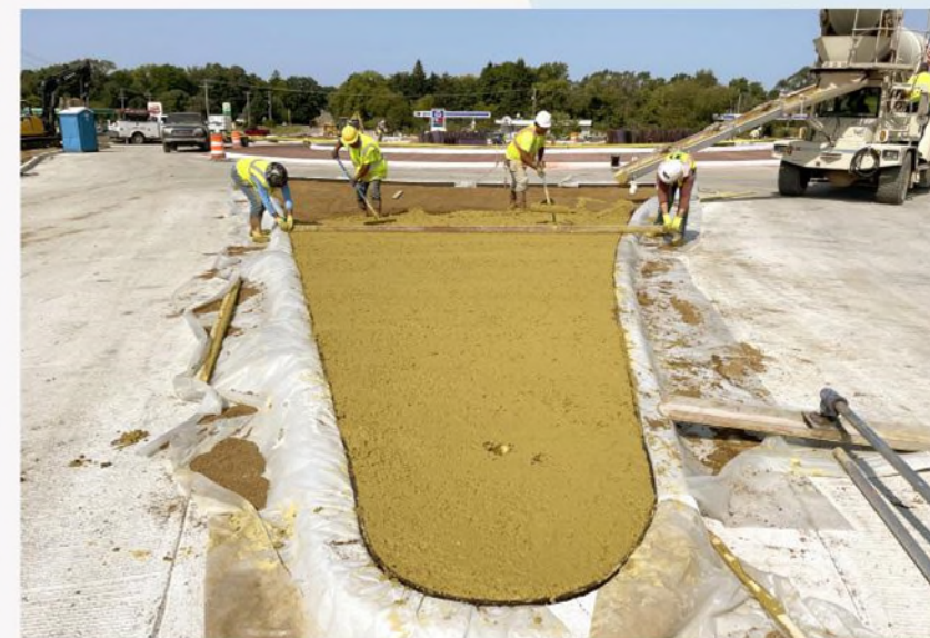
Decorative concrete placement at Michigan Avenue
