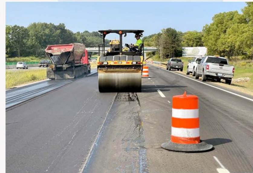
Resurfacing westbound I-94 west of Gibbs Road
