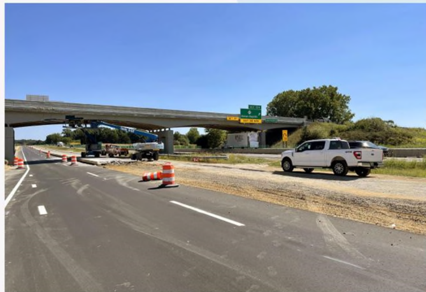
Superstructure repairs at M-99
