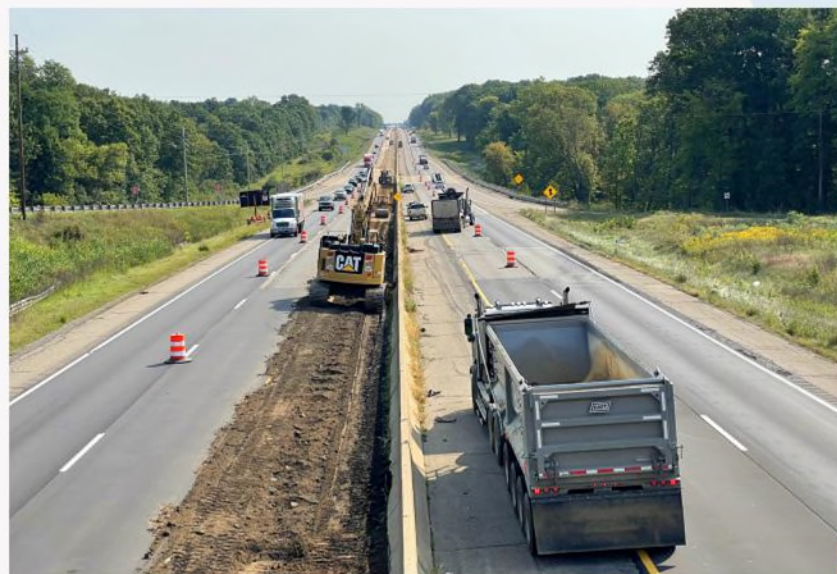
Rebuilding shoulder of westbound I-94 near Dearing Road
