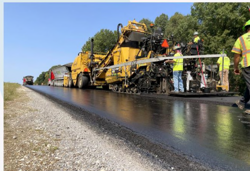
Resurfacing westbound I-94 west of Gibbs Road
