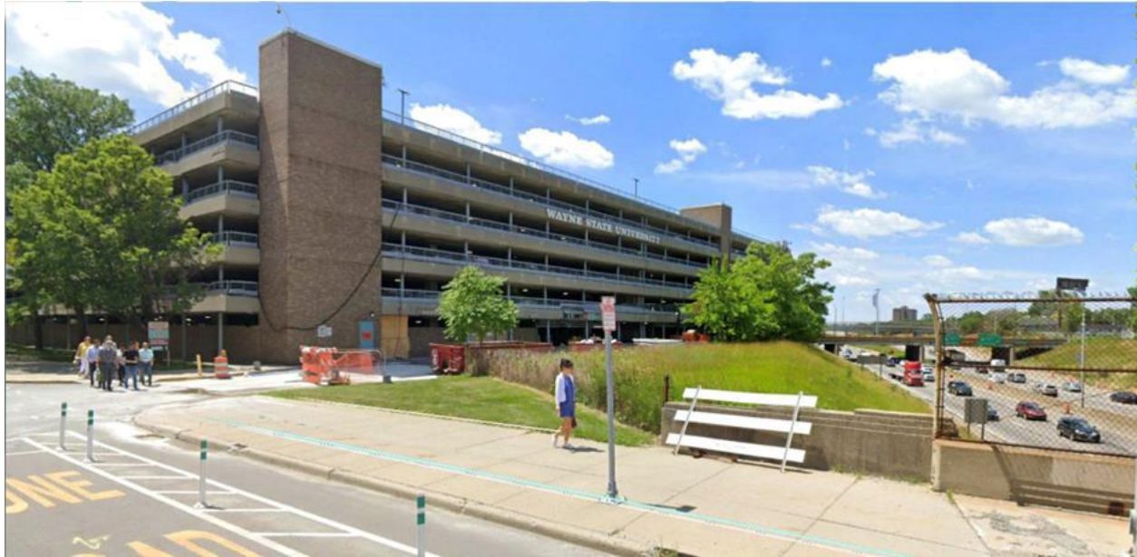
The southwest corner of the Cass Avenue bridge before construction.
