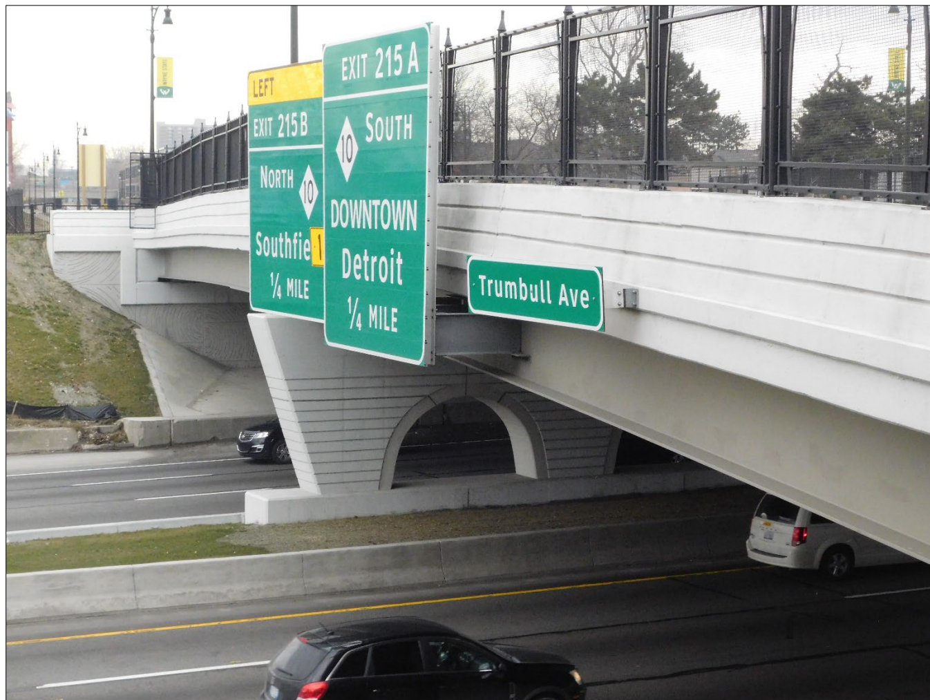
Figure 4-3: Trumbull Avenue Bridge Aesthetic Treatment
