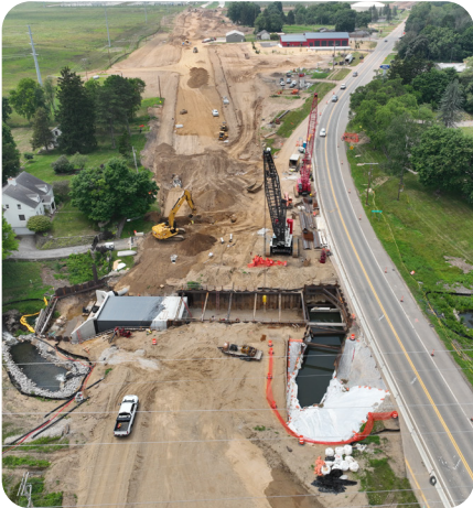
Image 2. Looking west at the new Bear Creek box culvert and road construction.
