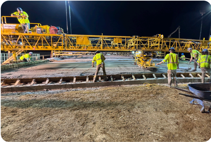
Image 1. The bridge contractor is pouring the concrete bridge deck, which will allow vehicular traffic to cross over the new southern Michigan Avenue bridge over I-69.
