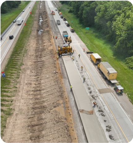
Image 2. I-69 paving of the concrete road driving surface.
