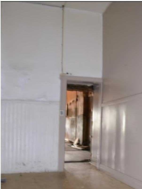
Left, Photo 38: Looking south, view of south and west walls of the storage room. Note: the west wall, which is the east wall of the men's restroom, lacks the bead board wainscot but carries the same cap molding.
