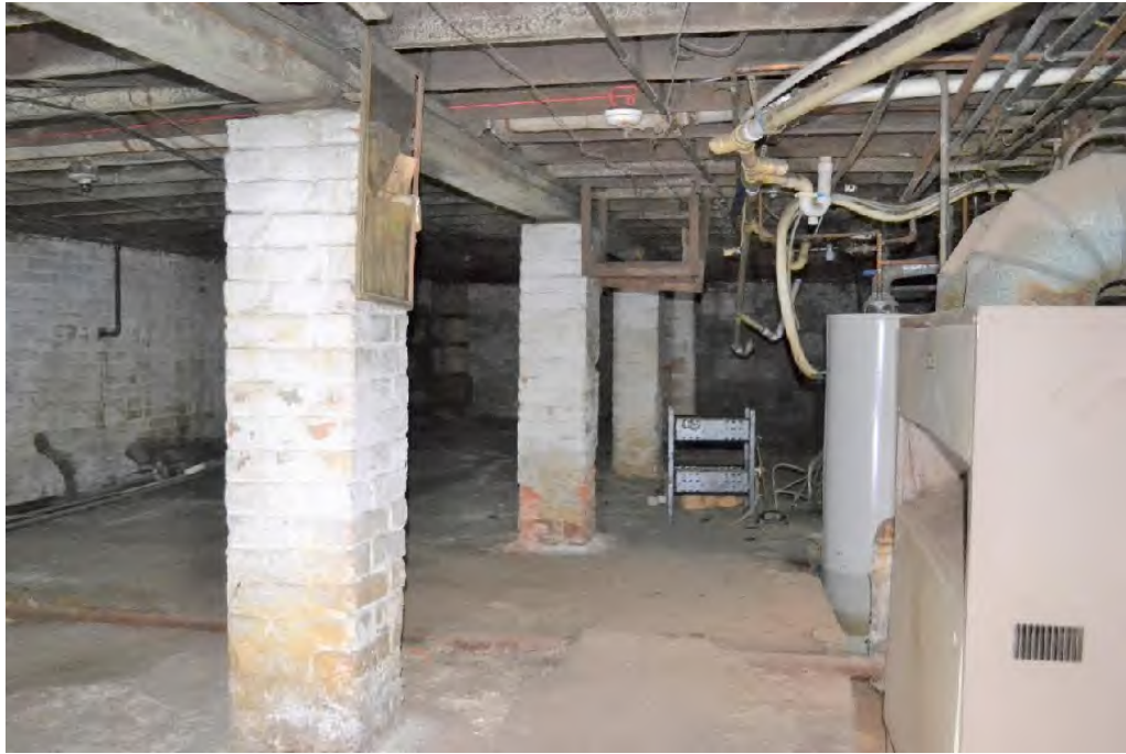
Photo 19: West basement, looking south. View from stairs (near north end of the basement). At the left is the central load bearing wall separating the west and east storefronts. Along mid frame are original brick posts supporting the floor beam. At right is the building furnace and a water heater (serving the first floor), the units were set in a shallow pit to accommodate their height. The floor, including the pit, were concrete finished.
