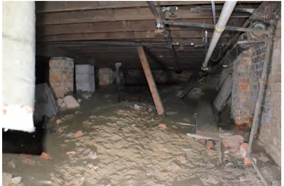
Photo 16: East basement, looking north. View shows the dirt and debris-filled north 2/3rds of the east basement. At left original brick and a replacement block posts support the floor beam
