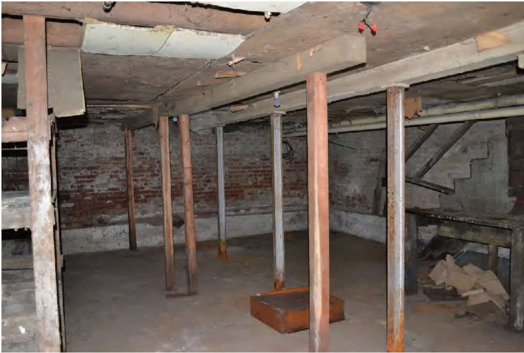
Photo 17: East basement, looking southwest. This view is towards the front (south) basement wall and shows the basement stairs and work bench to the right, storage shelving to the left and non-original wood and steel posts.
