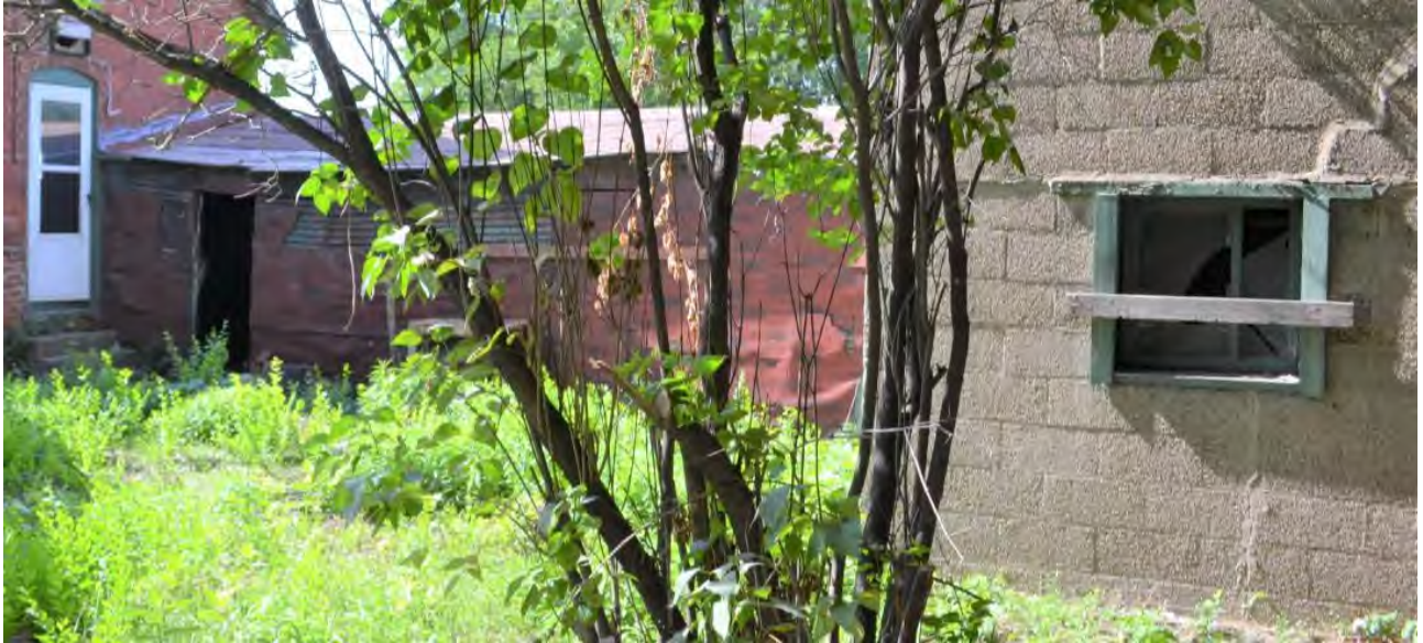
Photo 12 (detail, September 15, 2015): Looking west, southwest, showing the one-story wood-frame shed between the building and garage. Brick-look asphalt siding covers the clapboard cladding. At right is portion of the east (back) wall of the garage.
