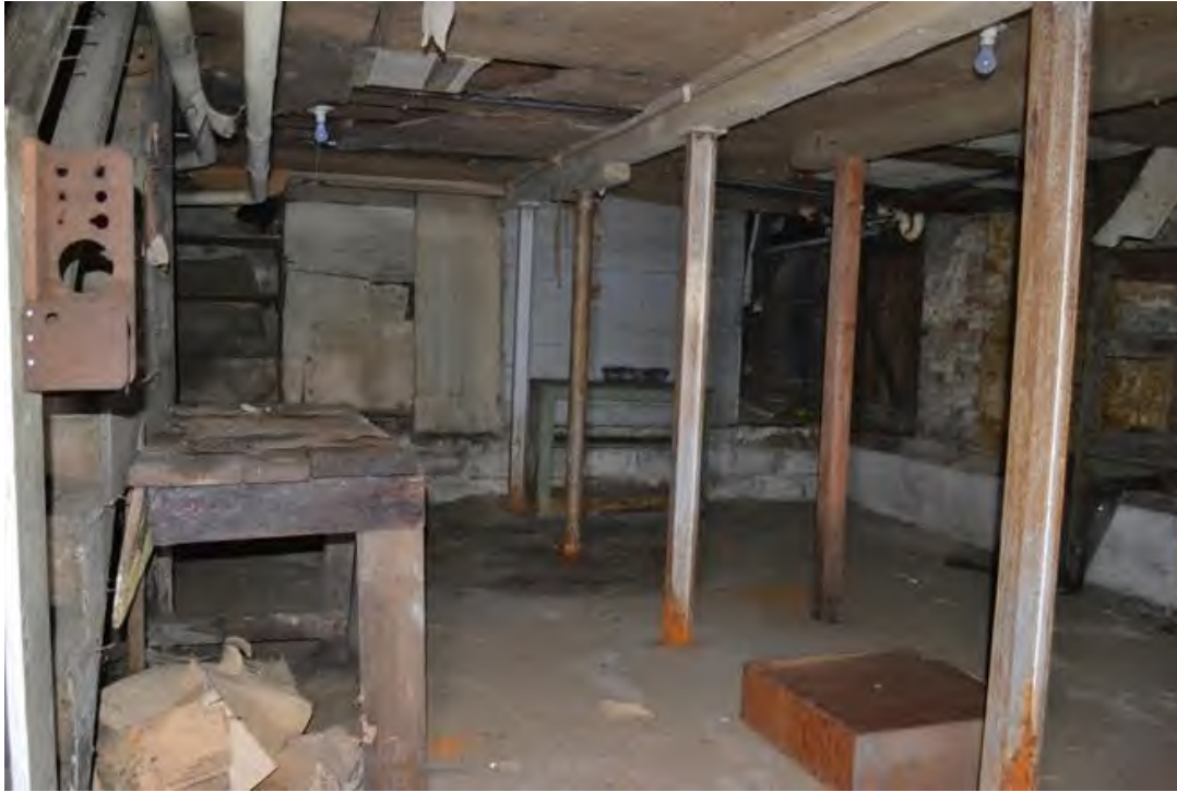
Photo 15: East basement, looking north. Most of the east basement is beyond the partition wall. At the far left (next to the work bench) are stairs to the first-floor dining room/east storefront. Note the non-original wood and steel posts.
