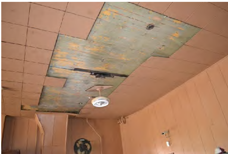
Photo 31 (detail, September 15, 2015): looking north, view of the original plank ceiling (barroom) where acoustic tiles are missing; although two different colors of paint are present it might be assumed the ceiling carried decorative tin cladding. The fluorescent fixture replaced an Art Deco milk glass pendant fixture that was typical of the décor during the Kovacs years. Above right, Photo 32, (detail, September 15, 2015):
