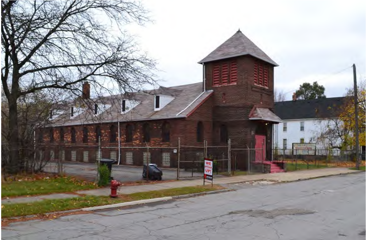
PHOTO 1: Looking southeast, showing the north (side) and west (front) elevations. Note the use of lighter-color replacement brick on the main level. (November 12, 2015)
