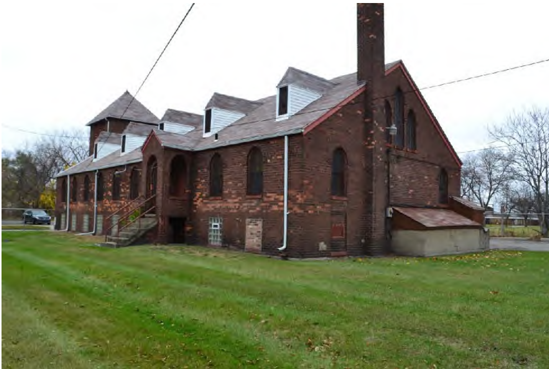
PHOTO 7: Looking northwest, showing the south (side) and east (rear) elevations. The open, gabled tower protects the side entrances to the upper and basement levels. (November 12, 2015)
