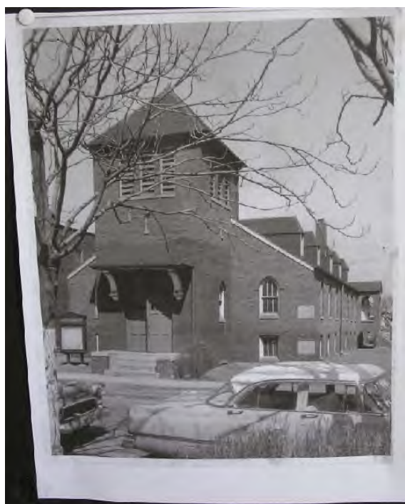
PHOTO 5, above: looking NE, view of the Main (west) and south elevations. Note side entry porch and belfry vents. The church has undergone very little change over the years. The main exception is the replacement of the lower level windows and replacement of the stoop roof supports. (September 25, 2007.)
