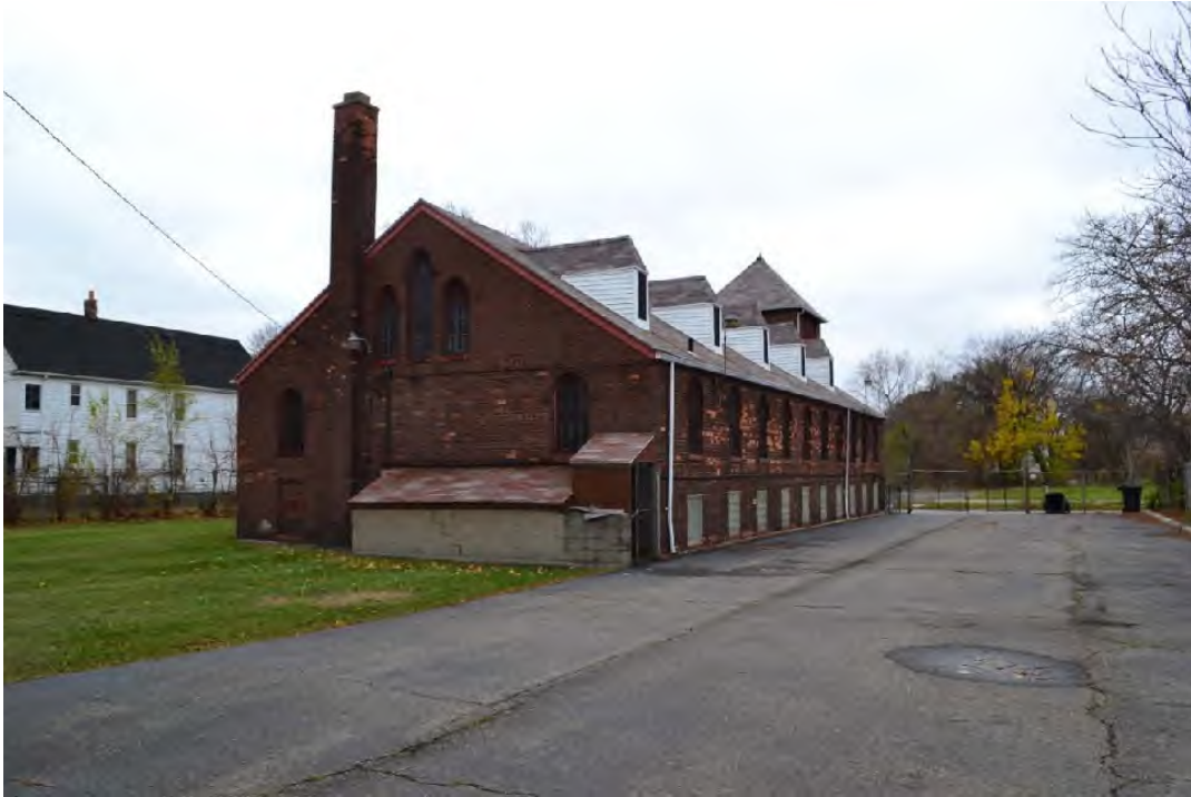
PHOTO 6: Looking west, the east (rear) and north (side) elevations. The low shed roof addition accesses the basement utility/furnace room and kitchen, the taller shed roof structure houses the steps into the addition. (November 12, 2015)
