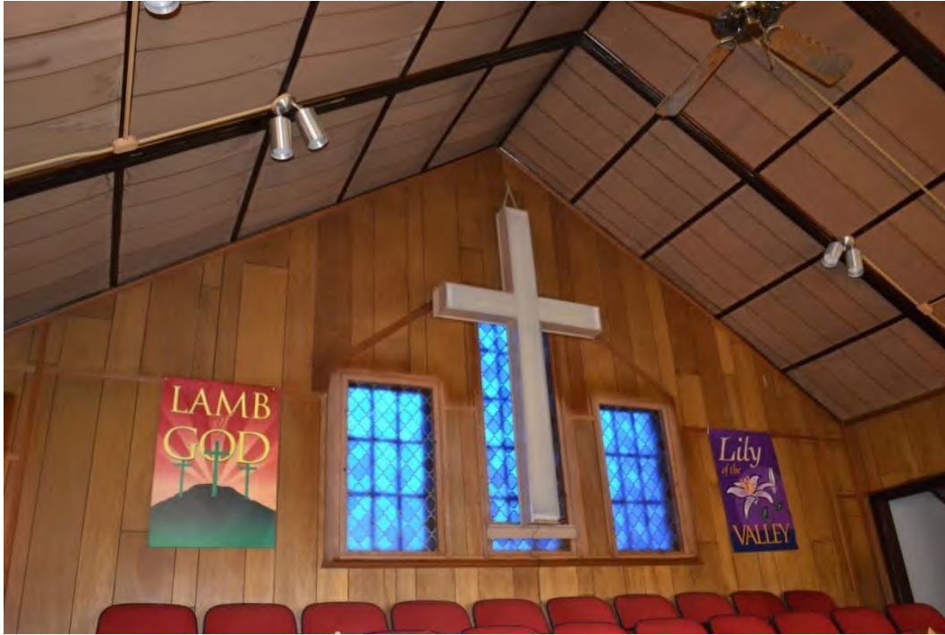
PHOTO 19: Looking east, showing the tri-partite window (a 15- light center sash flanked by nine light wood sash) at the back of the church. The interior side of the windows was modified to show flat arches, whereas on the exterior the windows still show the original Gothic arch configuration. (November 12, 2015)
