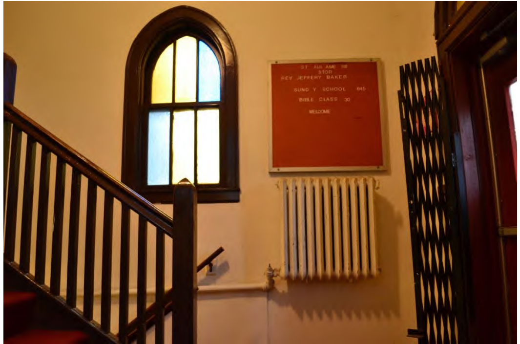
PHOTO 12, right: view of the south wall of the lobby showing the three-over-three window, simple Arts-and-Crafts railing and wall-mount radiator (November 12, 2015)
