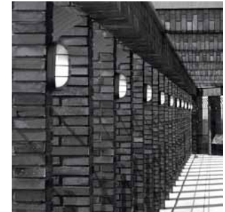
Bega #2841S bulk-head type lights for the Perimeter Walls
