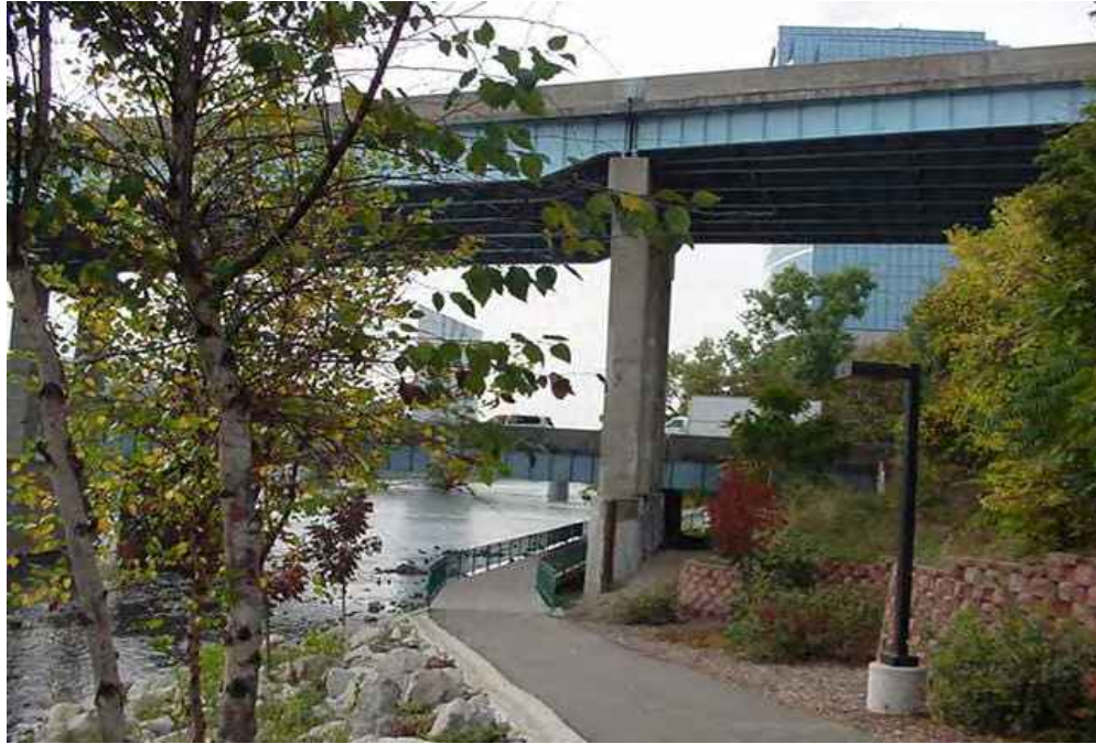
Figure 6.3 - West Side River Walkway
