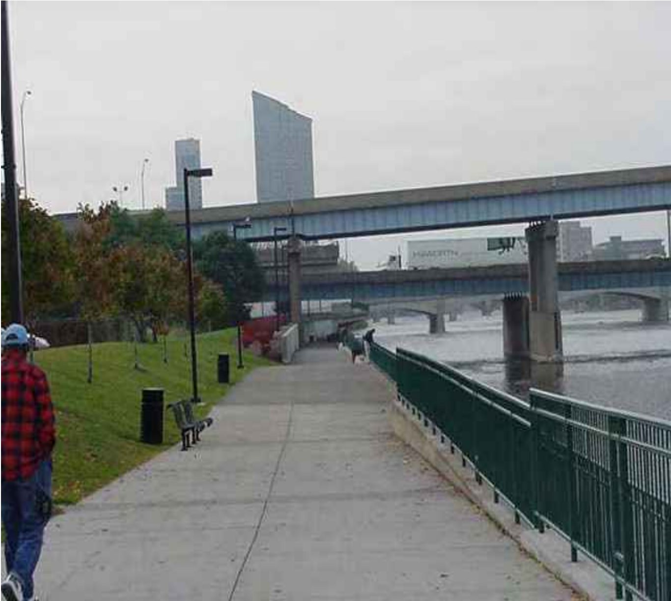
Figure 6.2 - Grand River Walkway
