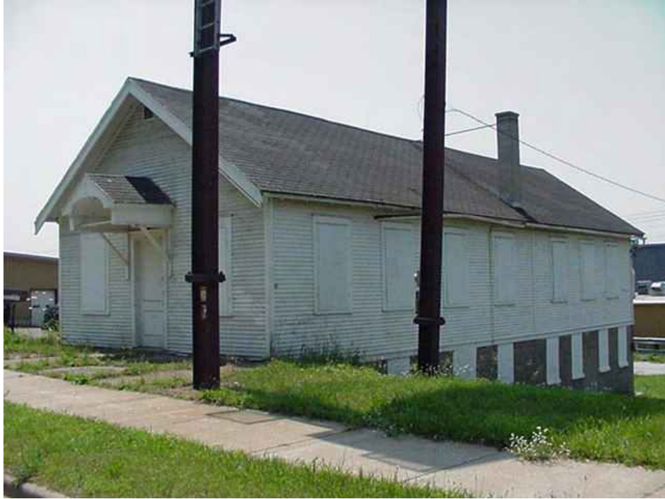
Figure 2.2 Former Ionia Avenue Mission Hall—views of front façade and north elevation.
