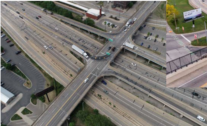
Aging pavement and bridge condition at Wealthy Street interchanges
