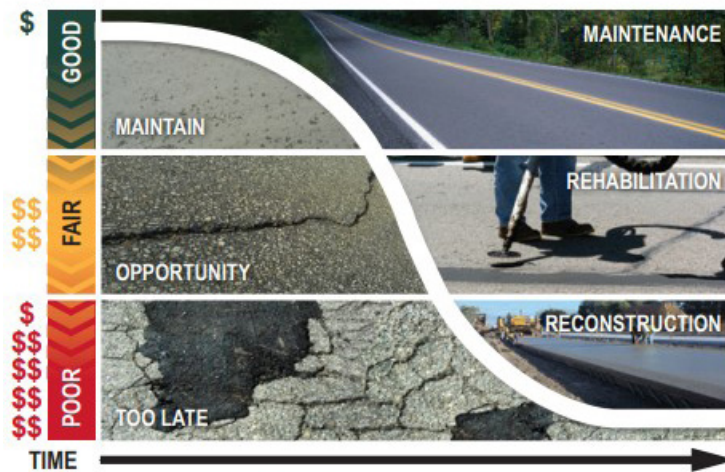
ROAD DETERIORATION (Image source: Macomb County Department of Roads)
