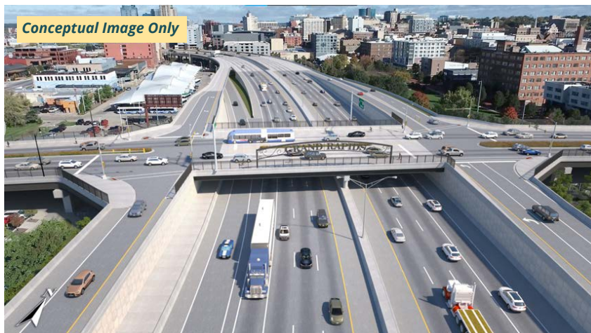
Designs of Wealthy Street Underpass and Overpass Aerial View in Option 3A
