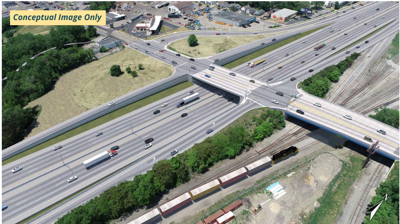
FIGURE 5-7. Burton Street Interchange: Diamond
