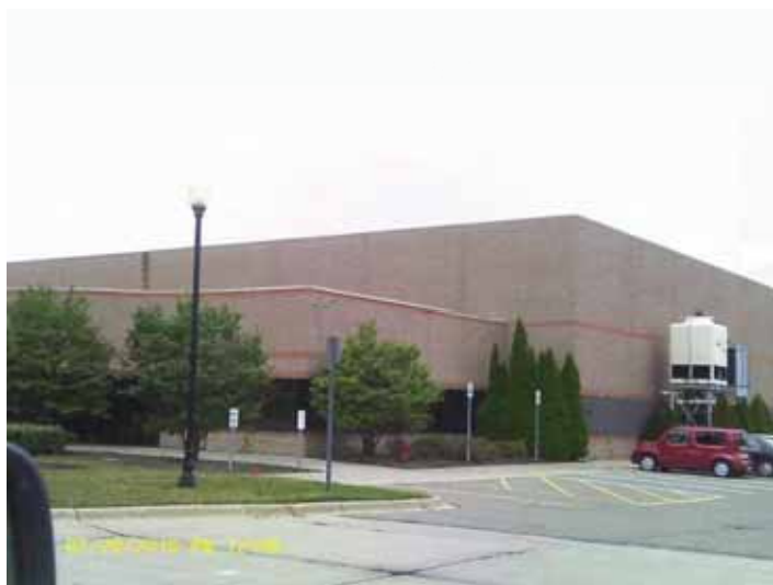
Industrial: Axxis Corporation – 7375 Commerce Boulevard
