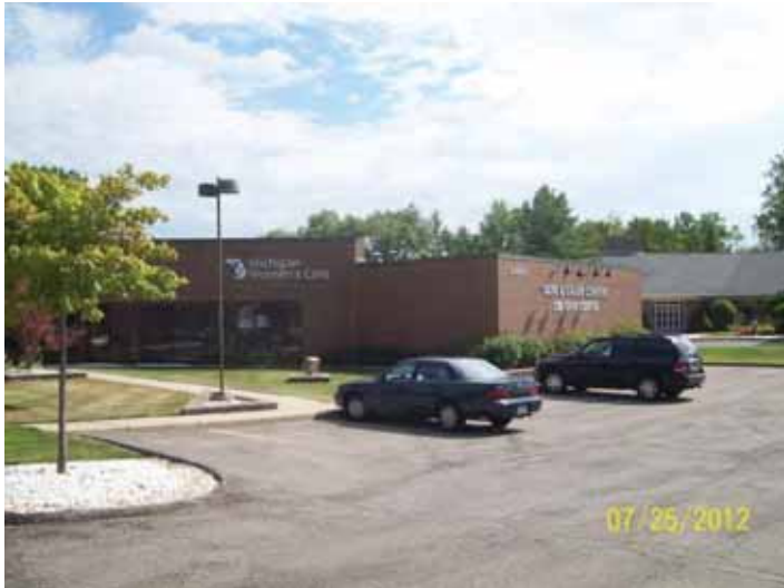
Commercial Office Complex: (Michigan Women's Care) - 42680 Ford Road
