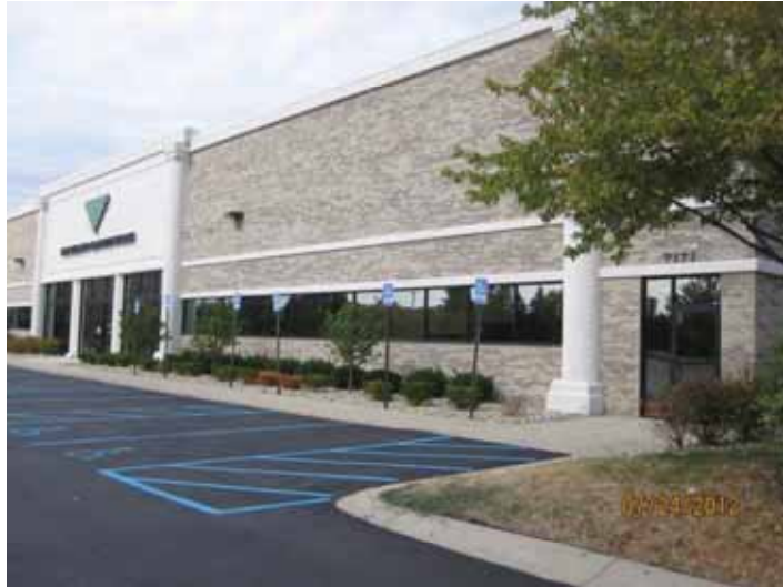
Marble & Granite Work - 7171 N Haggerty Road (west of Haggerty)
