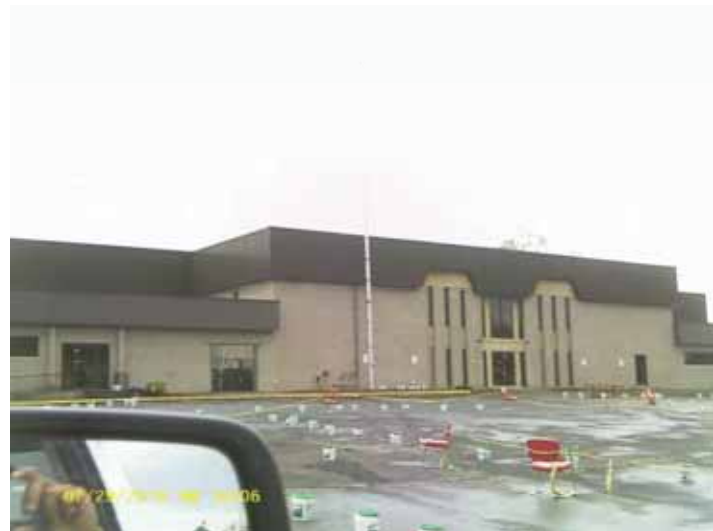
Apparently vacant building: 41677 Ford Road
