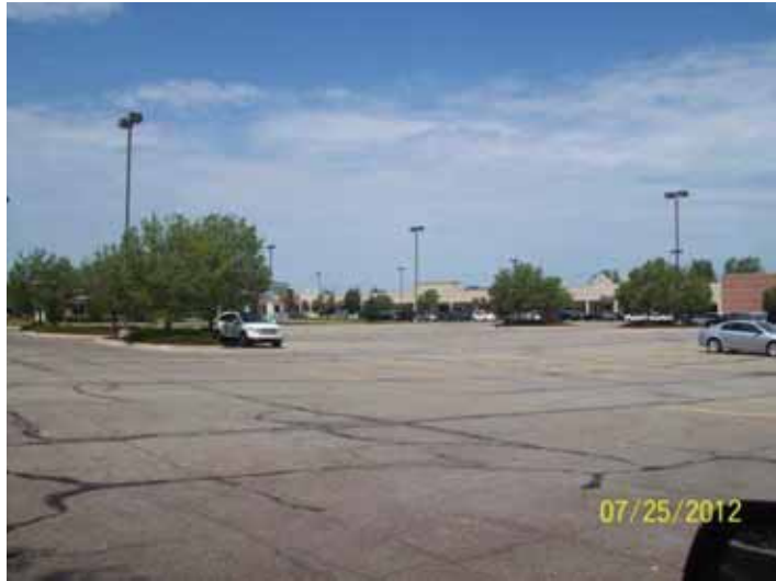
Retail Complex Parking
