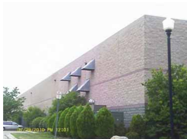
REC # 13: Industrial (MTW) – 7261 Commerce Boulevard
