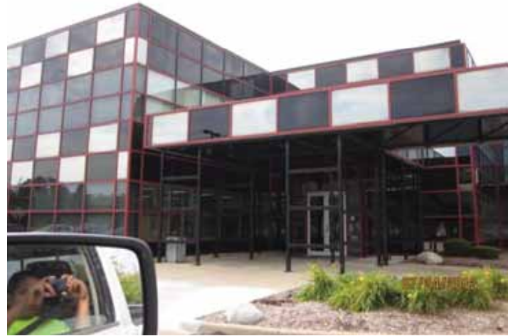
Yzaki North America Tooling Center – 6700 N Haggerty Road
