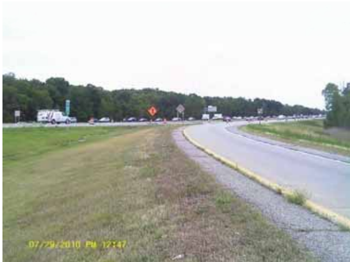
Street View: Entrance to I-275 SB looking south
