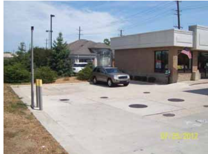
REC # 11: BP Gas Station - 44404 Ford Road (USTs & Vents)
