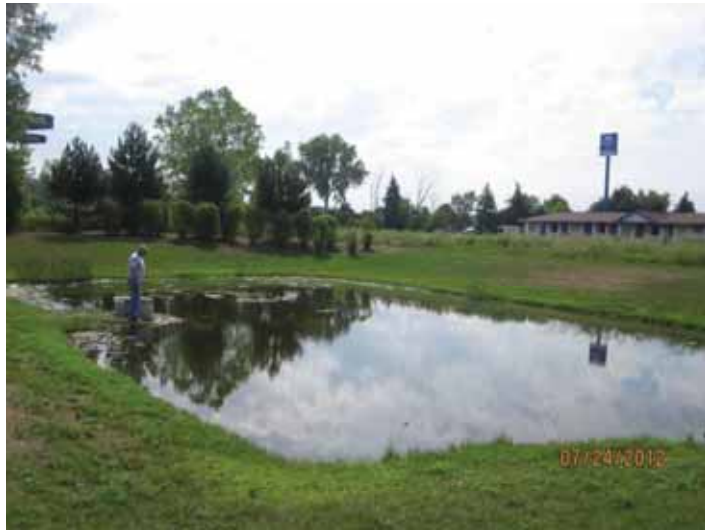
IKEA overflow parking area and constructed retention pond
