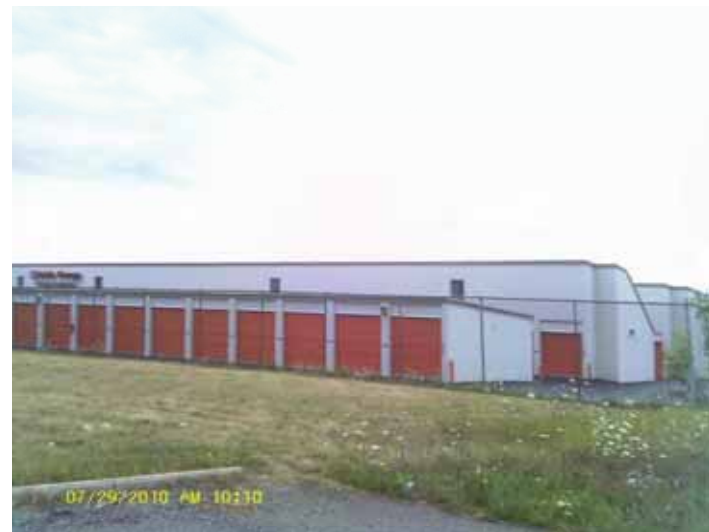
Public Storage - 2101 North Haggerty Road
