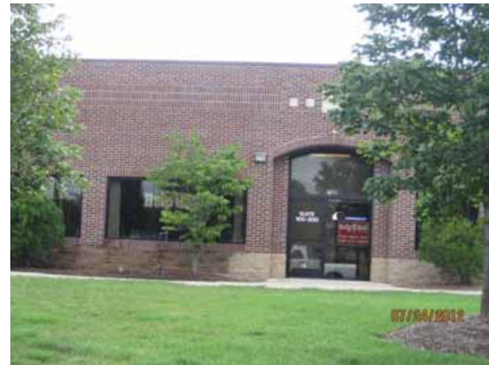
Tandy Engineering & Associate - 7120 N Haggerty Road
