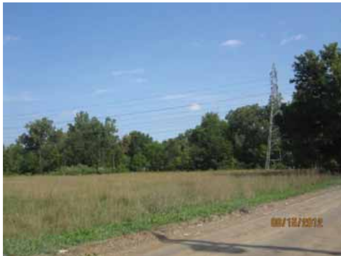
Power transmission line west of Lotz Road
