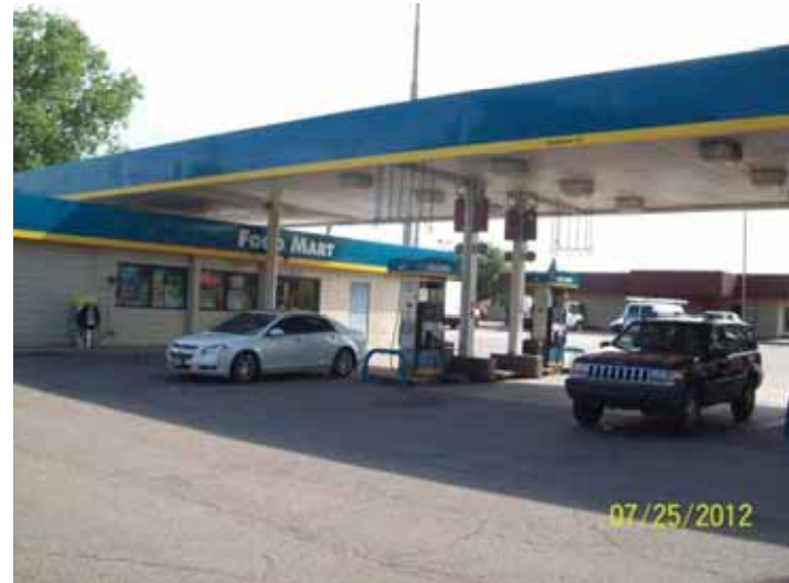
REC # 17: Valero Gas Station (Knight Enterprises) - 41350 Ford Road (Drums & Gas Vents)
