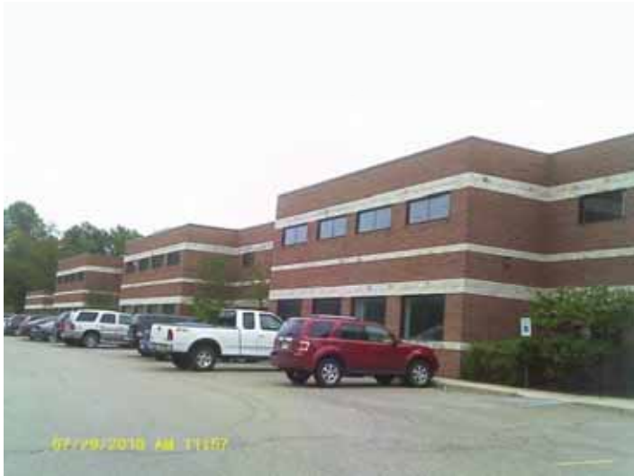
Koppernick Testing Center: 40433 to 40665 Koppernick Road
