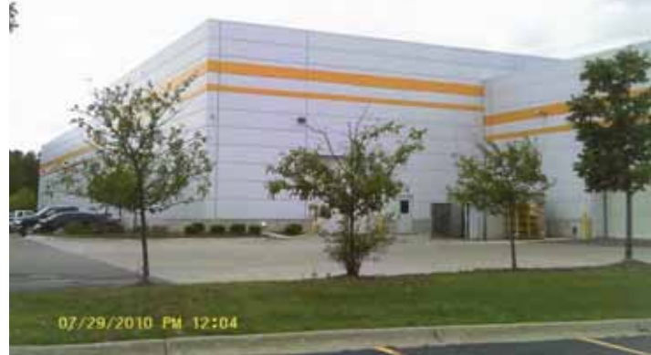
Industrial: G-TAC – 7075 Commerce Boulevard
