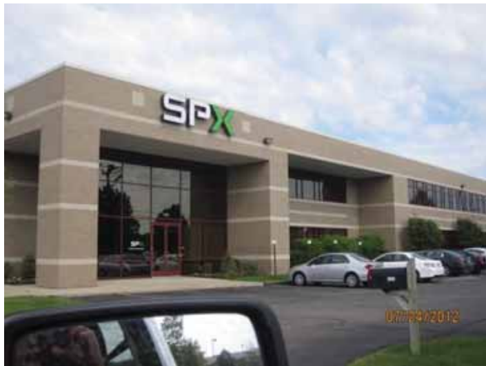
SPX Service Solutions - 7121 N Haggerty Road
