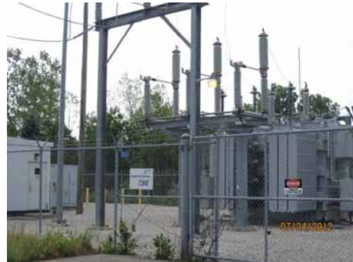
REC#43: Kopperrick Substation - 7101 Kopperrick Road (west of Haggerty Road)
