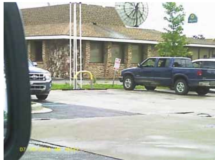
REC#2: BP Gas Station - 41345 Ford Road (USTs and vents)
