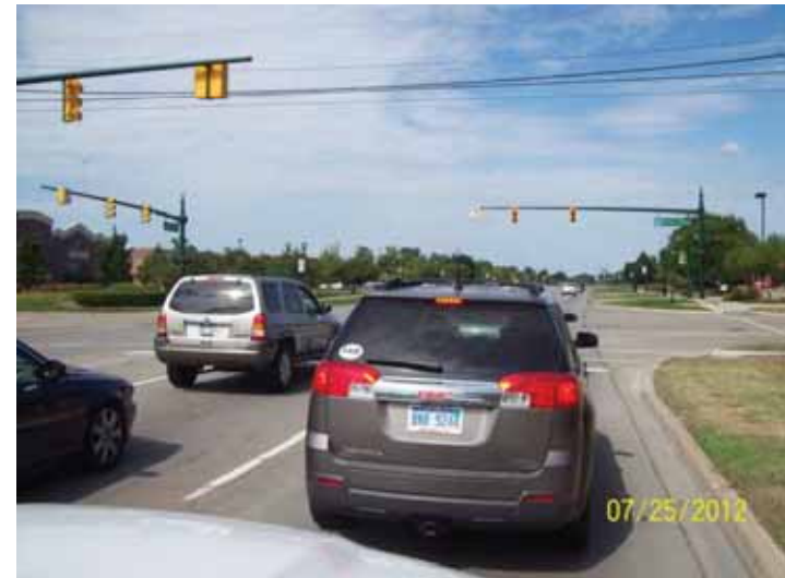
Morton Taylor Road/Ford Road Intersection (looking west)
