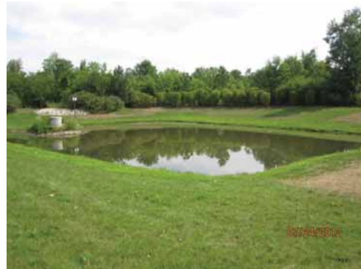
IKEA overflow parking area constructed retention pond
