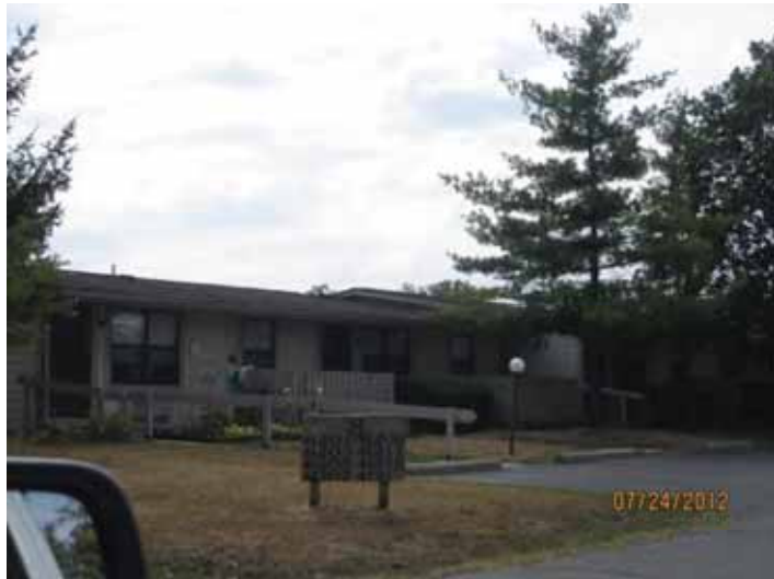
Heatmor Apartments – 41289 to 41301 Southwind Drive (typical)
