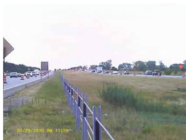
Street View: I-275 south bound (SB)
