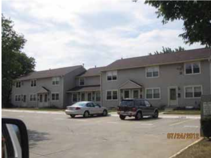
Canterbury Mews Apartment – 784 Canterbury Circle (typical)
