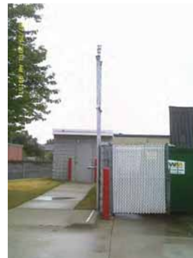
REC # 29: Speedway Gas Station - 5596 Lilley Road (tank vent)
