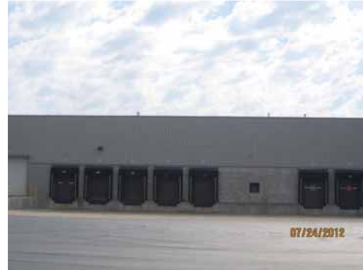
Marble & Granite Work (Loading area) - 7171 N Haggerty Road (west of Haggerty)
