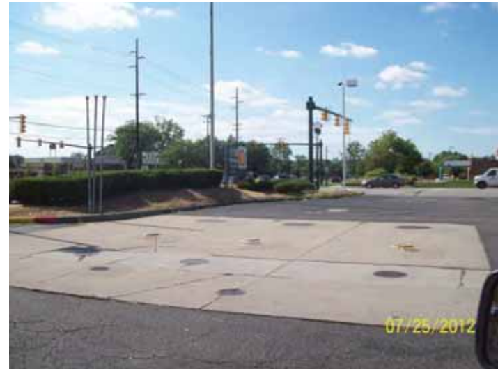
REC # 27: Shell Gas Station - 5640 Haggerty Road (USTs & vents)
