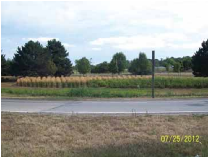
NW Quadrant of I-275/M-153 Interchange
