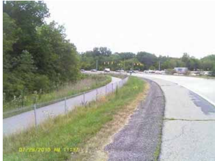
Street View: I-275 North Ramp looking backward (NE quadrant of interchange)
