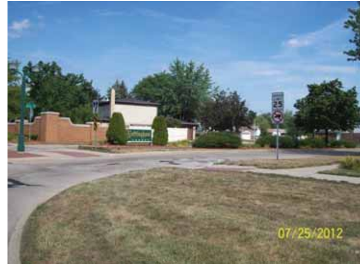
Nottingham Forest Housing Development: (Ford Road Entrance)
