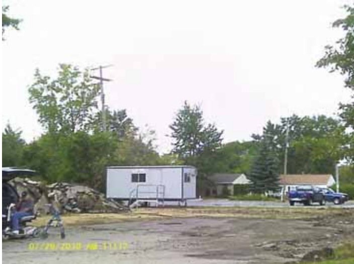
Backside of the Apparently Abandoned Building
