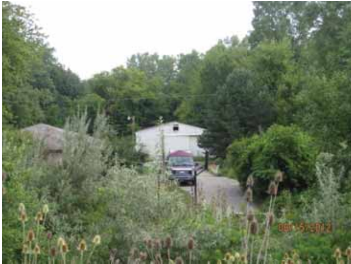
Residential house on Cherry Hill Road (east of I-275)
