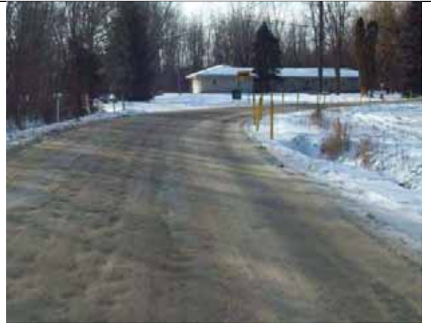
Exhibit 3: Lotz Rd Horizontal Curve (250' Radius – facing south)
