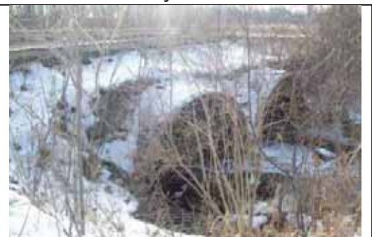
Exhibit 2: Existing 96" Cross Culverts Conveying Willow Creek
