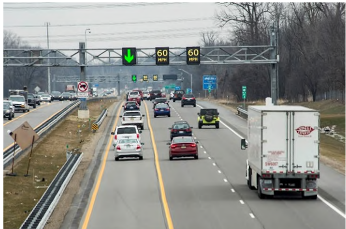
Figure 2. Configuration of US-23 Flex Lane
