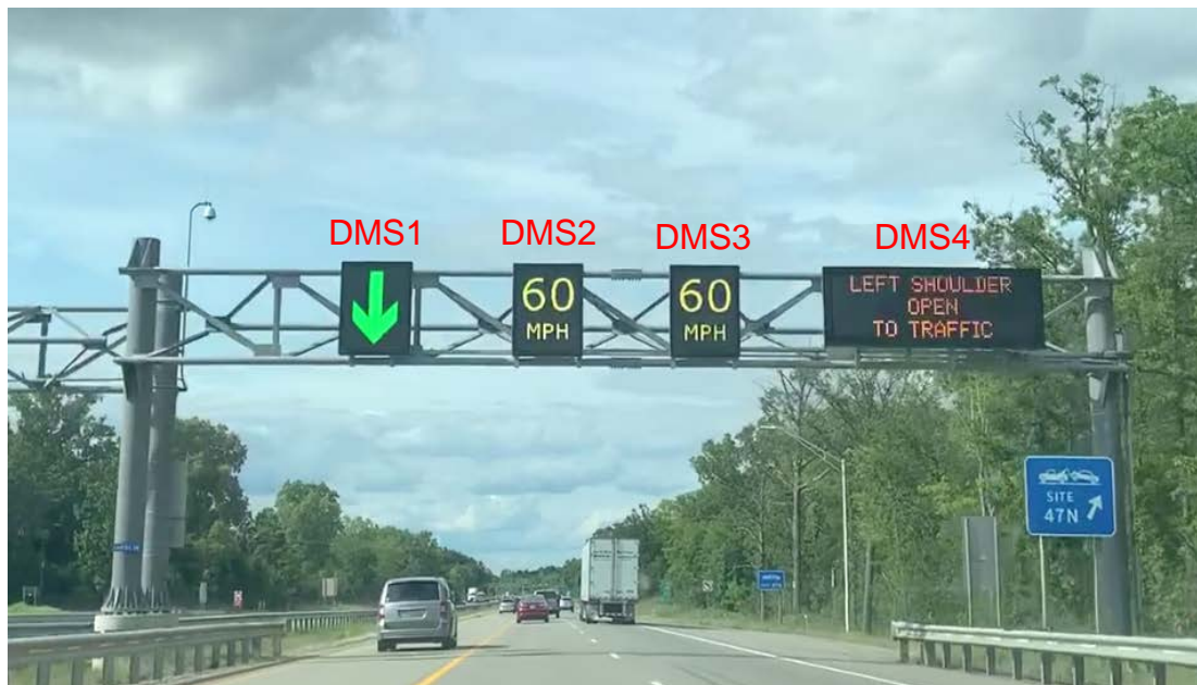
Figure 3-7 An example of gantry messages on the US-23 Flex route (NB MM46.8)
