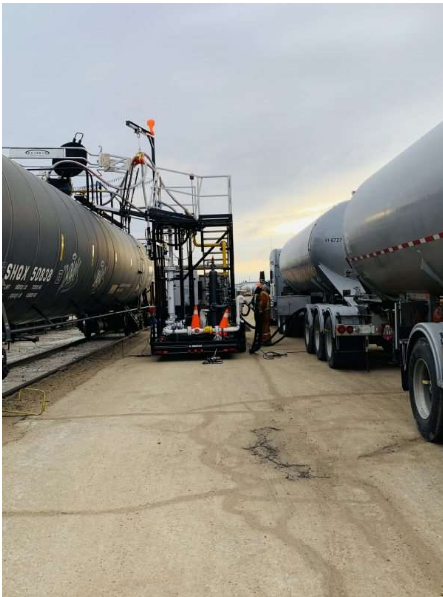
Figure 13. Example of Mobile Propane Transload Equipment
