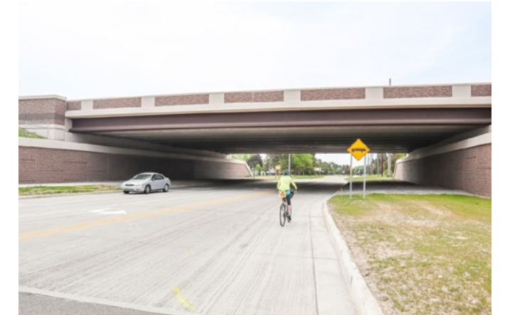
Coolidge Highway overpass lengthened to accommodate future mobility in the city of Troy.
