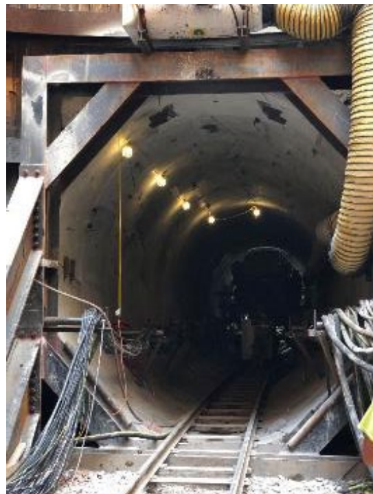
I-75 storage and drainage tunnel being built at the I-696 shaft portal
