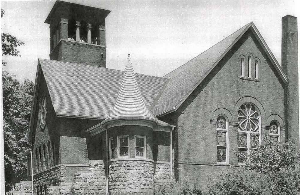
Southwest corner of the original building where the 1960s additions stand.
