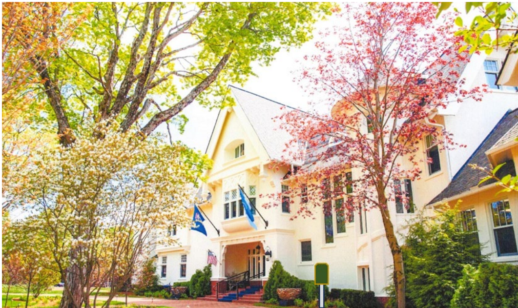
Figure 6. Photograph of the north elevation with proposed marker location.
