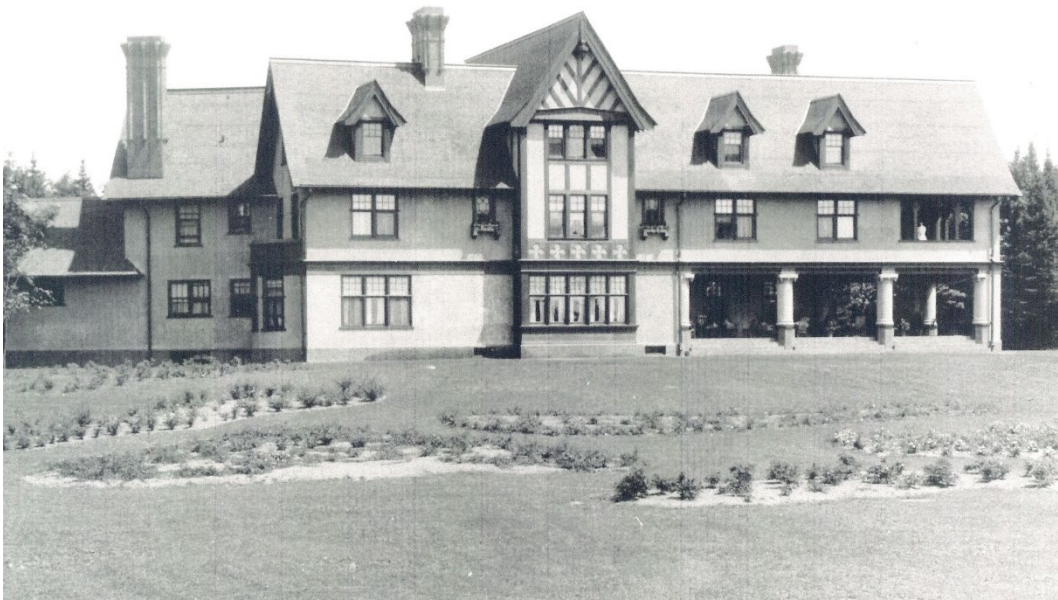
Figure 1. Photograph of the south elevation, 1910.
