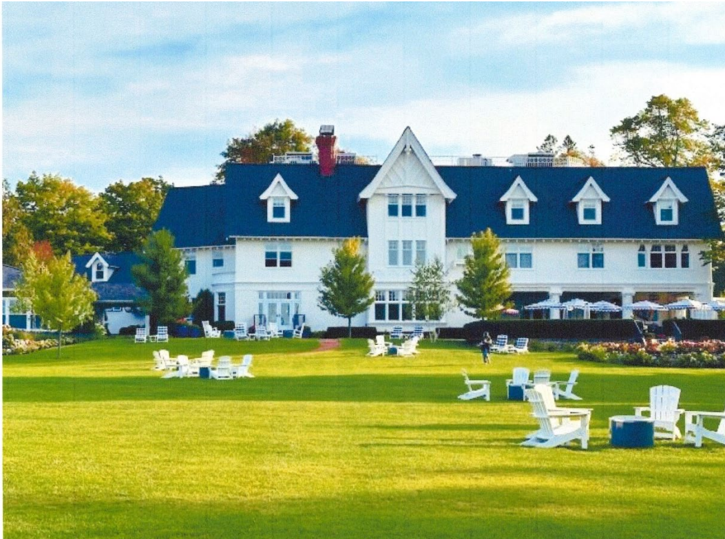
Figure 5. Photograph of the south elevation, 2025.
