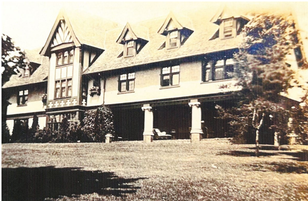
Figure 2. Photograph of the south elevation, 1927.
