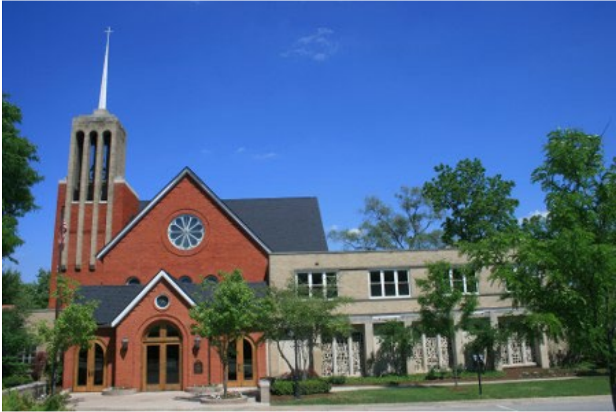
Current exterior of the church, including the original sanctuary (brick facade, left) with the 1962 and 1965 addition visible on the right.
