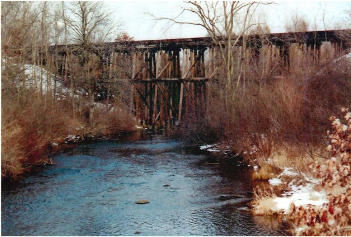
Figure 5. Photograph of the wooden trestle from the access trail, 1999.
