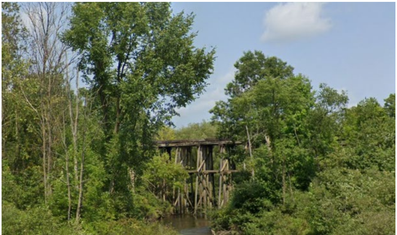
Figure 6. View of the wooden trestle from South Evergreen Drive, July 2024.
