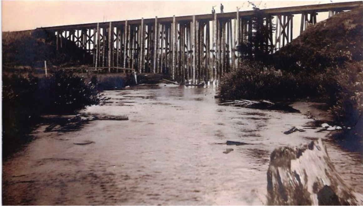
Figure 3. Postcard with the first photograph of the wooden trestle, 1902.
