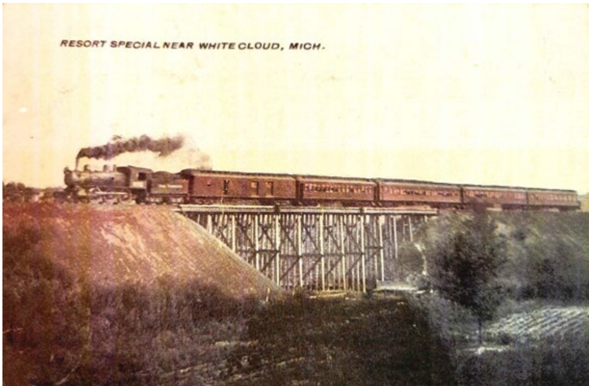
Figure 4. Postcard of passenger train crossing the wooden trestle, n.d. We believe that this image should be included on the marker.
