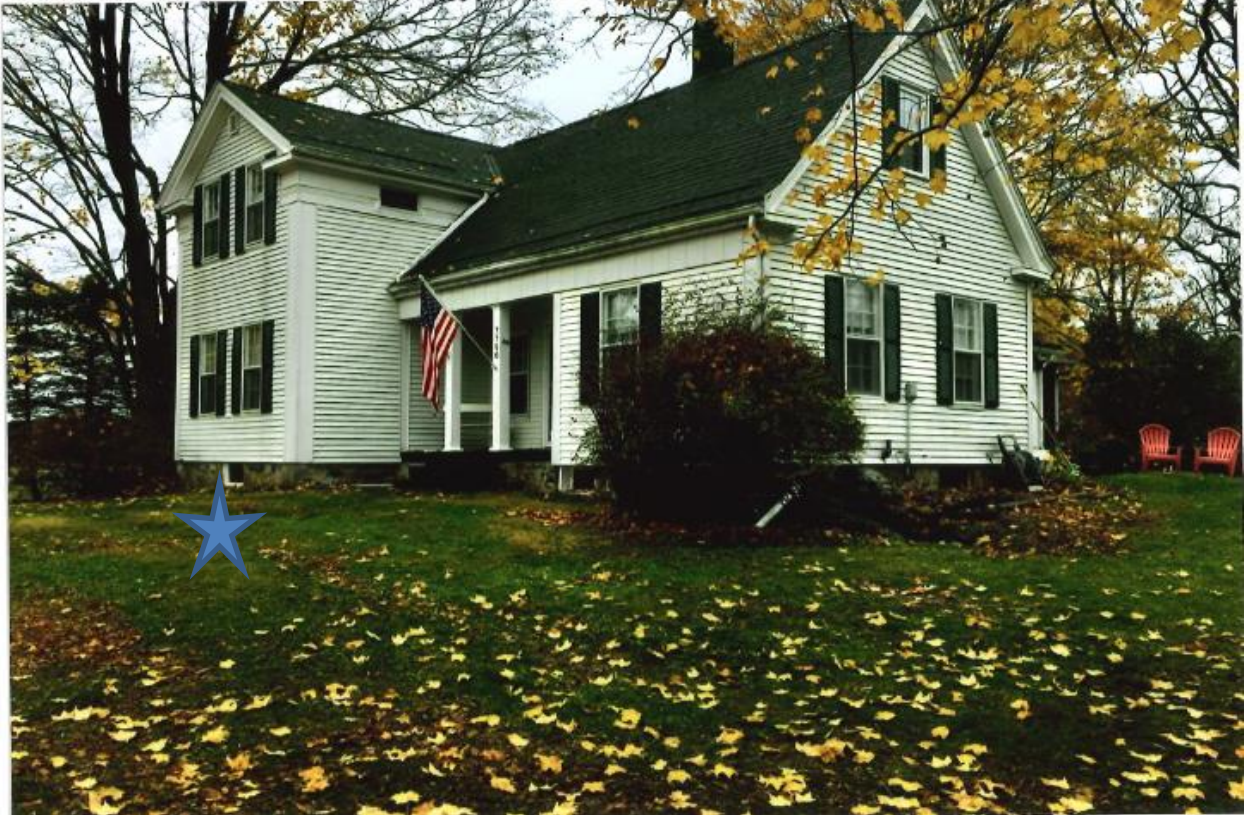
Figure 11. Oblique view of the south and east elevations
