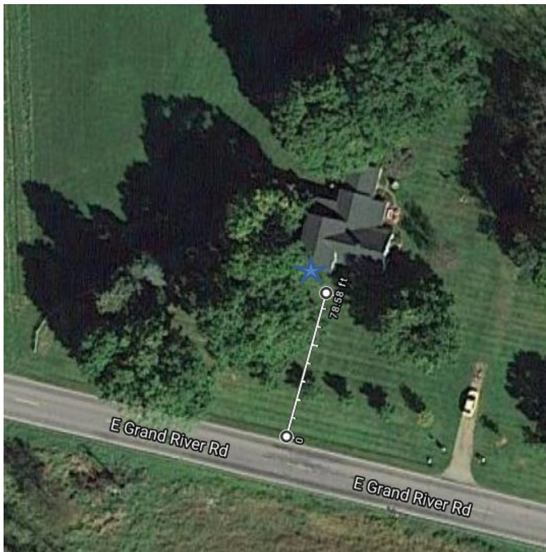
Figure 10. Aerial view of the property
