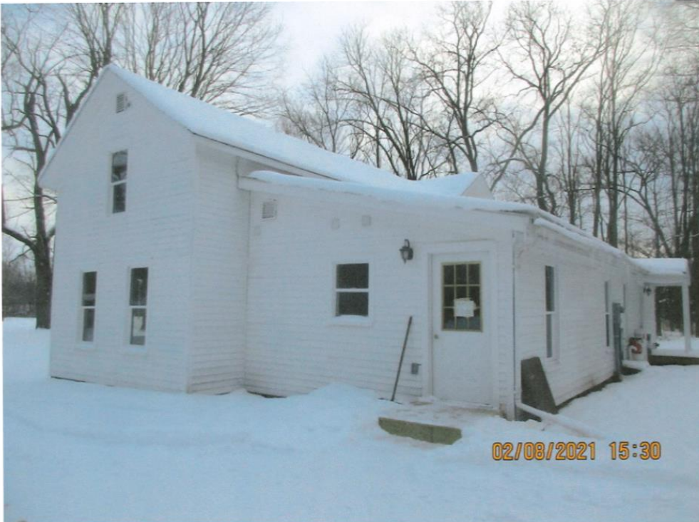
Figure 4. Oblique view-east and north elevations
