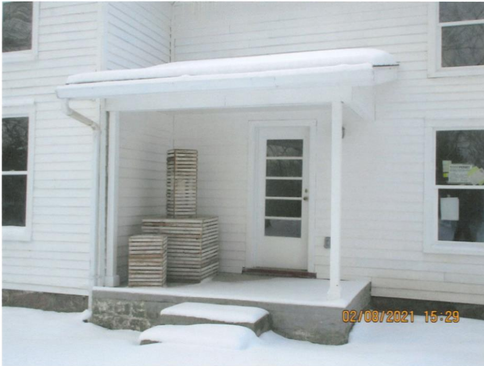
Figure 2. Porch Constructed in 2020
