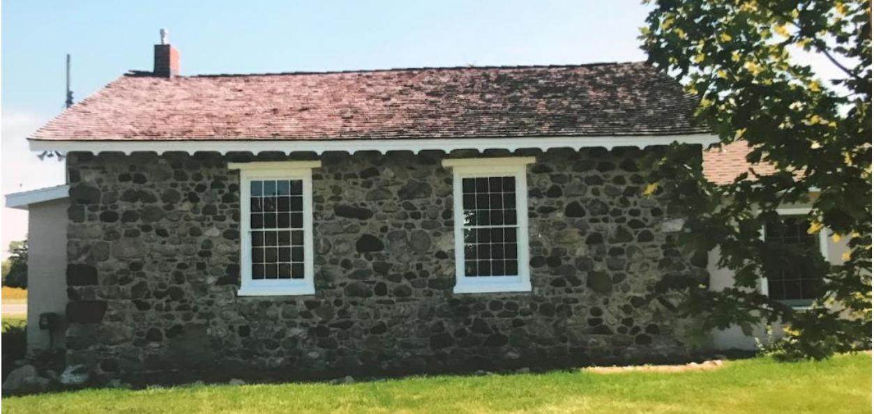
Figure 14. Stone School-west elevation
