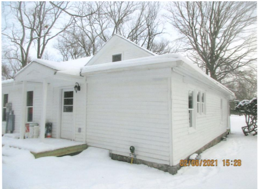
Figure 6. Oblique view- north and west elevations
