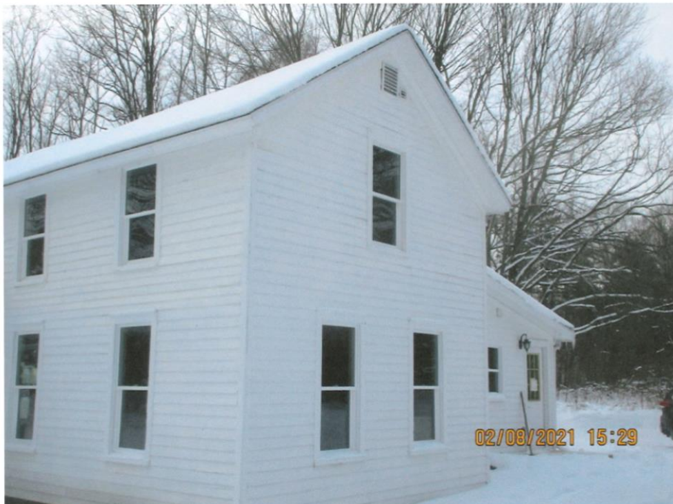
Figure 5. Oblique view-south and east elevations
