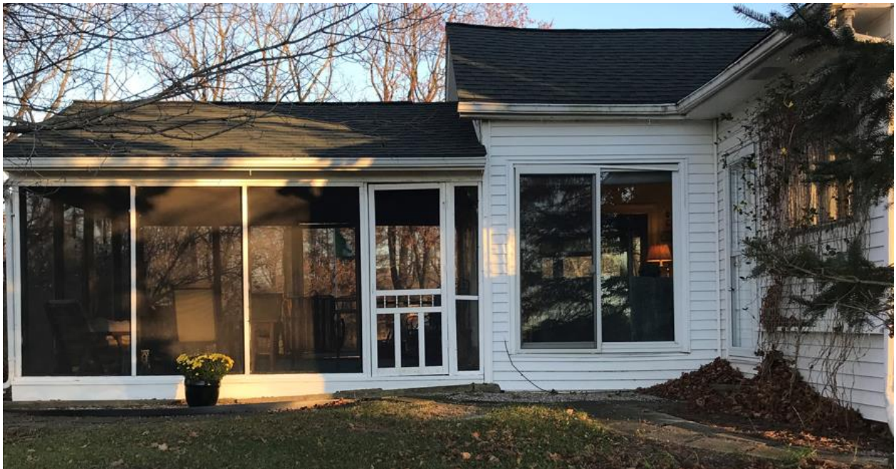
Figure 5. West elevation of the rear additions
