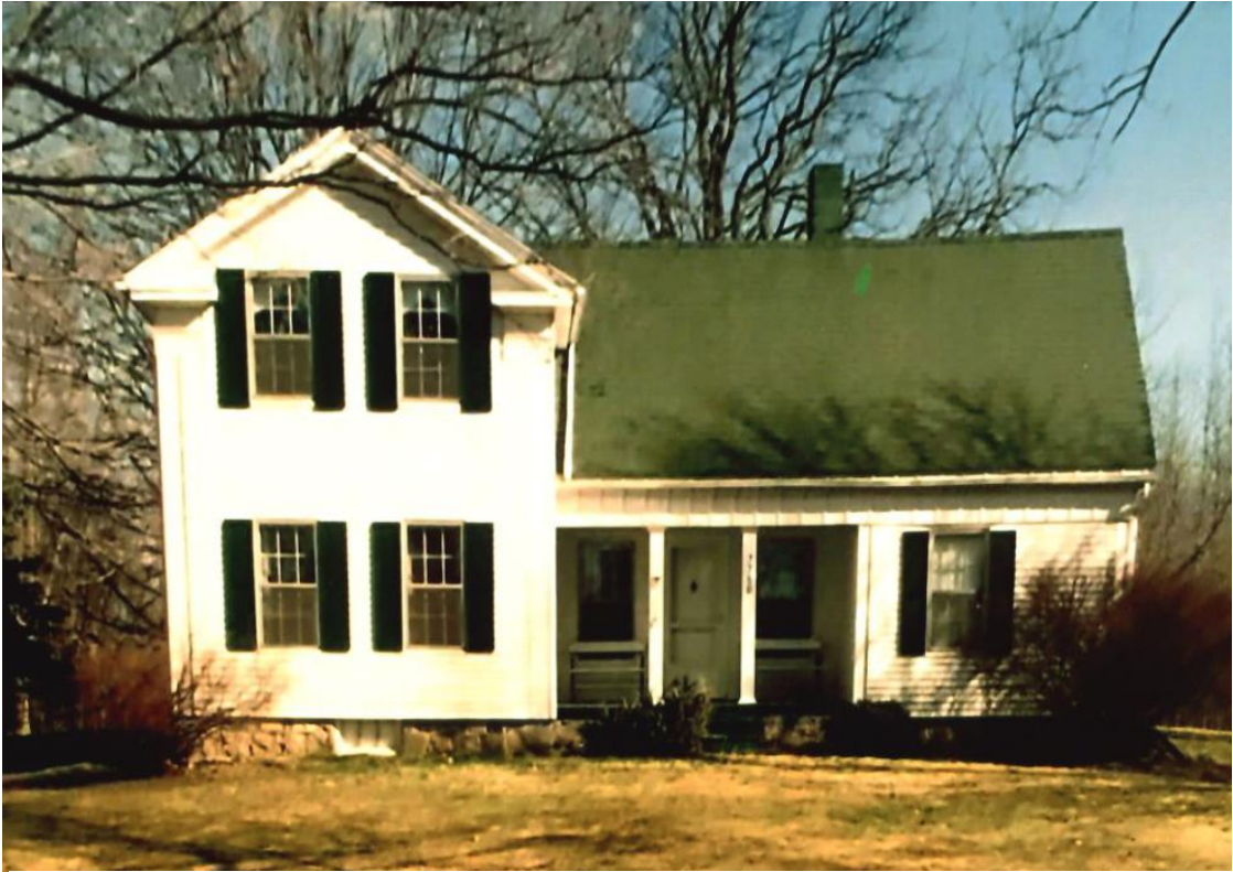
Figure 3. South elevation viewed from the road
