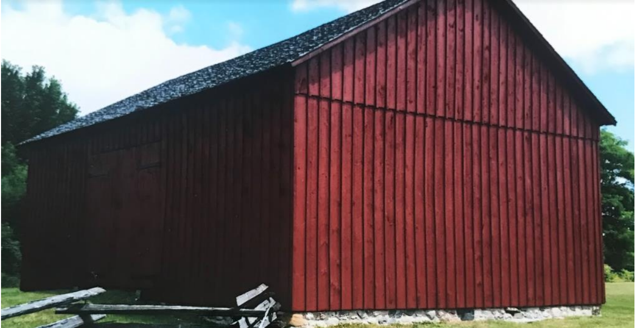
Figure 18. Dickerson Barn-oblique view-southwest
