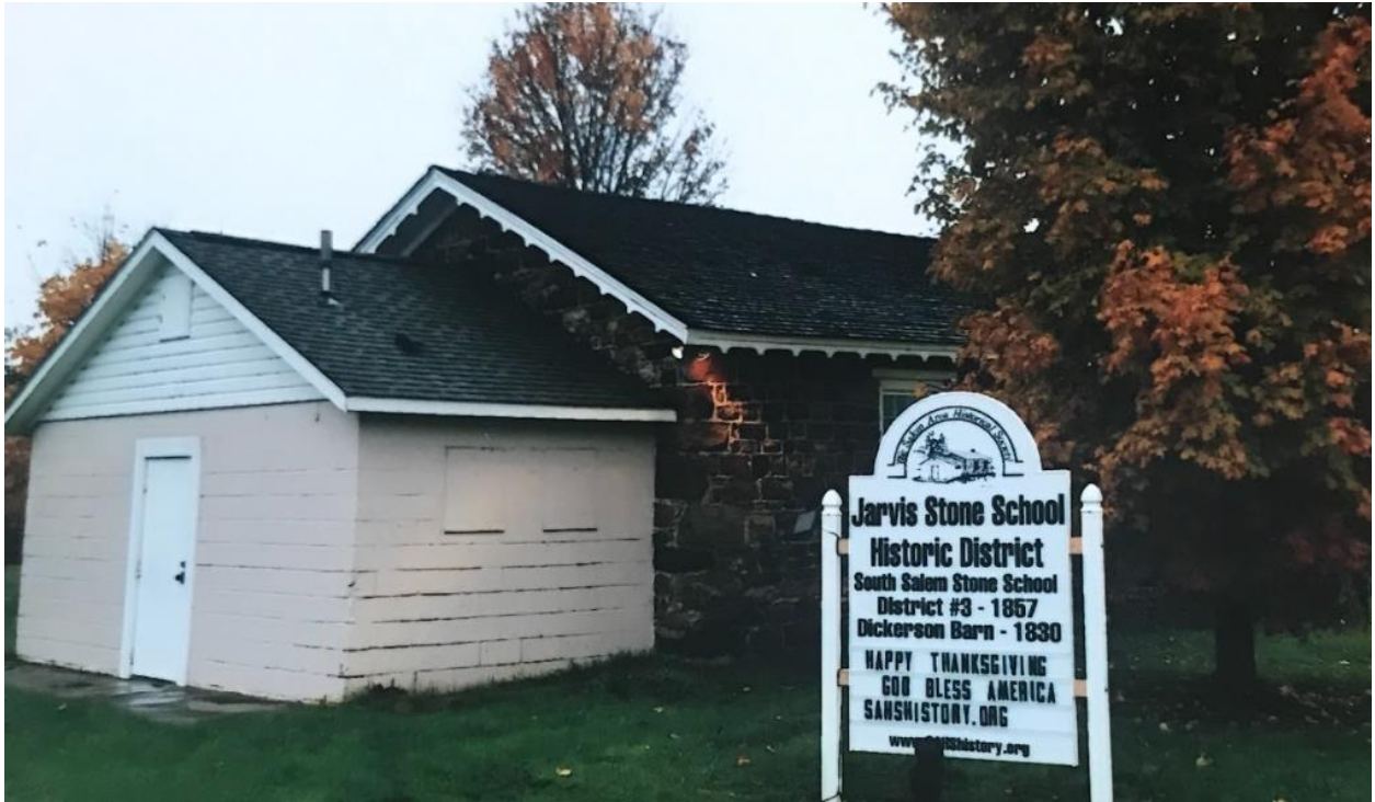
Figure 12. Stone School-oblique view-southeast
