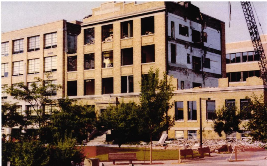
Figure 3. Demolition of the St. Joseph Seminary Building in 1983.
