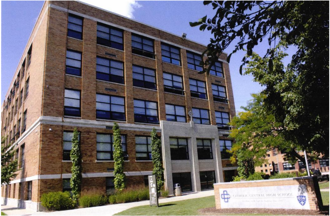
Figure 8. 1952 Catholic Central Highschool building, 2021.
