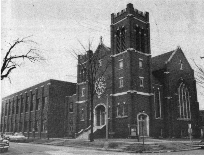
The 1918 church, demolished after the completion of the 1973 structure.
