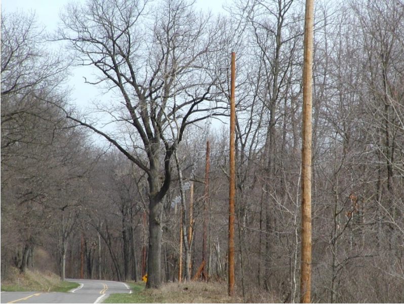
FIGURE 44 – ASC CONSTRUCTION BY A ROADSIDE
