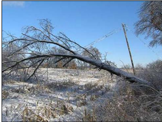
FIGURE 46 – ASC SUPPORTING A FALLEN TREE
