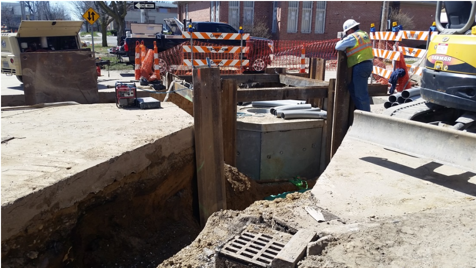
FIGURE 70 – INSTALLATION OF NEW MANHOLES OR VAULTS
