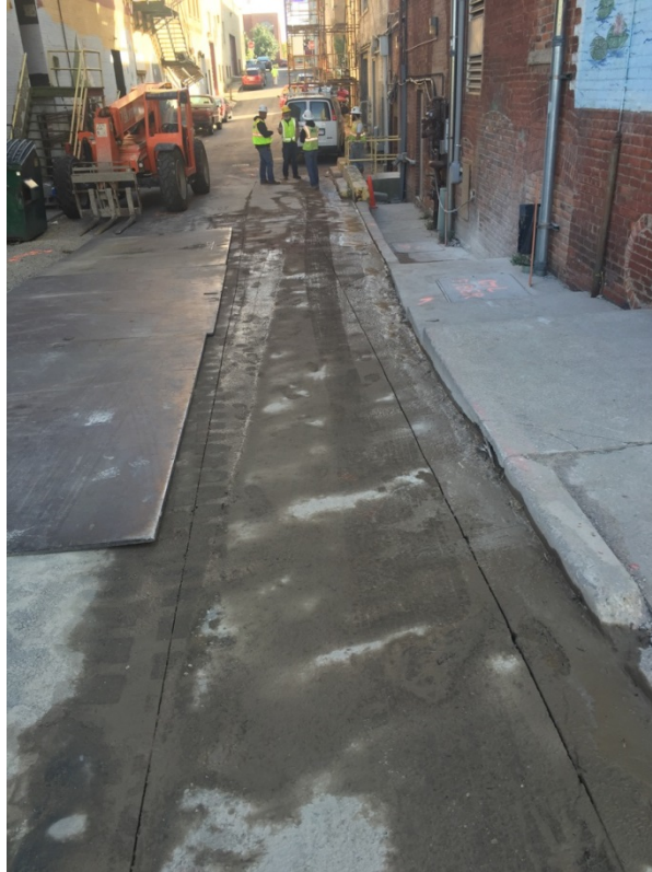
FIGURE 55 – REPLACEMENT OF THE DUCT BANK IN ALLEY FOR THE NEW SERVICE
