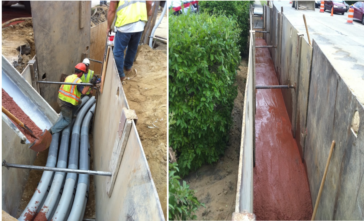
FIGURE 71 – INSTALLING NEW CONCRETE ENCASED DUCT BANK
