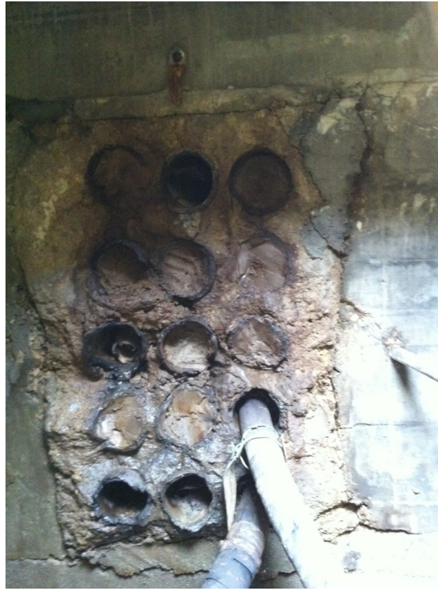
FIGURE 65 – DAMAGED / CRUSHED DUCT BANKS
