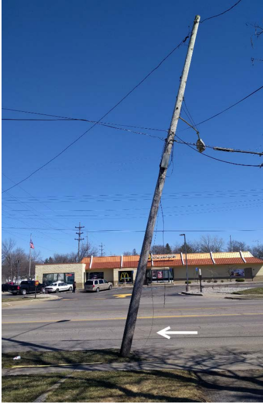
FIGURE 102 – SECONDARY POLE WITH BROKEN GUY
