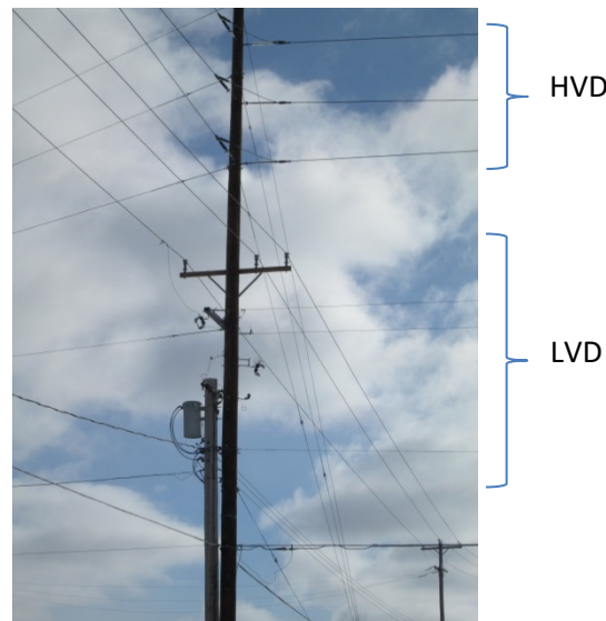
FIGURE 75 – UNDERBUILT LVD ON HVD SYSTEM AWAITING TRANSFER TO NEW POLE
