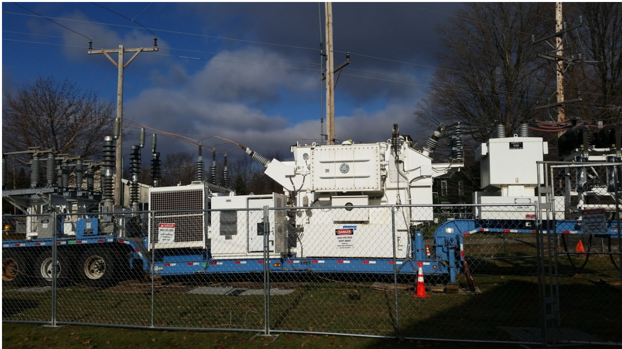
FIGURE 86 – MOBILE SUBSTATION
