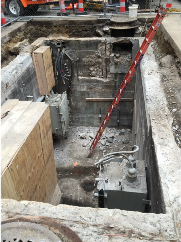
FIGURE 69 – VAULT OR MANHOLE ROOF REPLACEMENT
