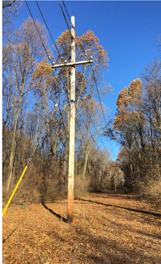
FIGURE 43 – SHIELDED LVD TREE WIRE CONSTRUCTION
