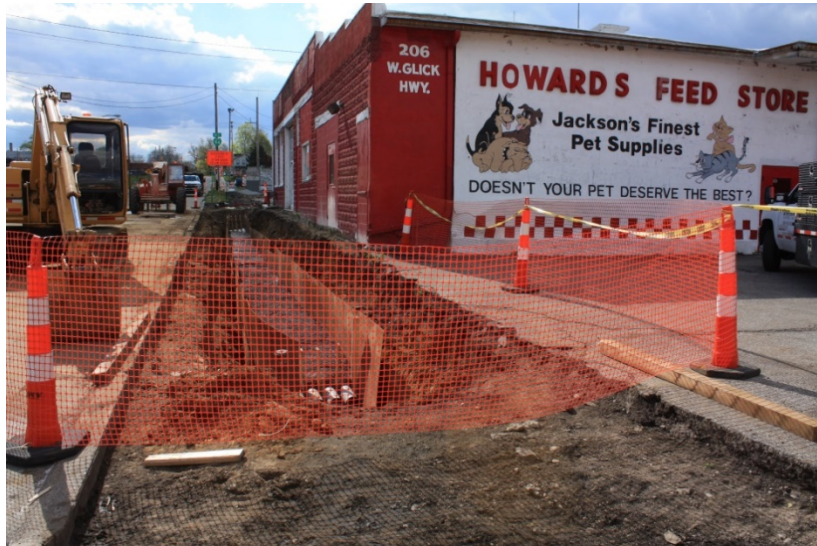
FIGURE 77 – NEW DUCT BANK BUILT IN SIDEWALK AREA
