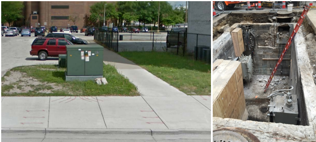
FIGURE 76 – DIRECT BURY SYSTEM (LEFT), VAULT WITH STRUCTURAL DAMAGE (RIGHT)
