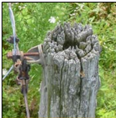
FIGURE 84 – DETERIORATION OF HVD POLE TOP FROM HELICOPTER INSPECTION
