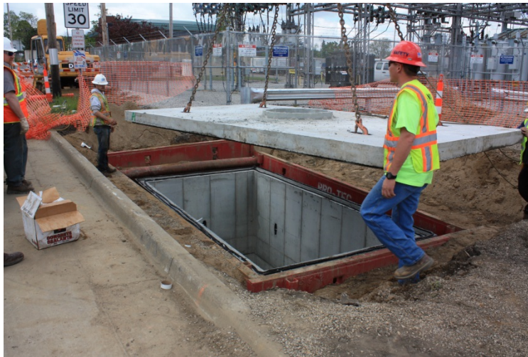
FIGURE 79 – INSTALLATION OF MANHOLE ROOF
