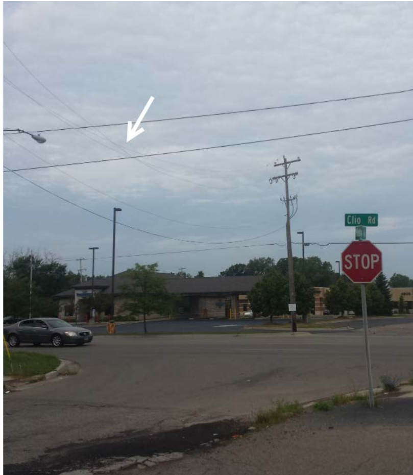
FIGURE 98 – SAGGED WIRES ON PIERSON FEEDER
