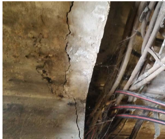
FIGURE 66 – DETERIORATED MANHOLE/VULT ROOFS
