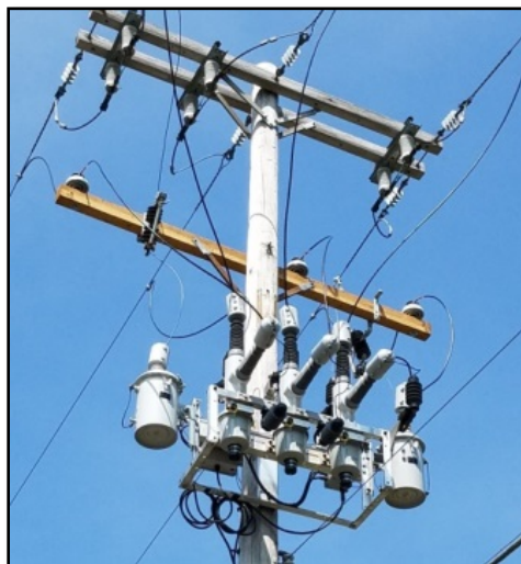
FIGURE 32 – INSTALLED AUTOMATIC TRANSFER RECLOSER
