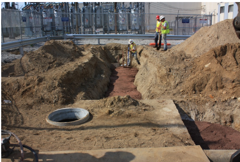
FIGURE 78 – INSTALLATION OF NEW DUCT BANK AND MANHOLE
