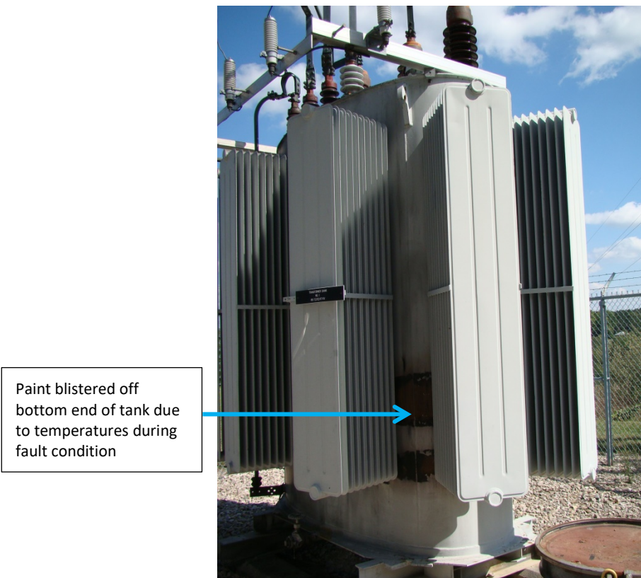
FIGURE 61 – FAILED TRANSFORMER AT SHANTY CREEK SUBSTATION
