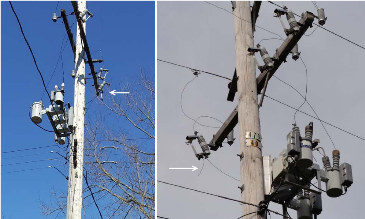
FIGURE 97 – BLOWN CAPACITOR FUSES
