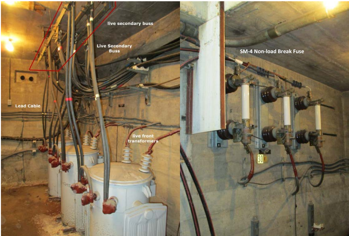
FIGURE 89 – OLD ROBINSON VAULT EQUIPMENT BEFORE RELIABILITY PROJECT
