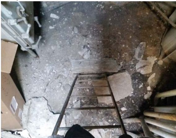
FIGURE 66 – DETERIORATED MANHOLE/VULT ROOFS
