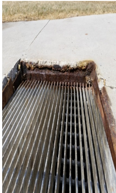
FIGURE 68 – RUSTED/DETERIORATED VAULT HATCHES AND VENTS
