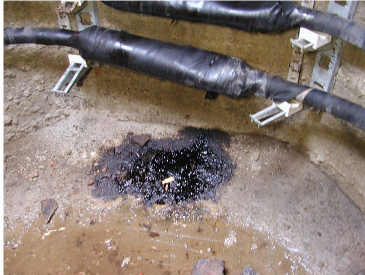
FIGURE 64 – DAMAGED CABLE
