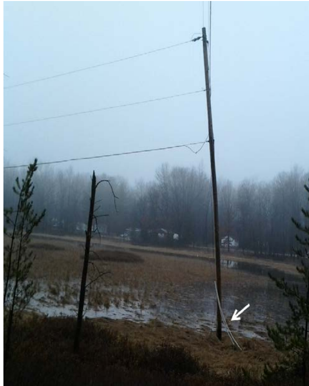
FIGURE 103 – PRIMARY POLE WITH BROKEN GUY
