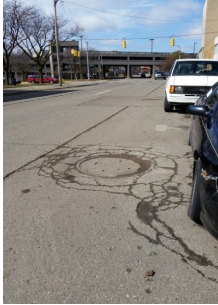
FIGURE 67 – SUNKEN/DETERIORATED MANHOLE ACCESS
