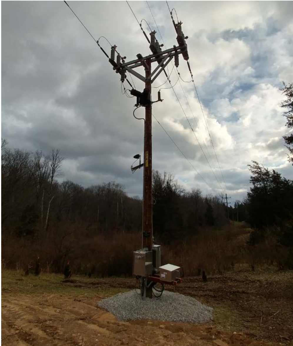
FIGURE 63 – TYPICAL 46 kV MOAB SWITCH
