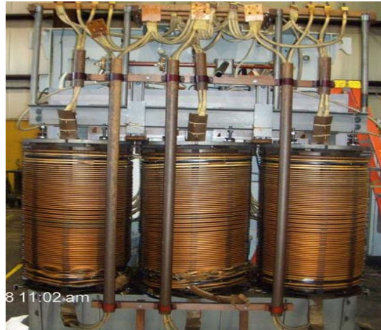
FIGURE 59 – AC TRANSFORMER FAILURE AT GLADWIN SUBSTATION
