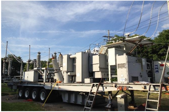
Portable Substation
