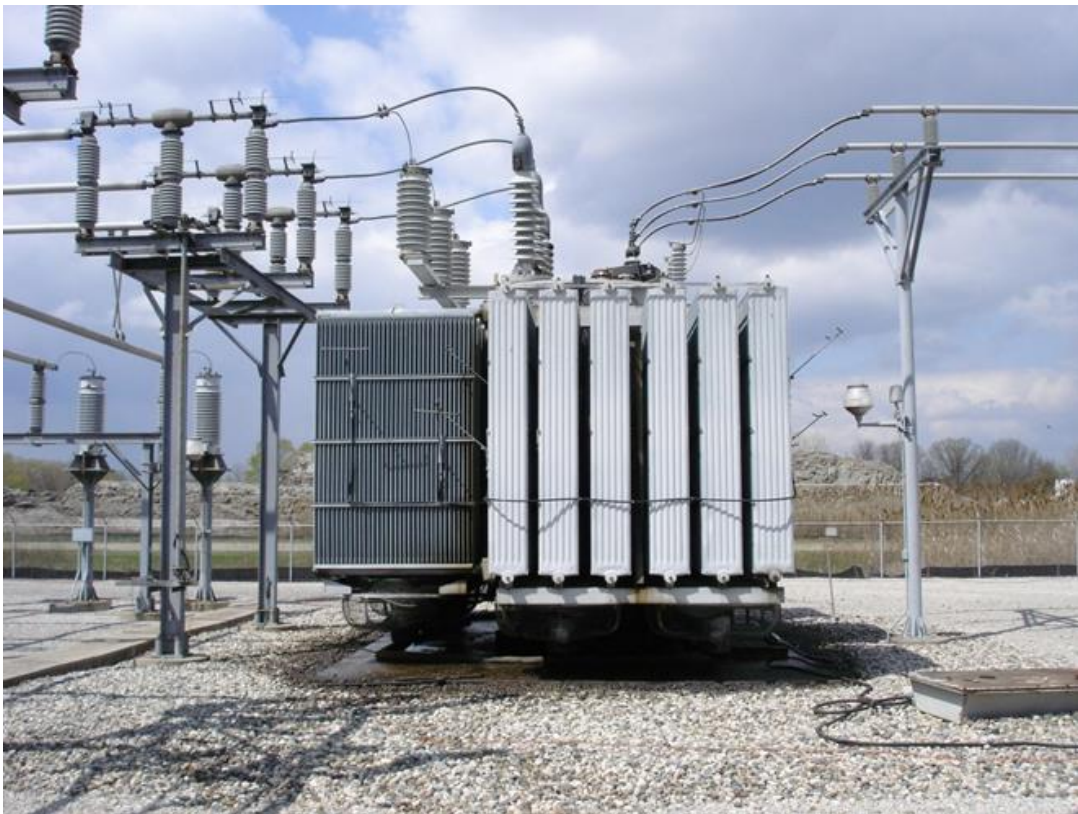
Exhibit 4.1.1 Substation Power Transformer
