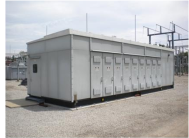
Two-Tier Switchgear
