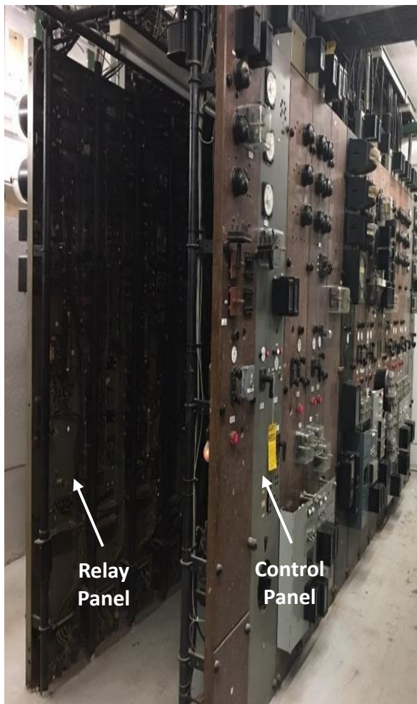
Old Marble Relay Panel (Separate panels for relay and control functions)
