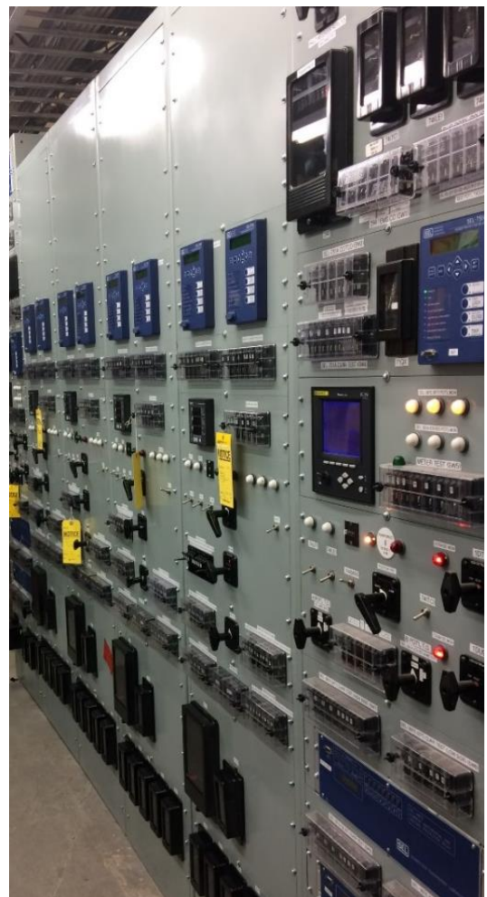
Modern Relay Panel (Single panel for relay and control functions)
