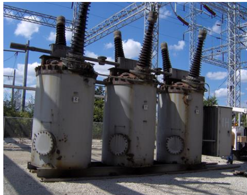
Traditional 120 kV Oil Breakers
