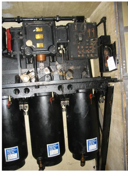
Traditional 4.8 kV Oil Breakers
