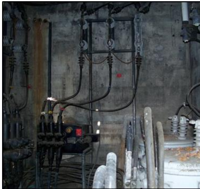
Exhibit 4.18.1 Underground Vault and Equipment
