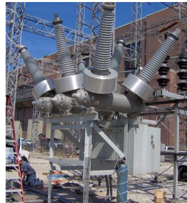
Modern 120 kV Gas Breakers
