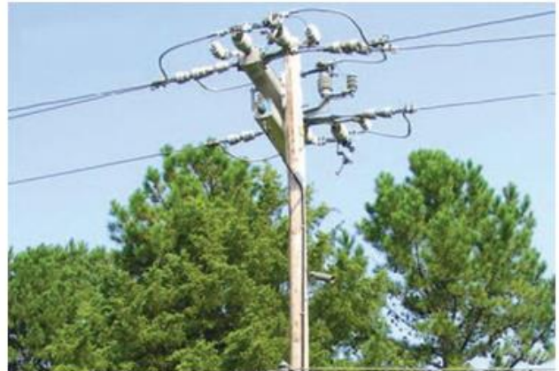
Bridges Auto Topper switches
