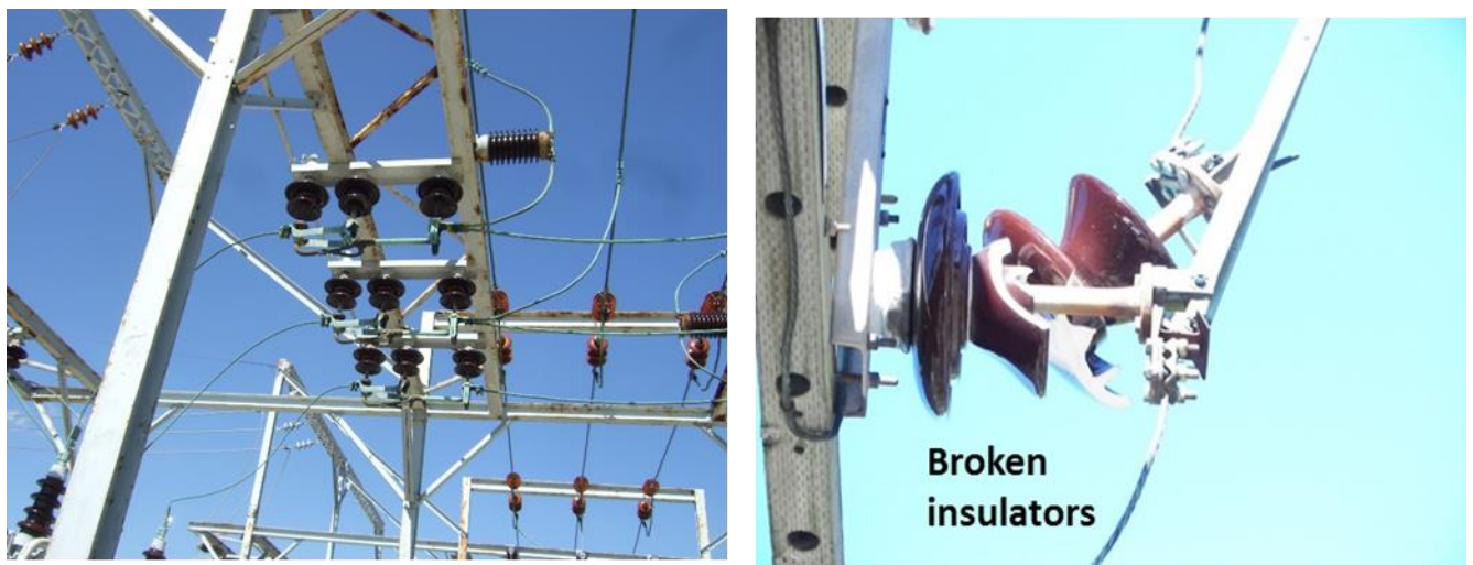
Exhibit 4.4.1 Cap & Pin Disconnect Switch
