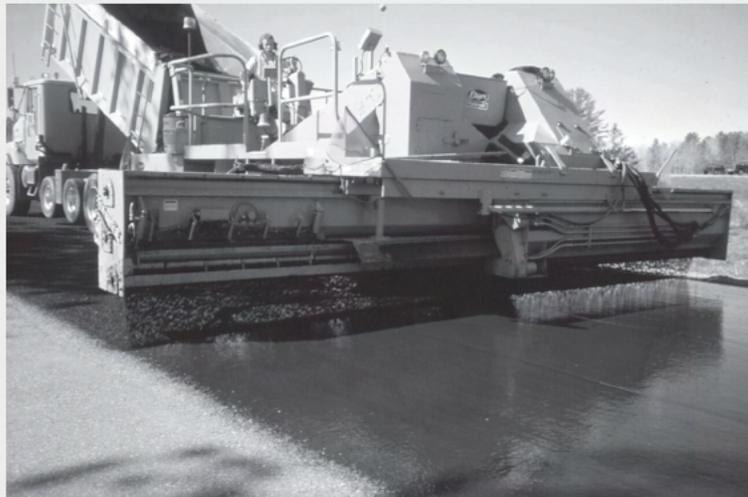
▲ Spreading cover aggregate
