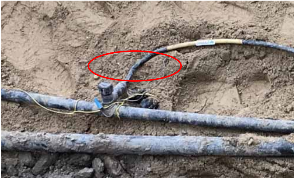
Location of cut by contractor
