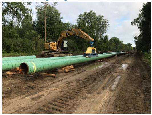
Transporting pipe from yard to site. Laid in a line along the right of way in preparation for bending and welding.
