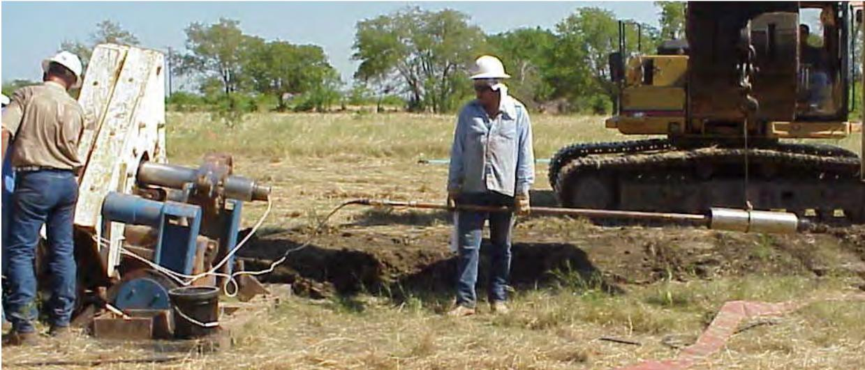
Steering tool being inserted into a non-magnetic collar
