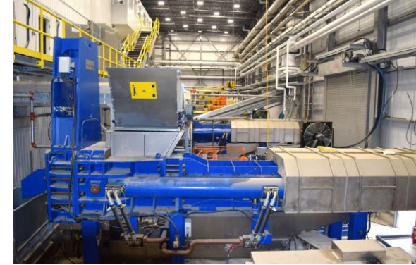
CITY OF TORONTO TORONTO, CANADA PROCESS + SUPPLY + O&M
