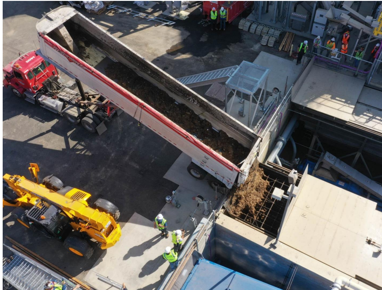
Organic fraction being delivered to Rialto Bioenergy Facility
