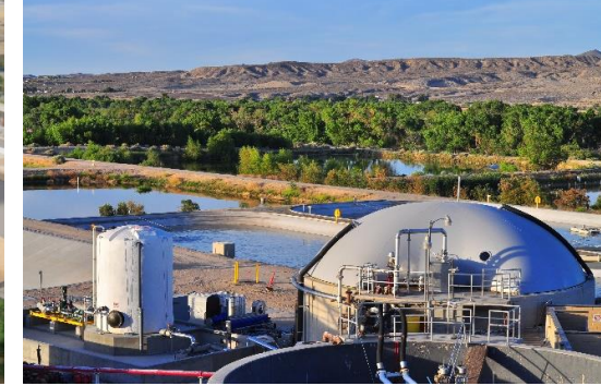
VICTOR VALLEY WATER RECLAMATION AUTHORITY VICTORVILLE, CA DBOOF
