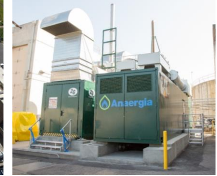
HALE AVENUE RESOURCE RECOVERY FACILITY ESCONDIDO, CA DBOOF
